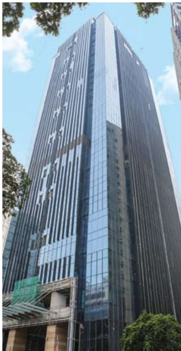
Construction of JKG Tower, Kuala Lumpur
