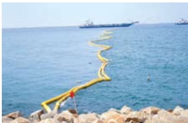
Silt curtain installed during reclamation works to control sedimentation dispersion
