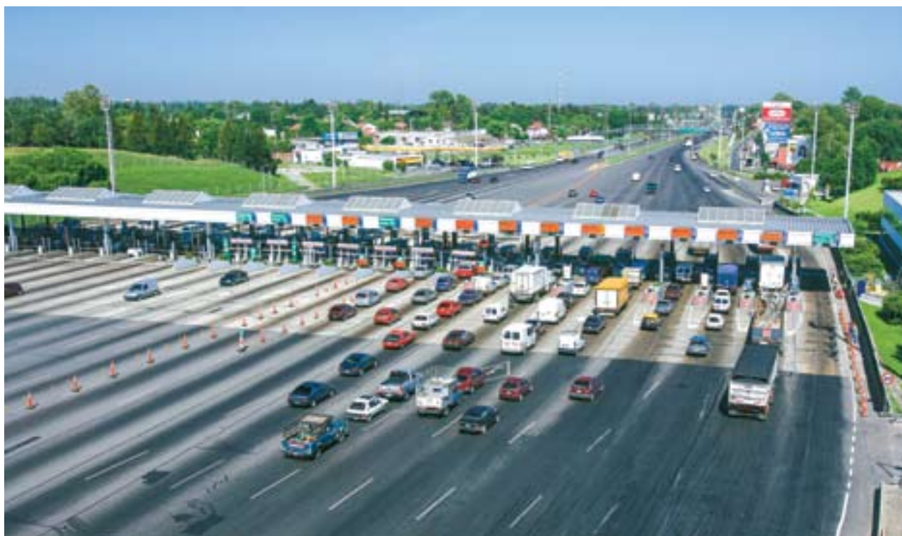
Western Access Tollway, Argentina
