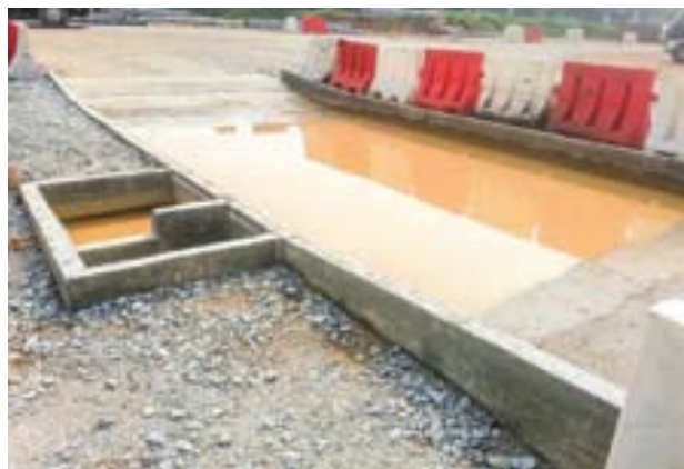
Wheel washing facility provided at site entrance
