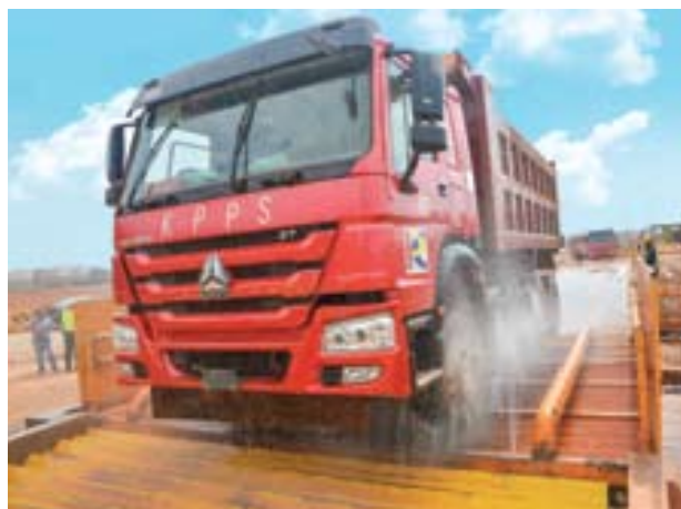
Wheel washing facility to minimise dust pollution
