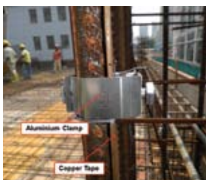
Provision of aluminium clamp for fixing of copper tape for earthing purpose
