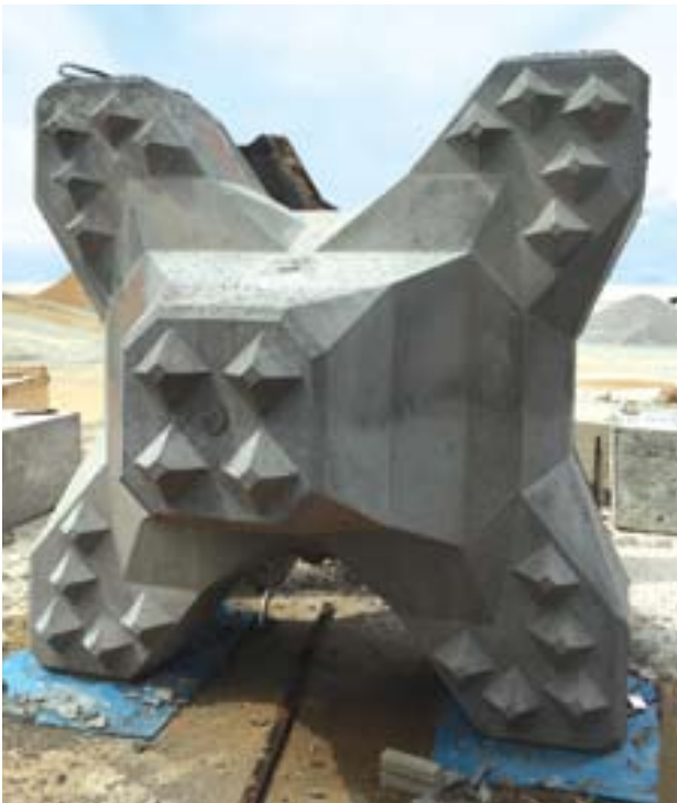
Acropode used for the construction of the breakwater at Kuantan Port
