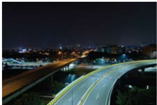
LED streetlights installed on NPE
