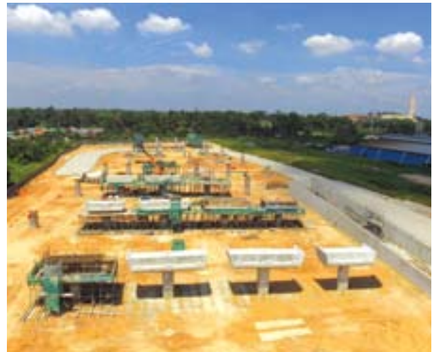
Construction of the WCE
