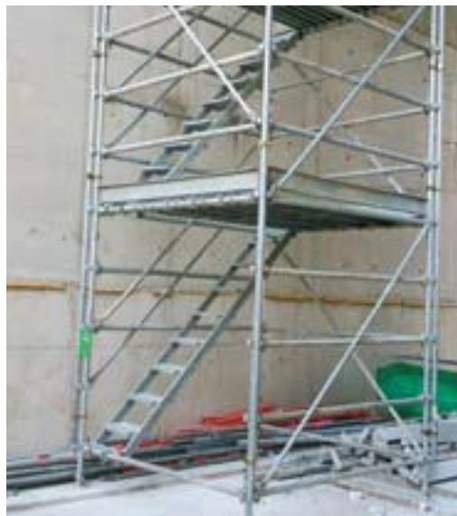
Safe access for workers by using modular scaffold system
