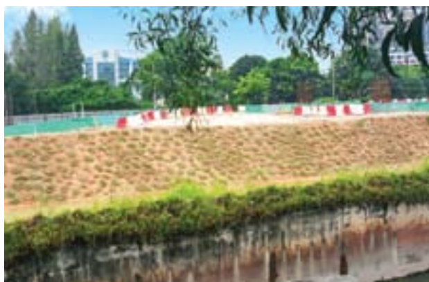
Spot turfing as slope protection
