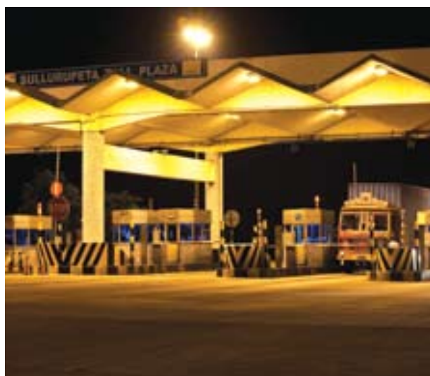
Toll plaza at Swarna Tollway
