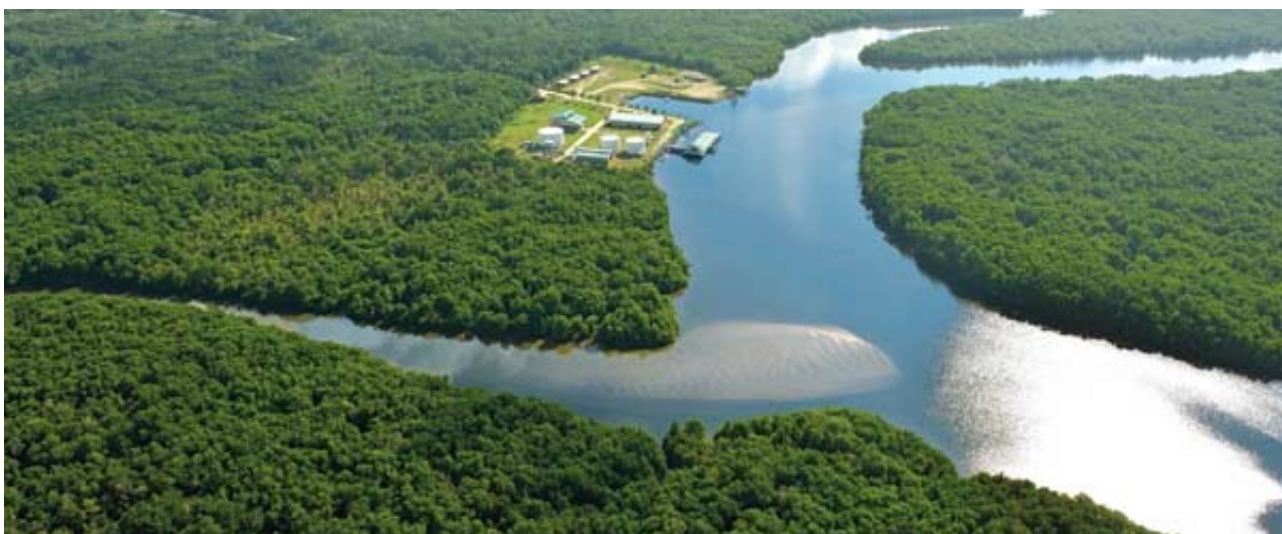
Sg. Sabang Jetty Bulking Facility
