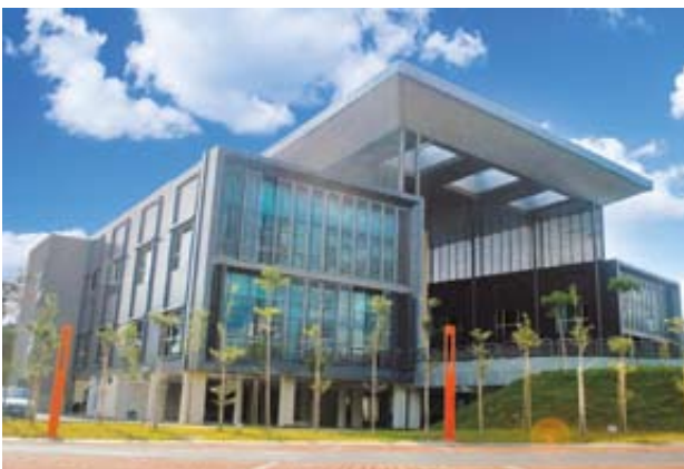
Socso Rehabilitation Centre, Malacca
