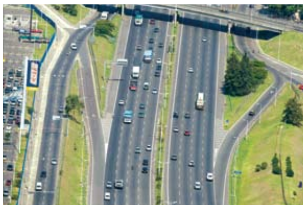
Western Access Tollway, Buenos Aires, Argentina
