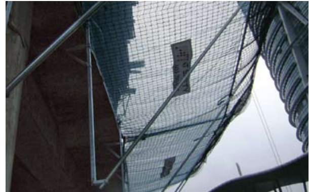
Fall Arrest Safety Nets prevent falling debris from causing injury to people underneath
