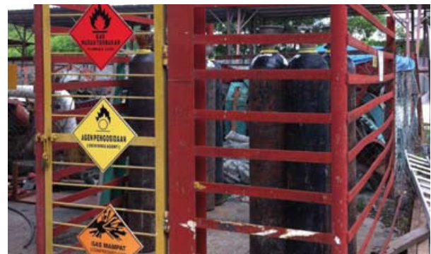
Flammable gas is stored in a safe place to prevent fire hazard
