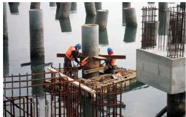
Proper installation of brackets for piles in accordance with quality procedures at our berth expansion project, Kuantan Port
