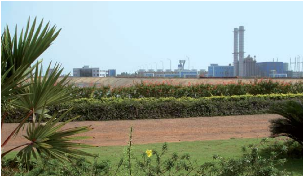
Gautami Power Plant, Andhra Pradesh, India
