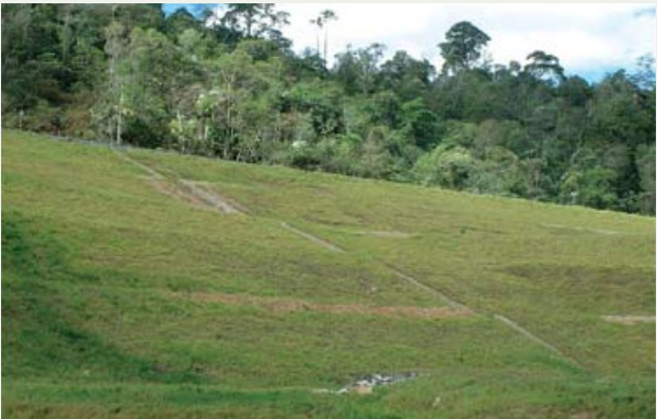
Turfing of slopes to prevent soil erosion
