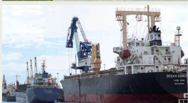
INFRASTRUCTURE Ships at berth, Kuantan Port, Pahang
