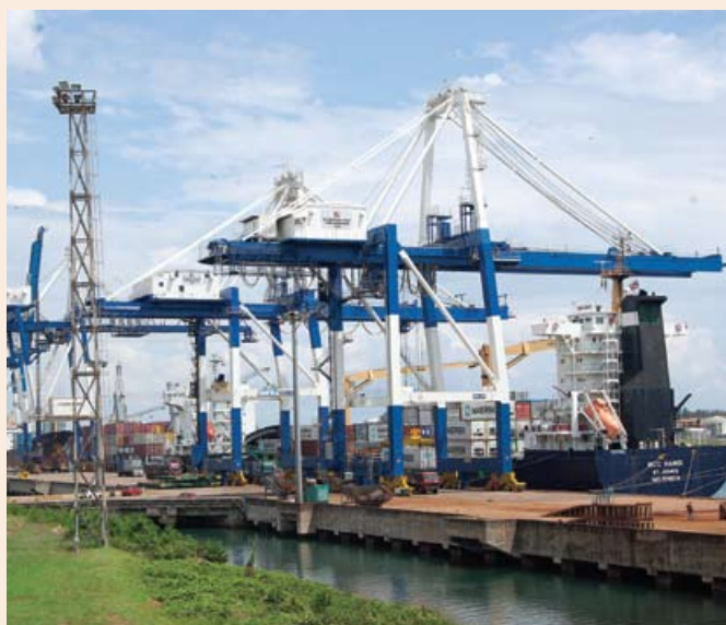
Unloading operations at Kuantan Port, Pahang
