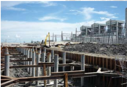
ICP Piles used at Jana Manjung Power Station, Manjung, Perak
