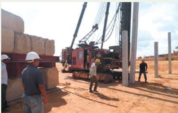
Use of custom made guide to pitch square piles in the correct position at our Perkeso Rehabilitation Centre Project, Malacca
