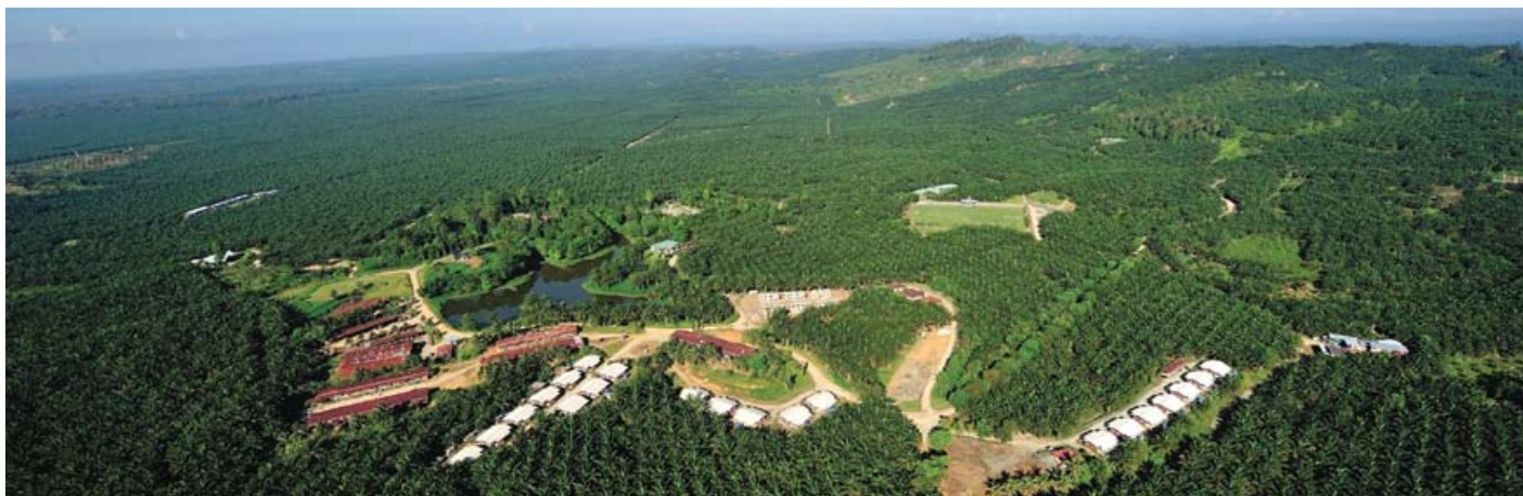
Aerial view of Sungai Sabang Estate
