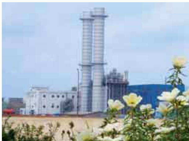
Gautami Power Plant in Andhra Pradesh, India
