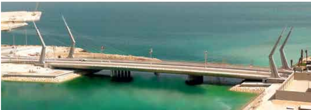
Lulu Reef Access Bridge in Bahrain
