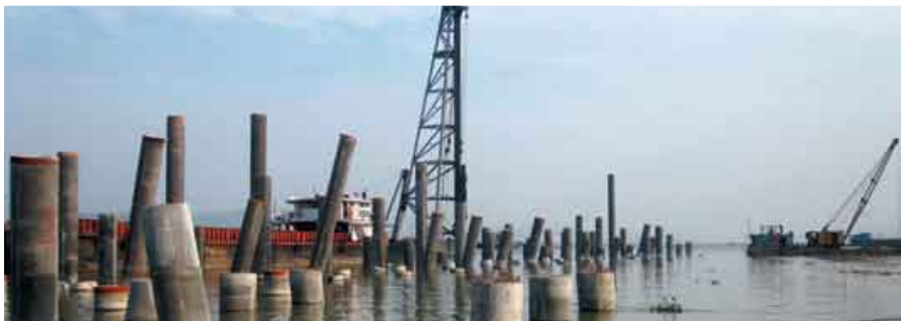
XinHui Paper Mill Jetty, Jiangmen, China
