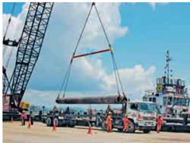
Unloading steel pipes at Kuantan Port
