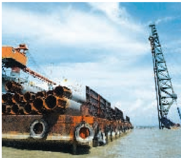
Piles used at the Penang Second Bridge
