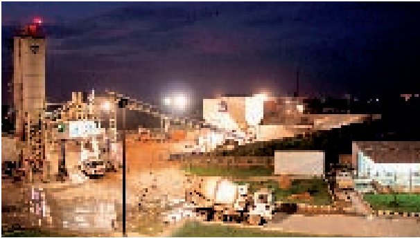
Batching plant in Bachupally, India
