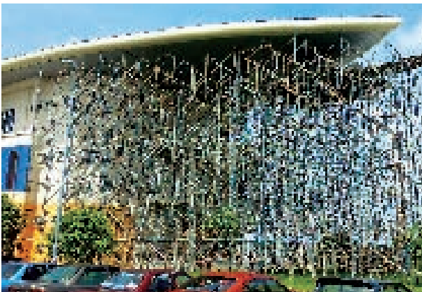
Scaffoldings used at TLDM, West Port
