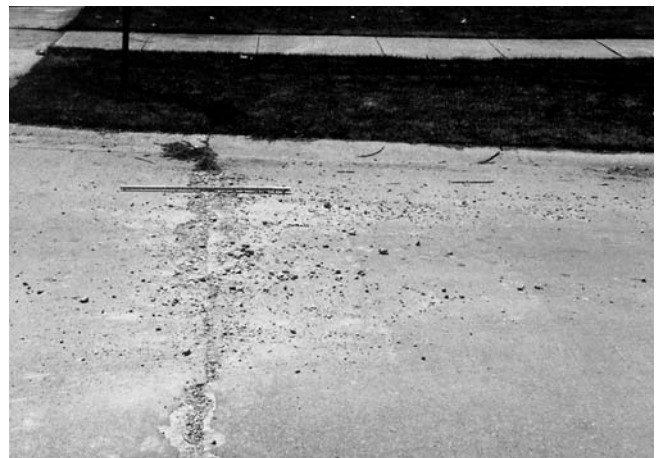
FIG. X2.1 Low-Severity Blowup/Buckling
