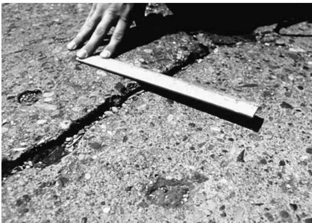
FIG. X2.14 Medium-Severity Faulting
