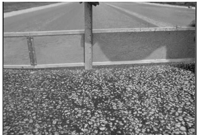
FIG. X1.42 Medium-Severity Rutting
