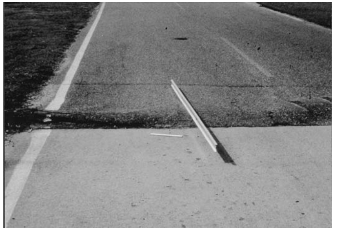
FIG. X1.46 High-Severity Shoving
