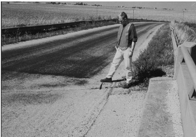
FIG. X1.44 Low-Severity Shoving
