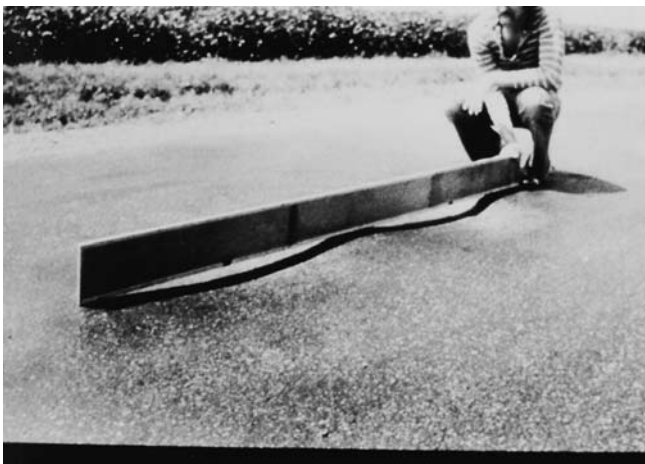
FIG. X1.15 High-Severity Corrugation
