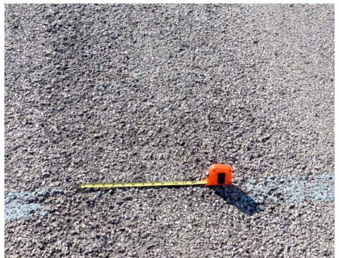
FIG. X1.51 Medium-Severity Raveling
