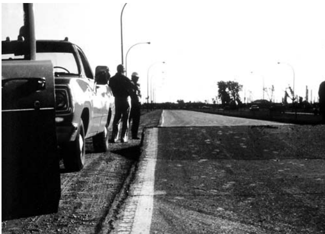
FIG. X2.3 High-Severity Blowup/Buckling
