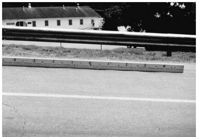
FIG. X1.13 Low-Severity Corrugation
