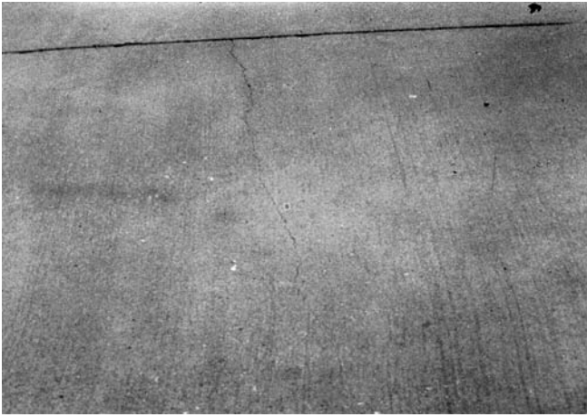
FIG. X2.44 Shrinkage Cracks
