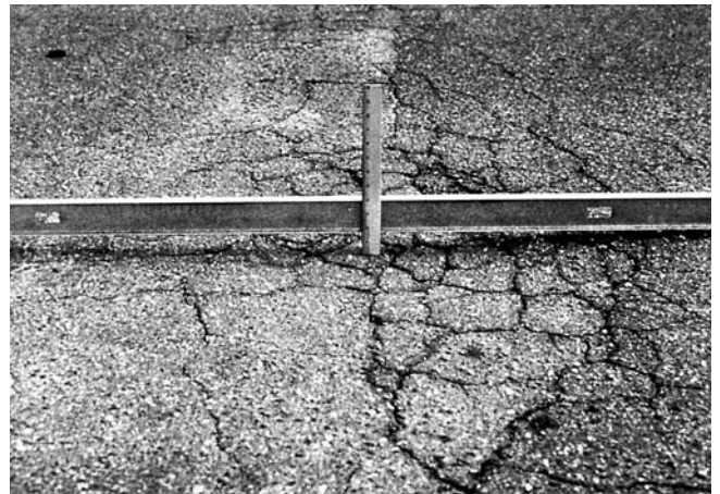
FIG. X1.18 High-Severity Depression
