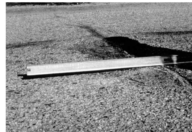
FIG. X1.10 Low-Severity Bumps and Sags
