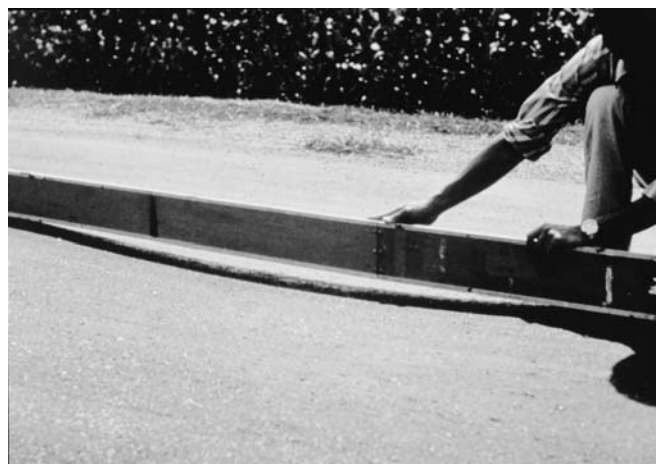
FIG. X1.17 Medium-Severity Depression
