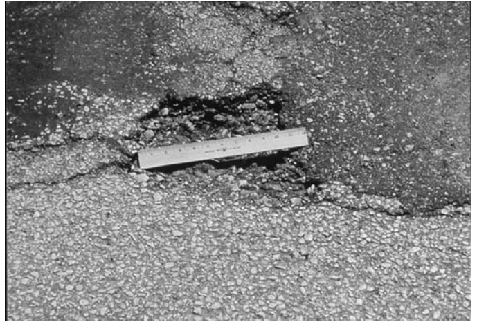
FIG. X1.35 Low-Severity Pothole
