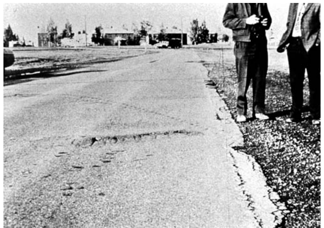
FIG. X1.11 Medium-Severity Bumps and Sags
