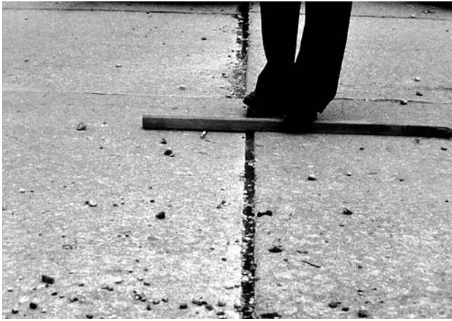
FIG. X2.13 Low-Severity Faulting
