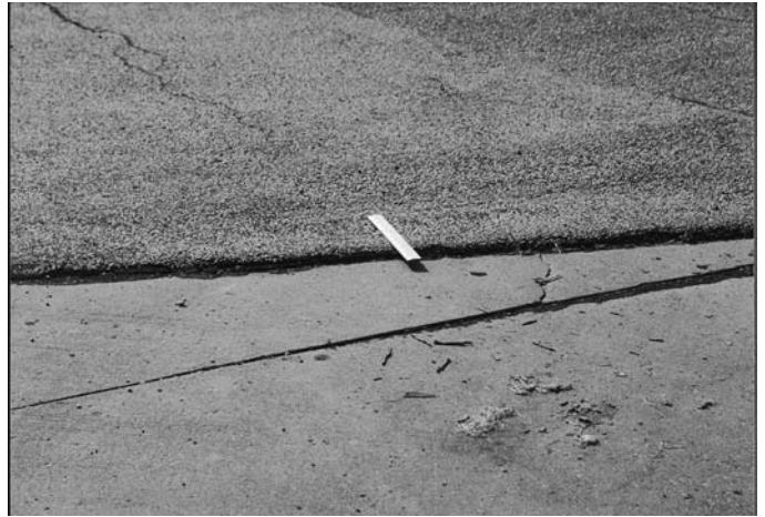
FIG. X1.45 Medium-Severity Shoving
