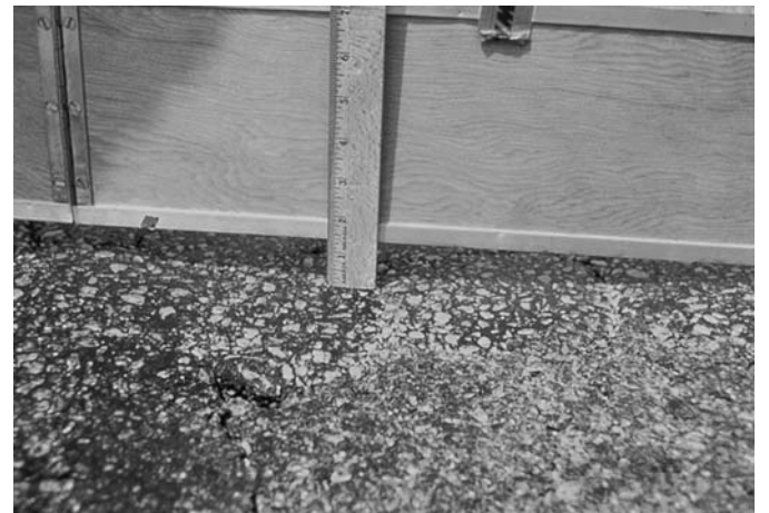
FIG. X1.43 High-Severity Rutting
