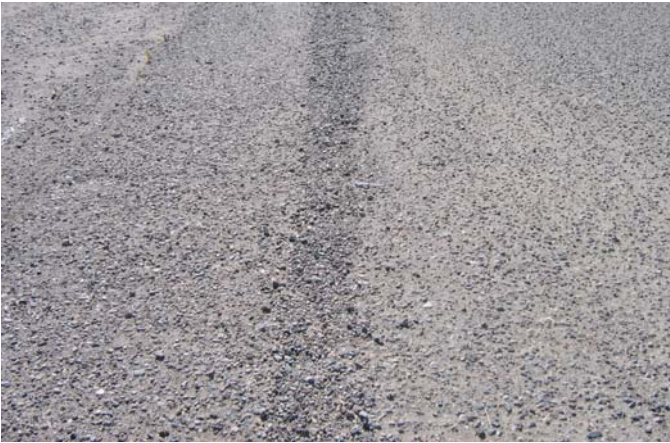
FIG. X1.52 High-Severity Raveling
