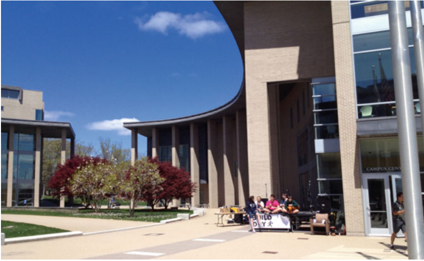
Fig. 4.2 Olin College campus—which includes a circular courtyard surrounded by the academic buildings and student center (right). Students occupy a table for the “Build Day” festivities which were happening during a site visit in 2013
