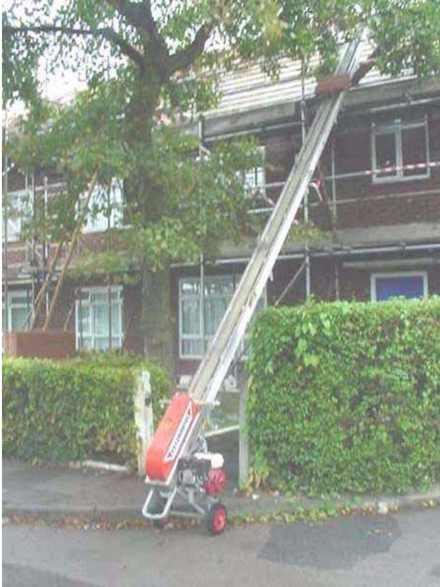
Builder's hoist, with small petrol engine
