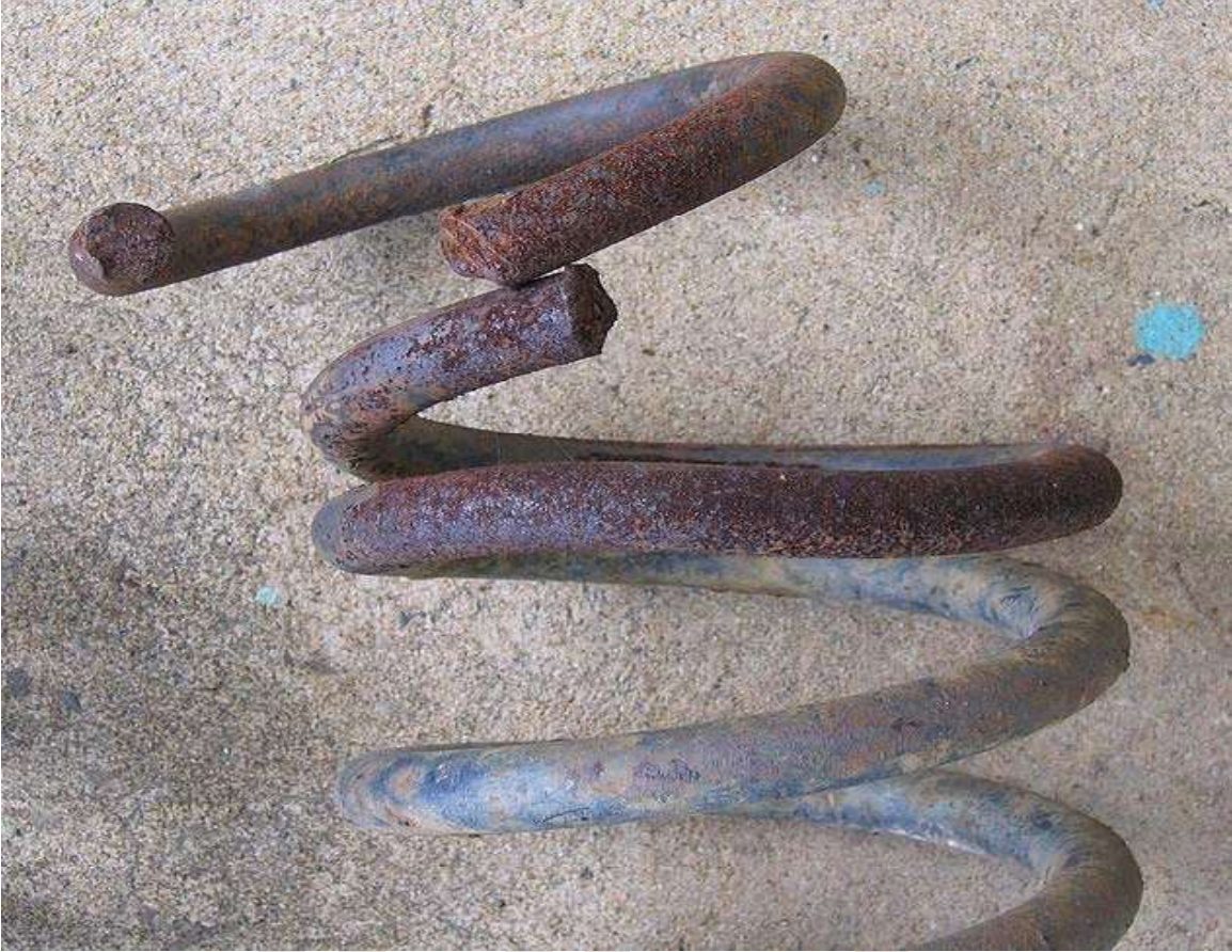
Oxy-cut spring showing deformation due to loss of tempering in adjacent turn
