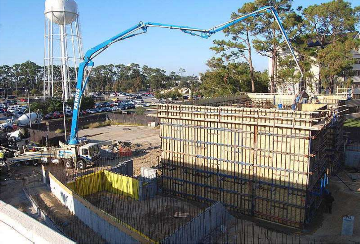
Construction site with concrete pump.
