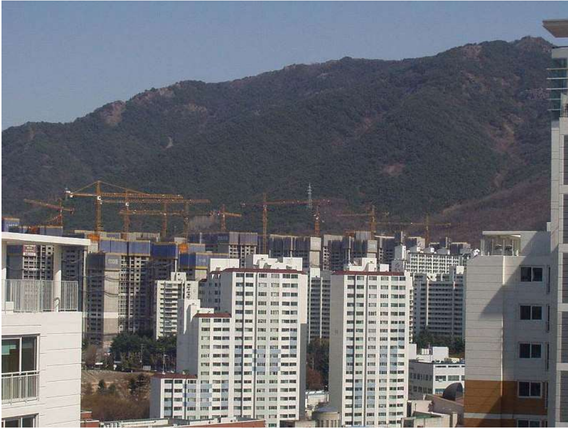
Apartment complex under construction in Daegu, South Korea
