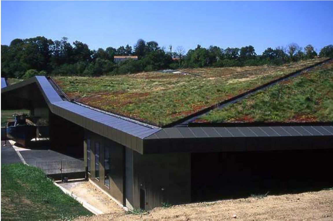
Green roof planted with native species at L'Historial de la Vendée, a new museum in western France
