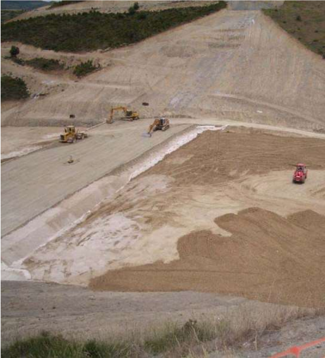
Construction of an Embankment Dam in Navarra, Spain
