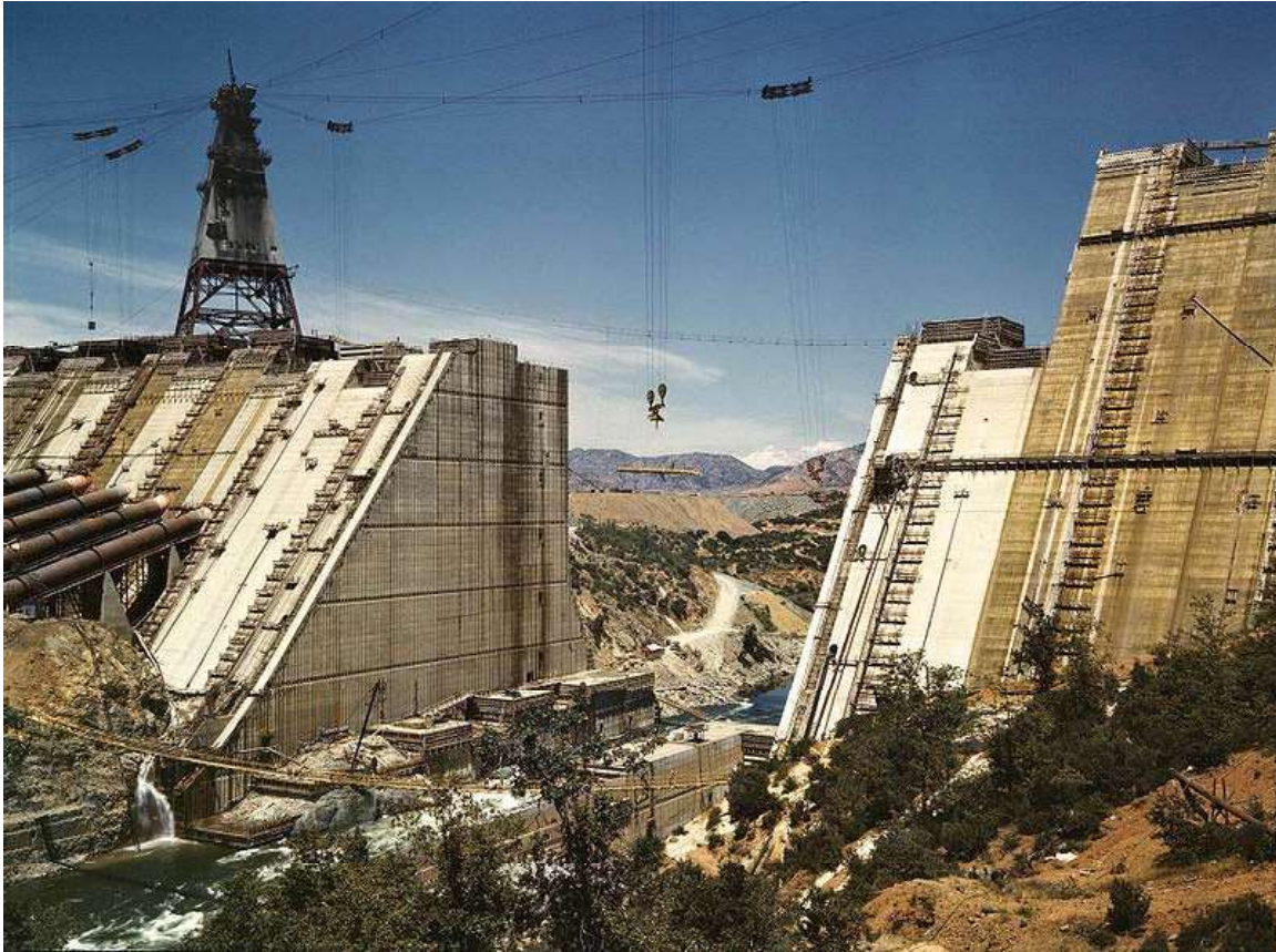
Shasta Dam under construction in June 1942
