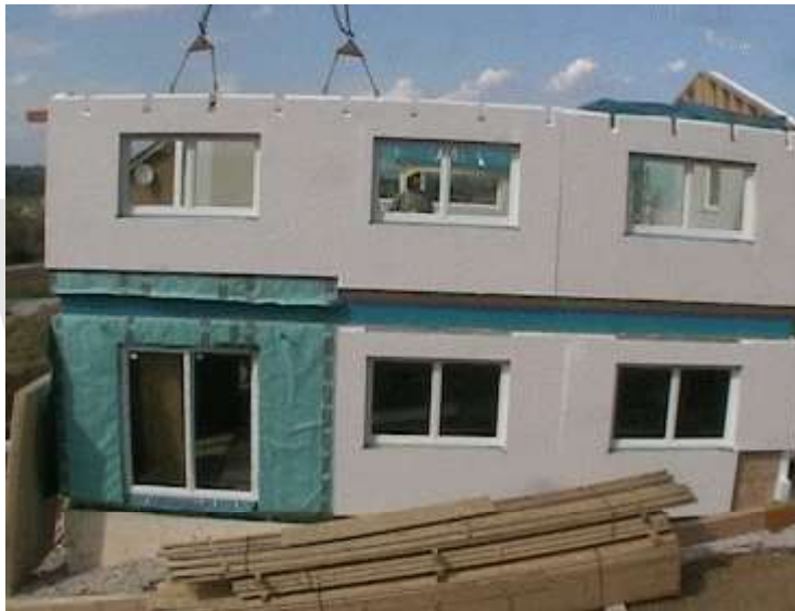
Construction of a prefabricated home
