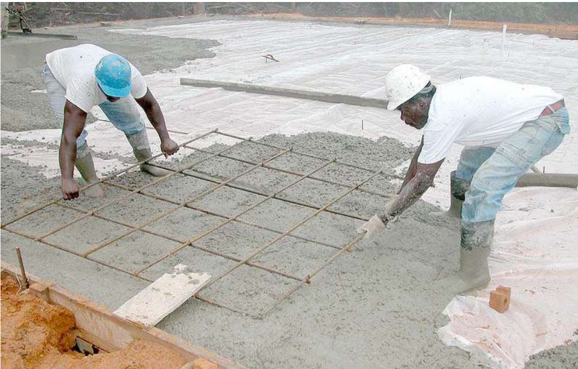
Concrete and metal rebar used to build a floor
