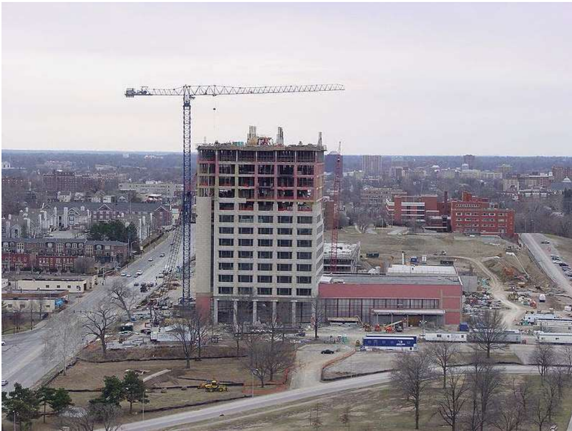
Construction on a building in Kansas City, Missouri
