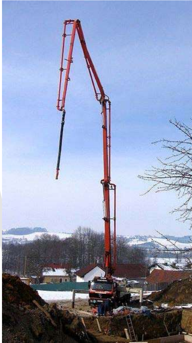
Boom concrete pump
