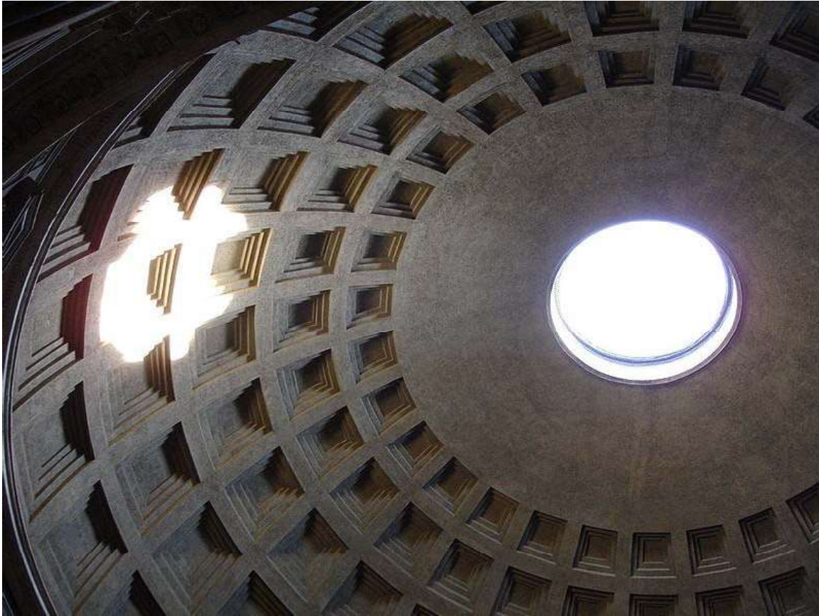
The Pantheon in Rome looking up inside the concrete dome.
