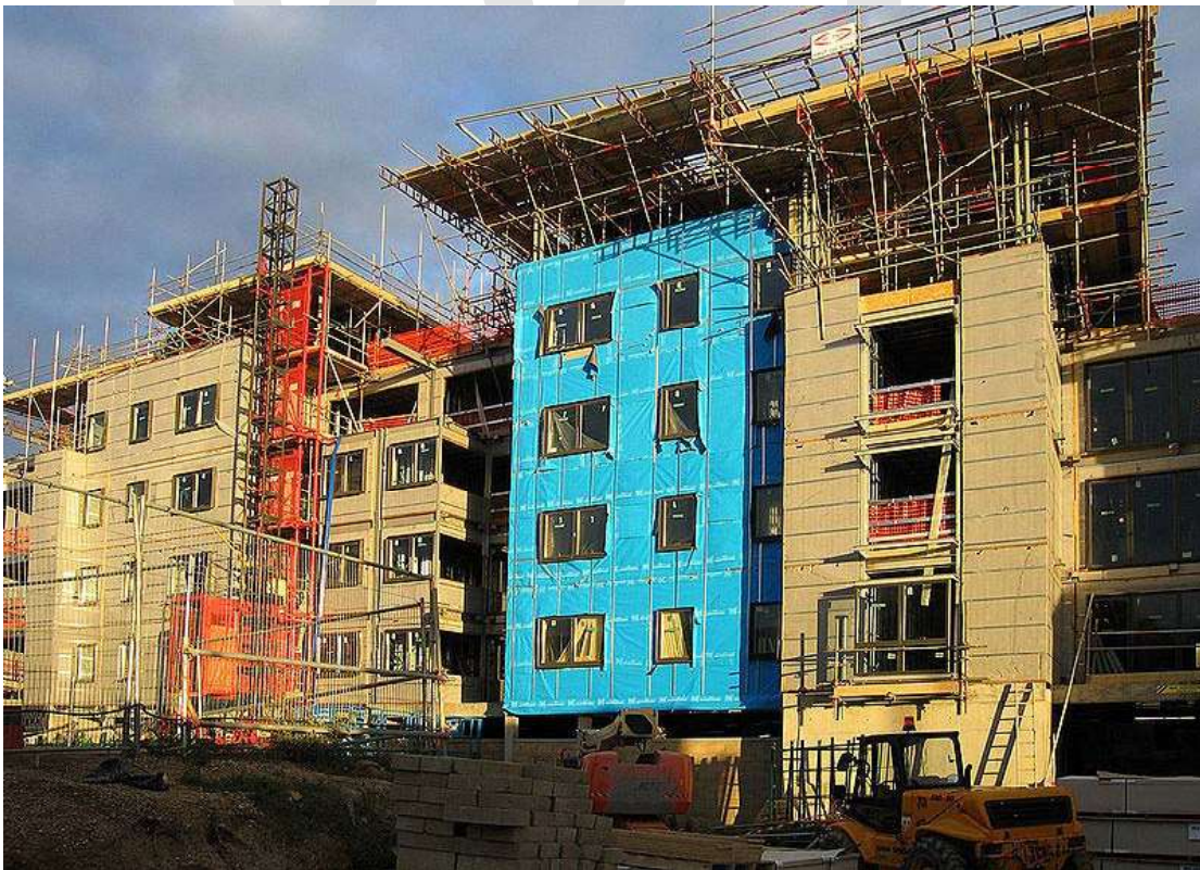
Building construction for several apartment blocks
