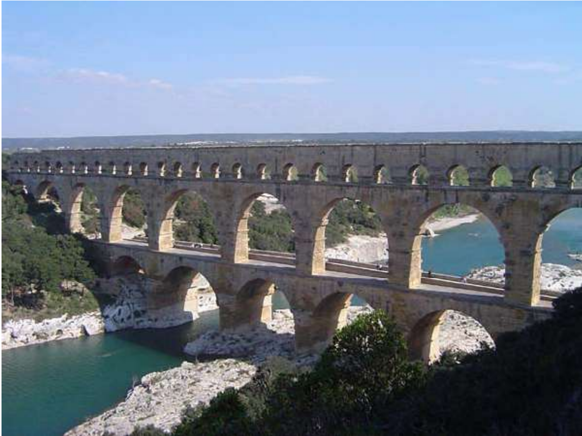
Pont du Gard, France, a Roman aqueduct built circa 19 BC.
