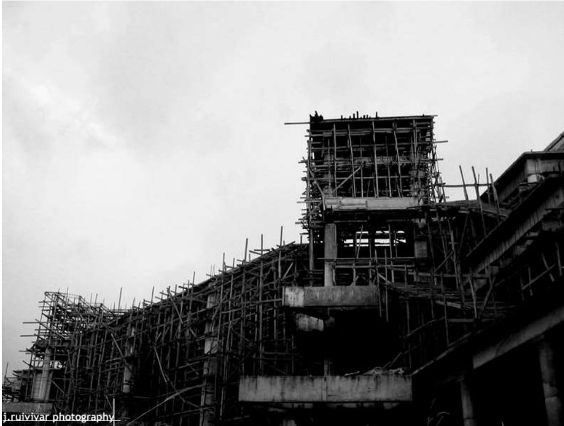
A large unfinished building
