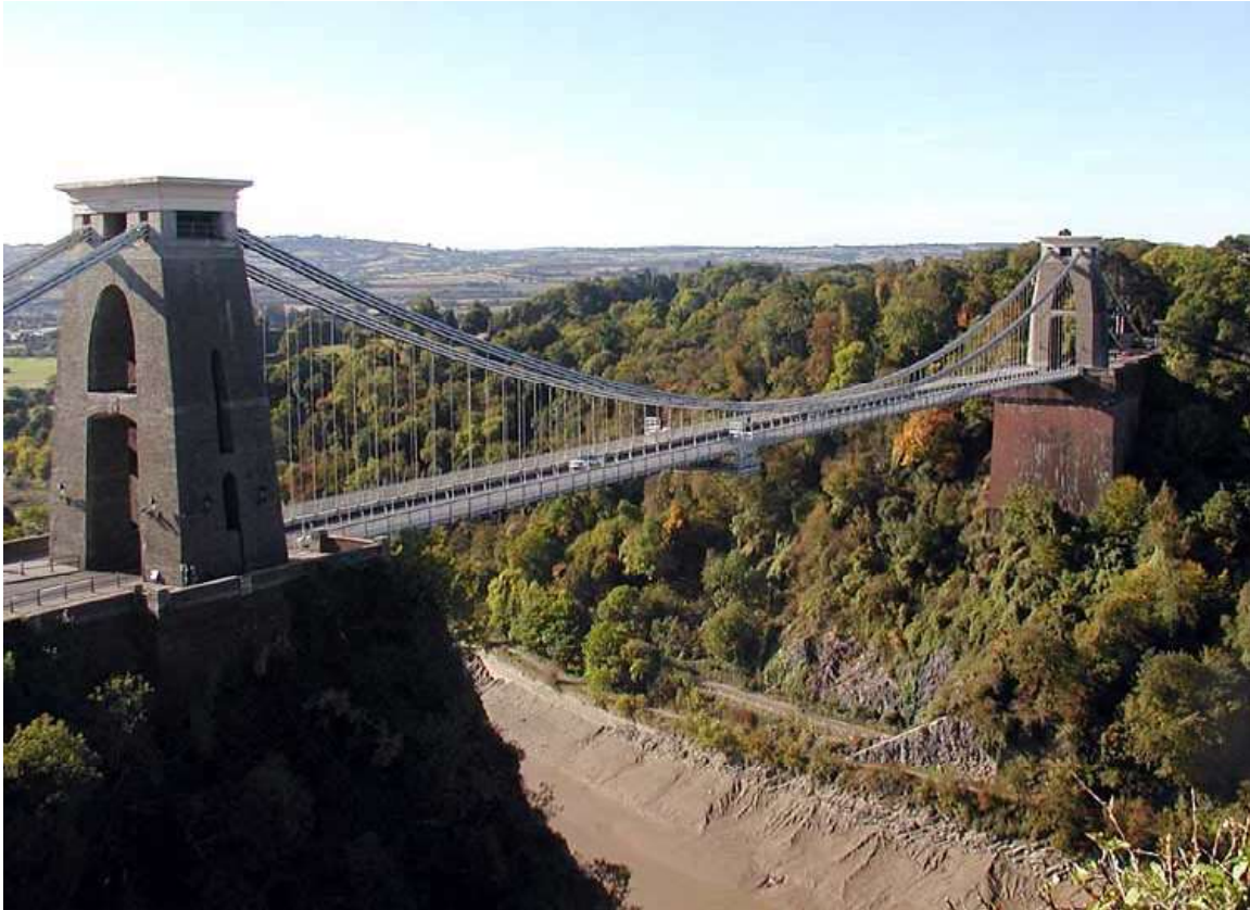
Clifton Suspension Bridge, designed by Isambard Kingdom Brunel, in Bristol, UK
