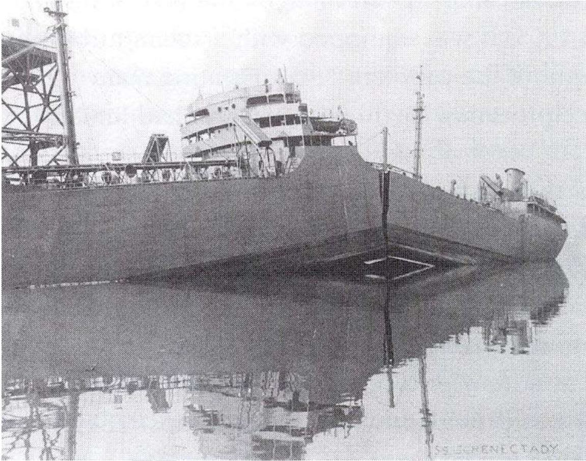
The S.S. Schenectady split apart by brittle fracture while in harbor (1944)
