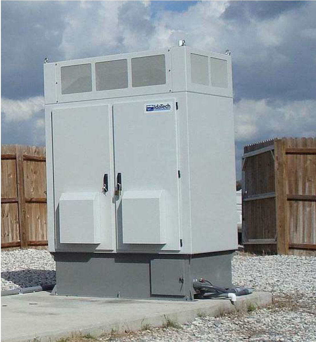
A backup power fuel cell for telecom applications
