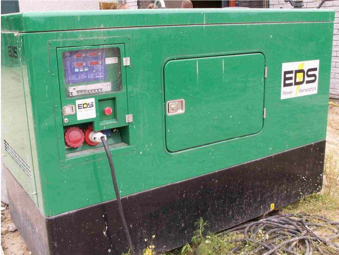
Another generator, powered by fossil fuels and used at a construction site
