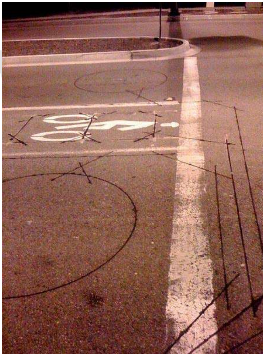
An example of the Inductance loop installed in the road for cars and bikes
