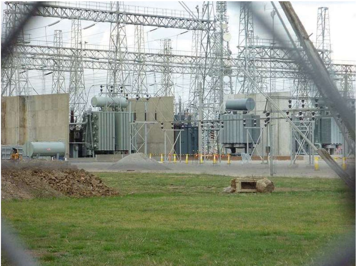
Image of an electrical substation in Melbourne, Australia showing 3 of 5 220kV/66kV transformers, each with a capacity of 185MVA
