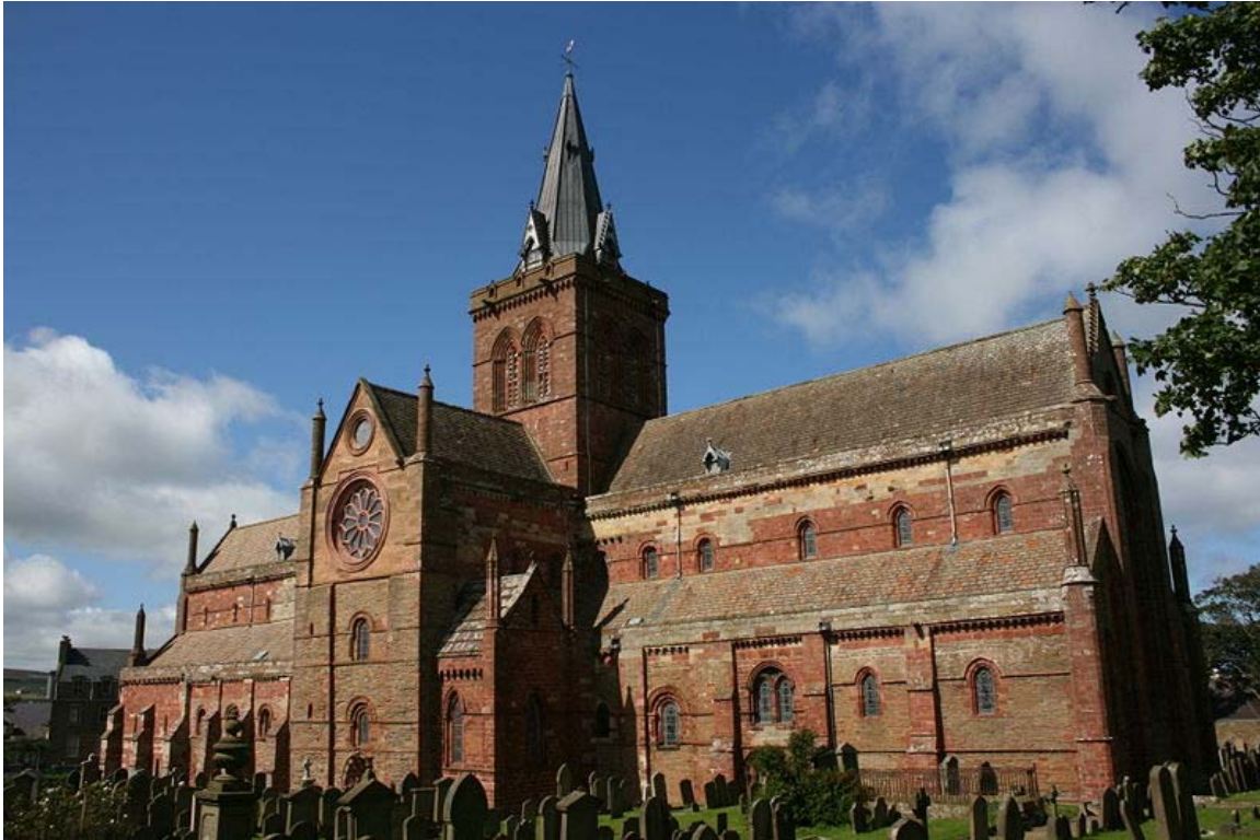
St. Magnus Cathedral, Kirkwall, Orkney, constructed of locally quarried sandstone.
