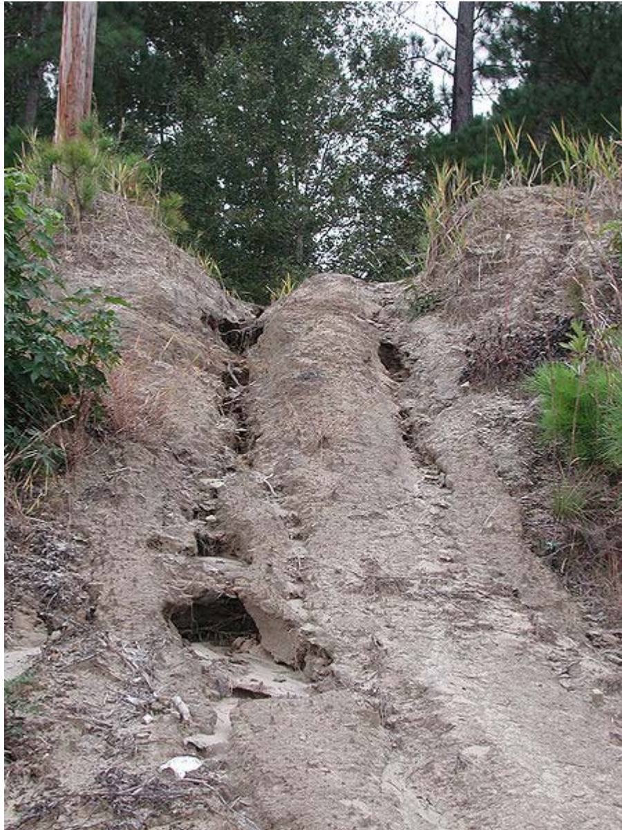
Bank erosion started by four wheeler all-terrain vehicles, Yauhanna, South Carolina
