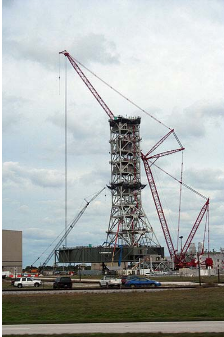
Ares I mobile launch platform under construction
