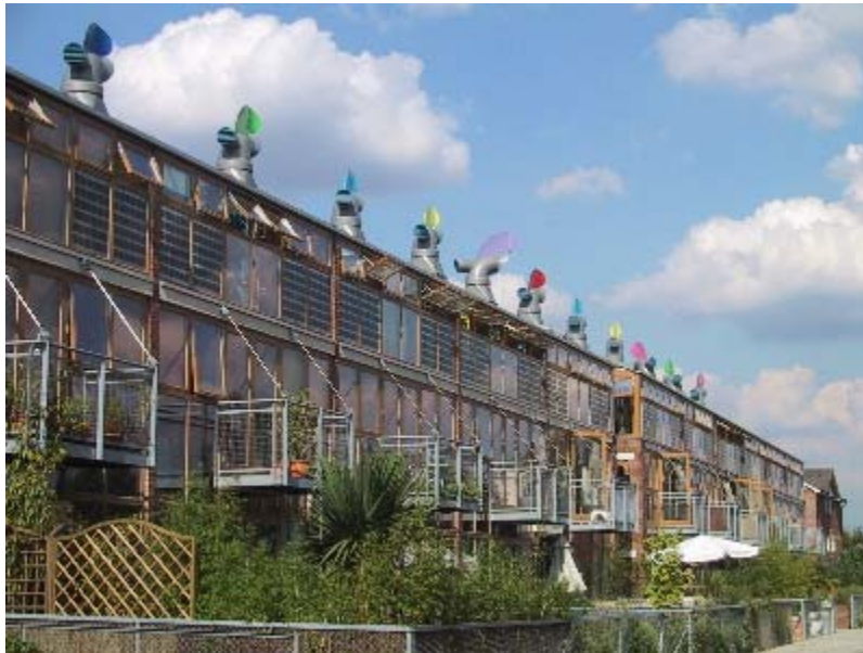
BedZED zero energy housing
