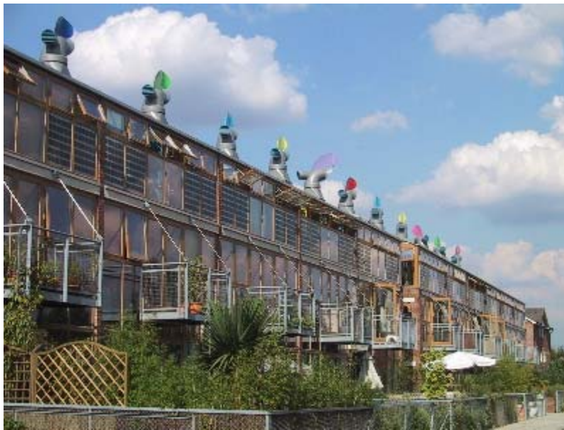
BedZED zero energy housing.
