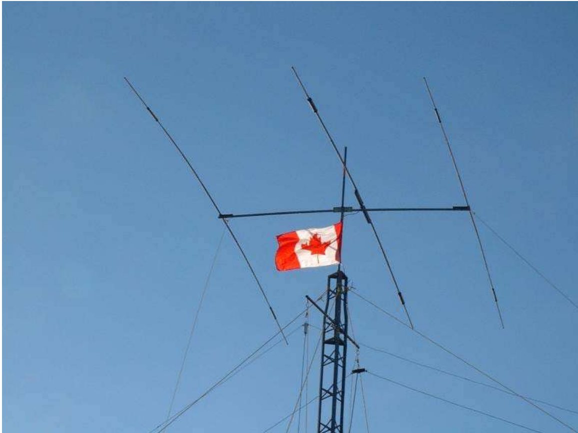
A Yagi-Uda beam antenna
