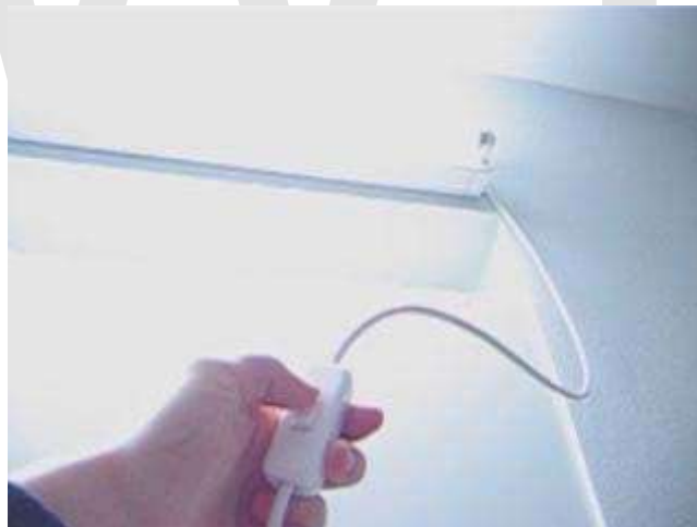
Starting a lamp that has an electronic ballast
