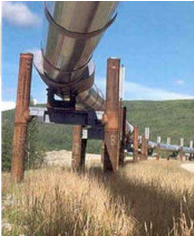
An elevated section of the Alaska Pipeline
