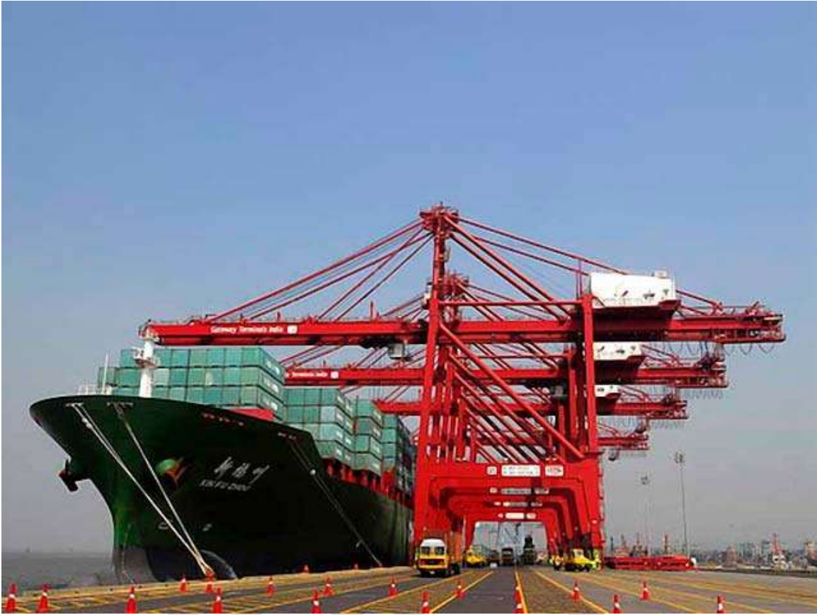
Harbour cranes unload cargo from a container ship at the Jawaharlal Nehru Port in Navi Mumbai, India
