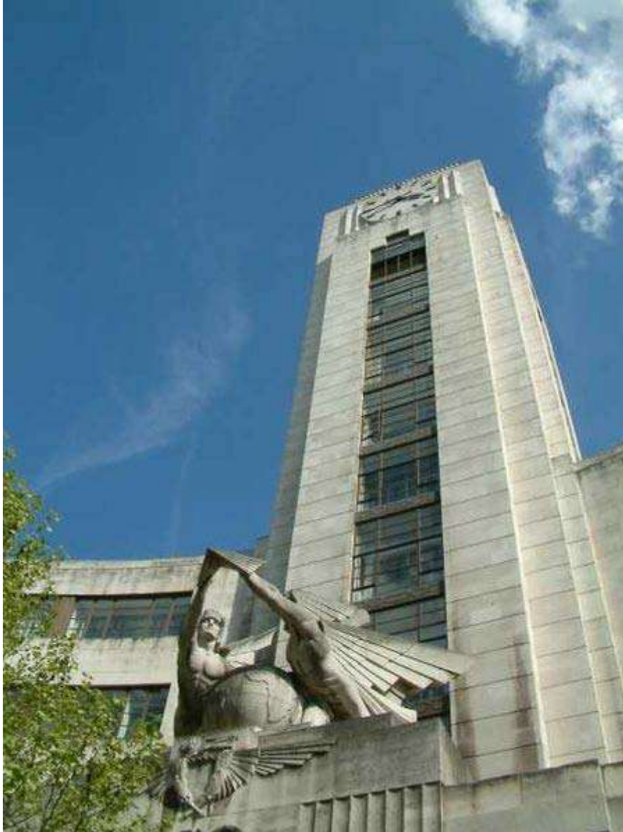
The Imperial Airways Empire Terminal, Victoria, London. Trains ran from here to flying boats in Southampton, and to Croydon Airport.
