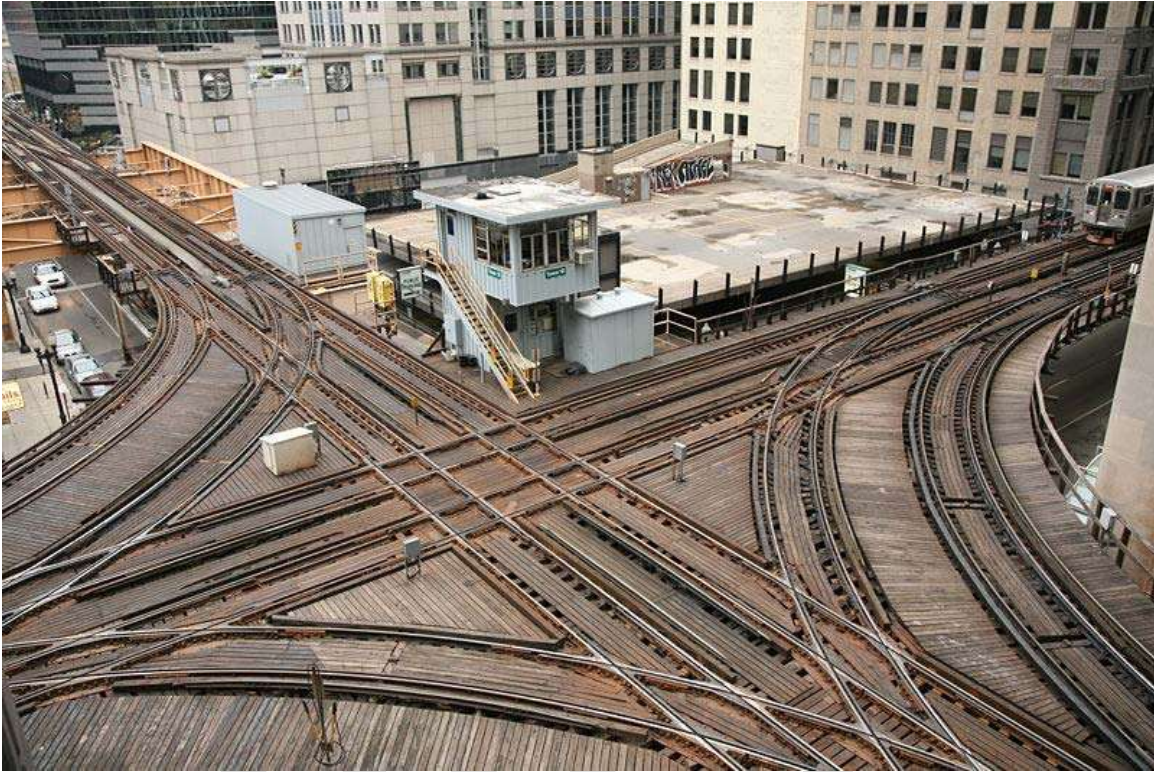
(Up): Tokyo's Yamanote Line, one of the world's busiest commuter rail lines. (Down) Chicago Transit Authority control tower 18 guides elevated Chicago 'L' northbound Purple and Brown lines intersecting with westbound Pink and Green lines and the looping Orange line above the Wells and Lake street intersection in the loop.
