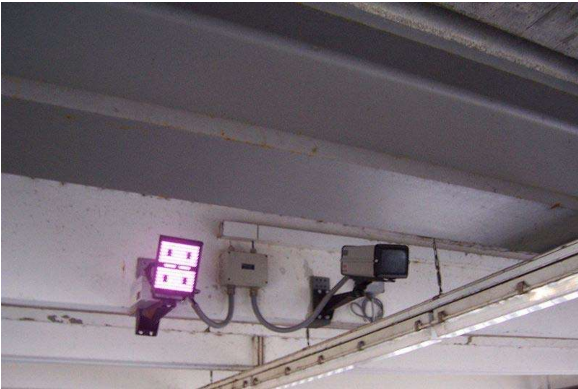
Swiss European surveillance: facial recognition and vehicle make, model, color and license plate reader.
