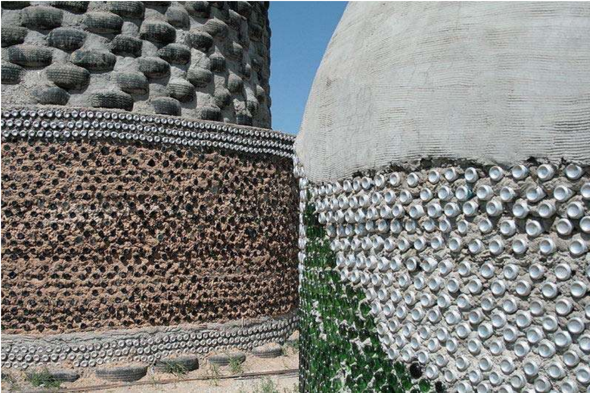
The bottle, can and tire walls of 2 Earthships.
