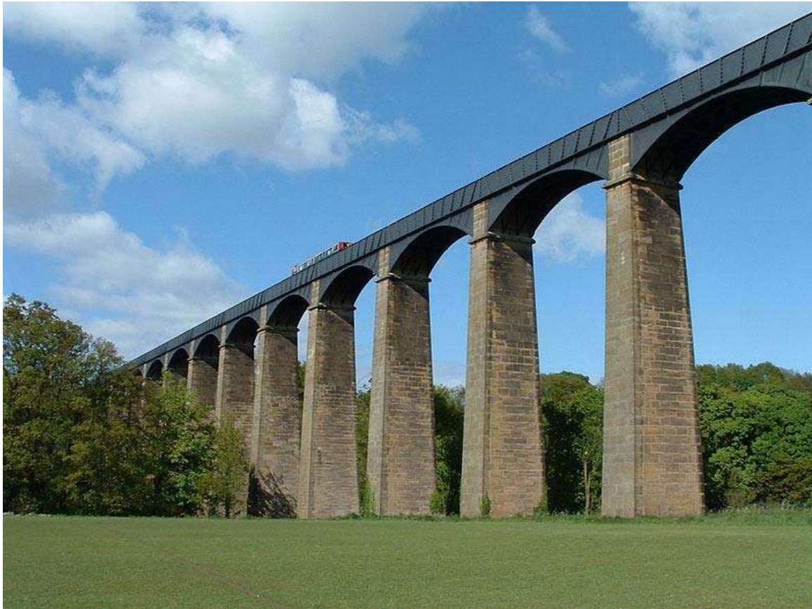
Pontcysyllte Aqueduct, Llangollen, Wales
