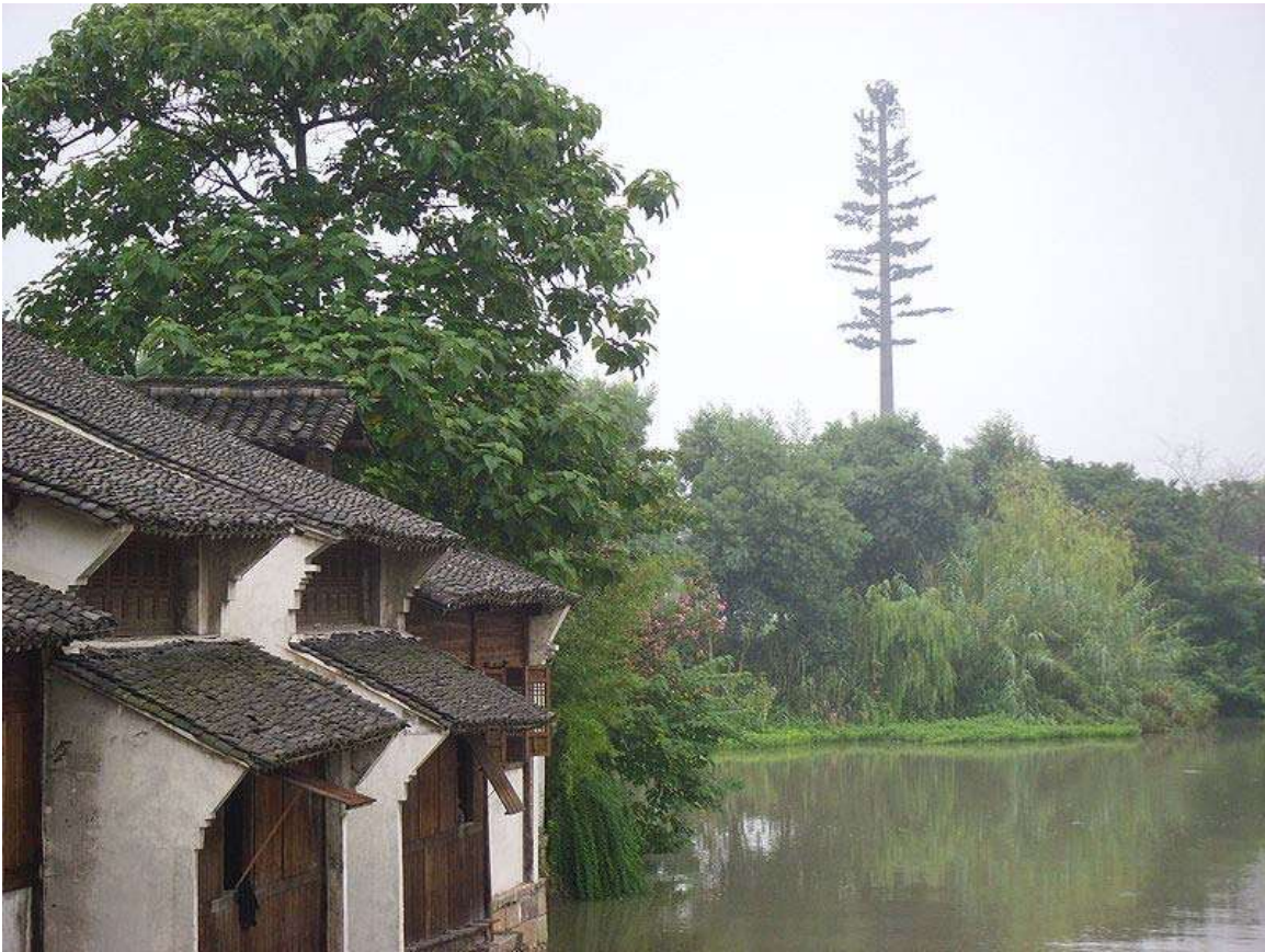
Communications tower, camouflaged as a slim tree
