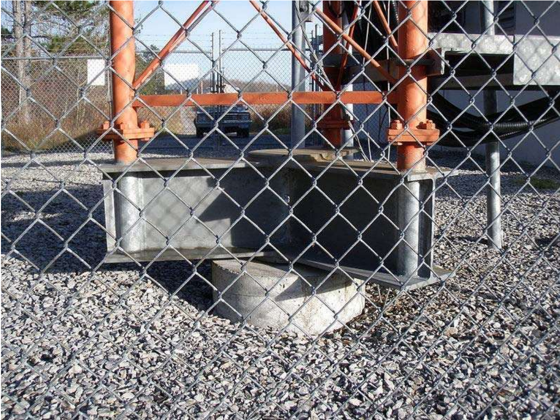
A radio mast base showing how virtually all support is provided by the guy-wires
