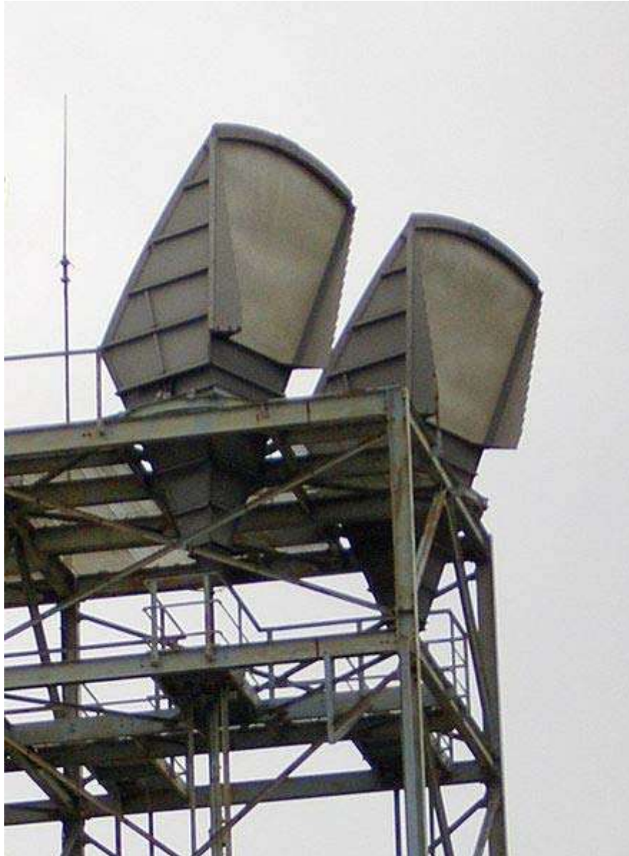
Hogg microwave relay antennas on roof of AT&T telephone switching center, Seattle, Washington, USA Hogg antennas
