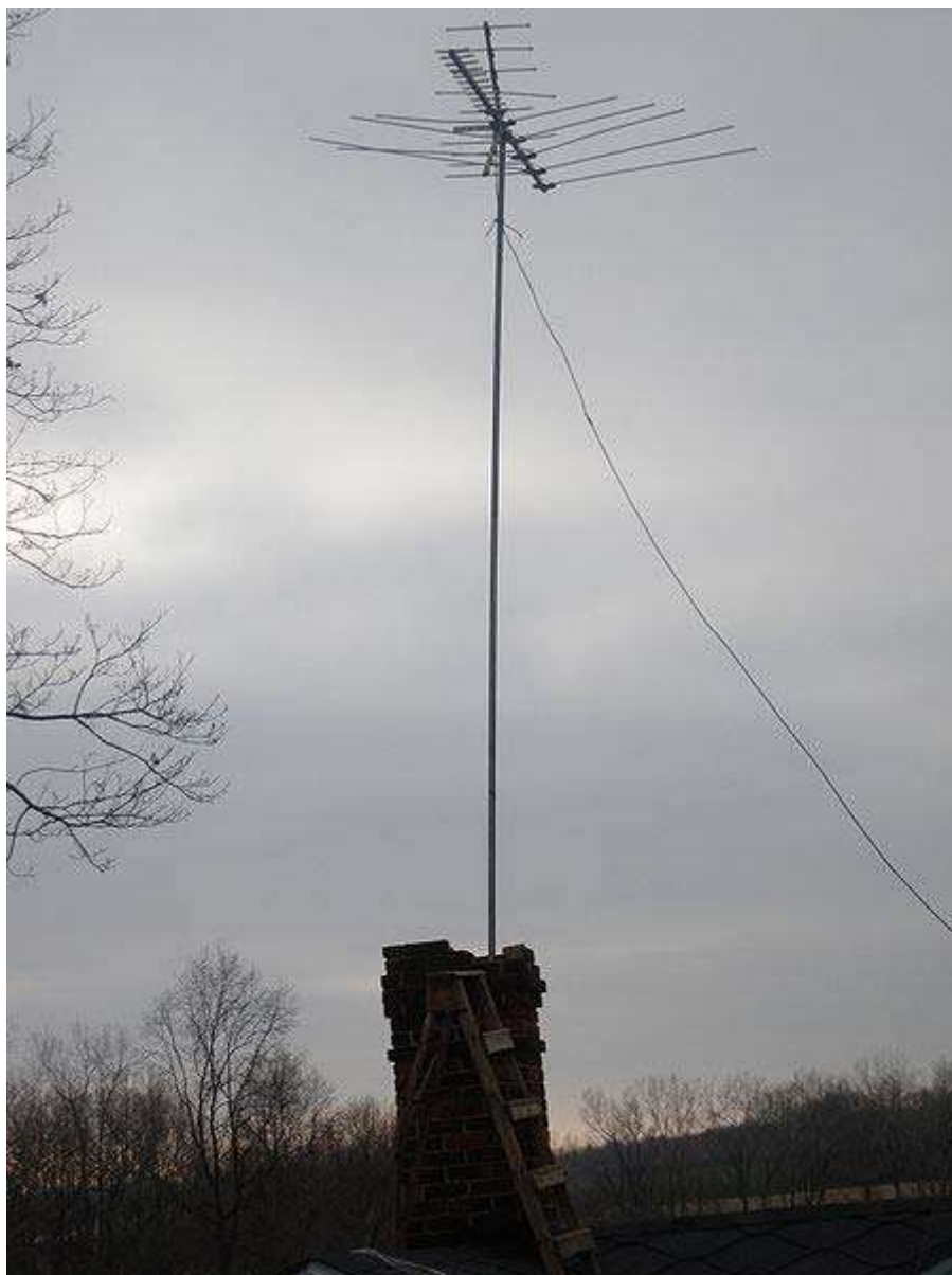
An antenna pole setup in a chimney, reaching 35 feet (10.7 meters) off the ground
