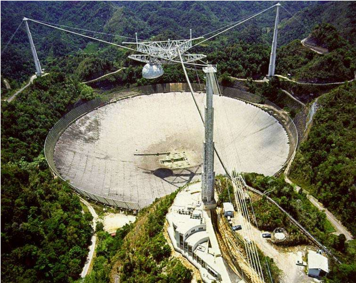
The largest dish antenna in the world, the radio telescope at Arecibo Observatory, Puerto Rico, 305 meters (1000 feet) in diameter. It has a gain of 10 million, or 70 dBi, at 2.38 GHz.
