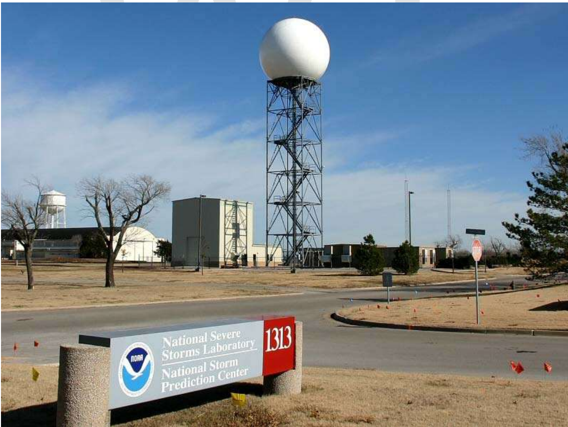
NEXRAD Radar at the WSR-88D Radar Operations Center
