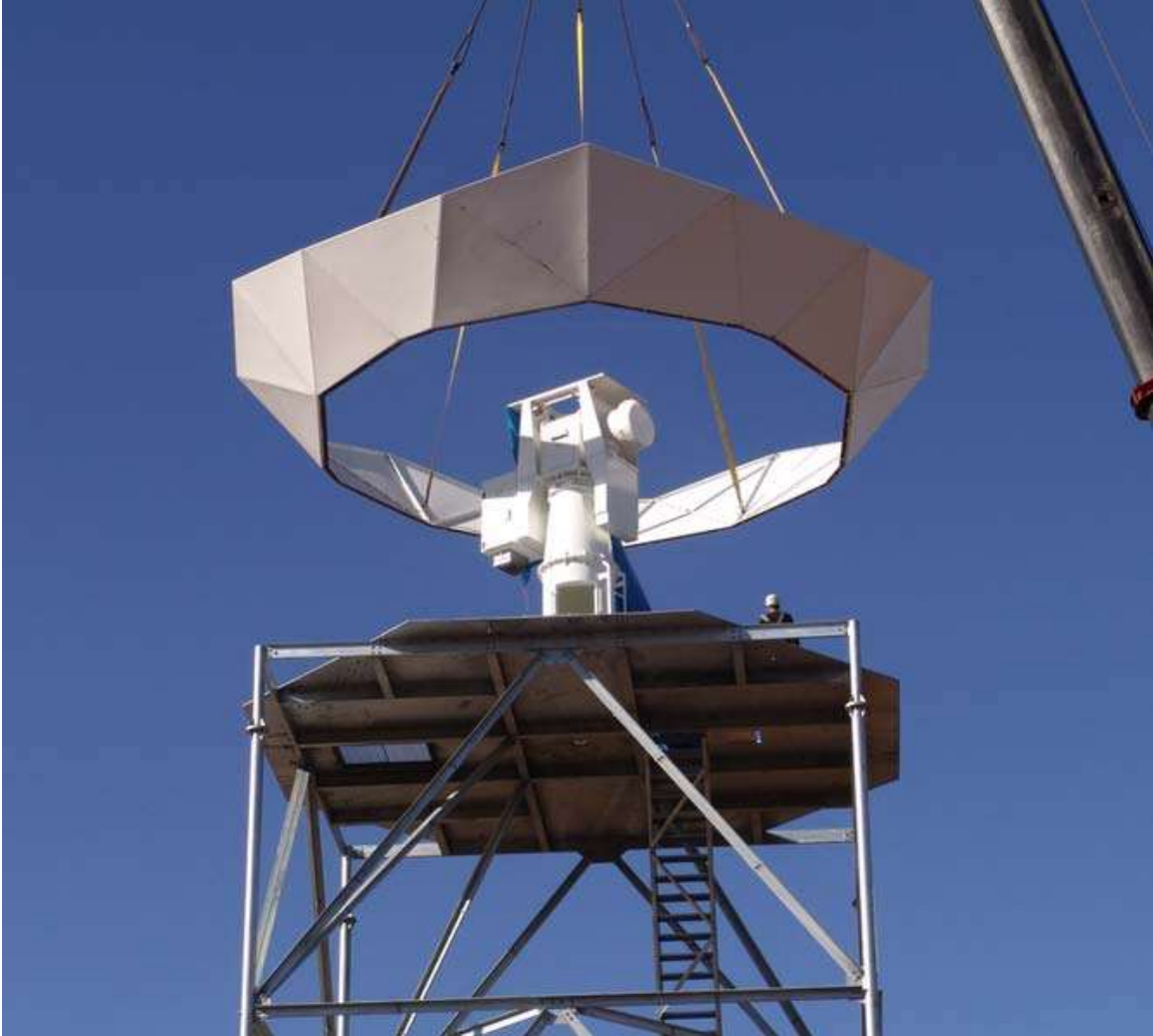
Lifting of radome base for OU-PRIME
