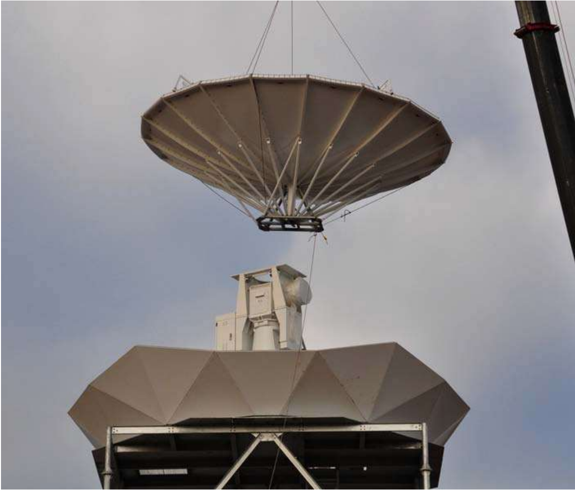
Installation of 8.5-meter dish for OU-PRIME
