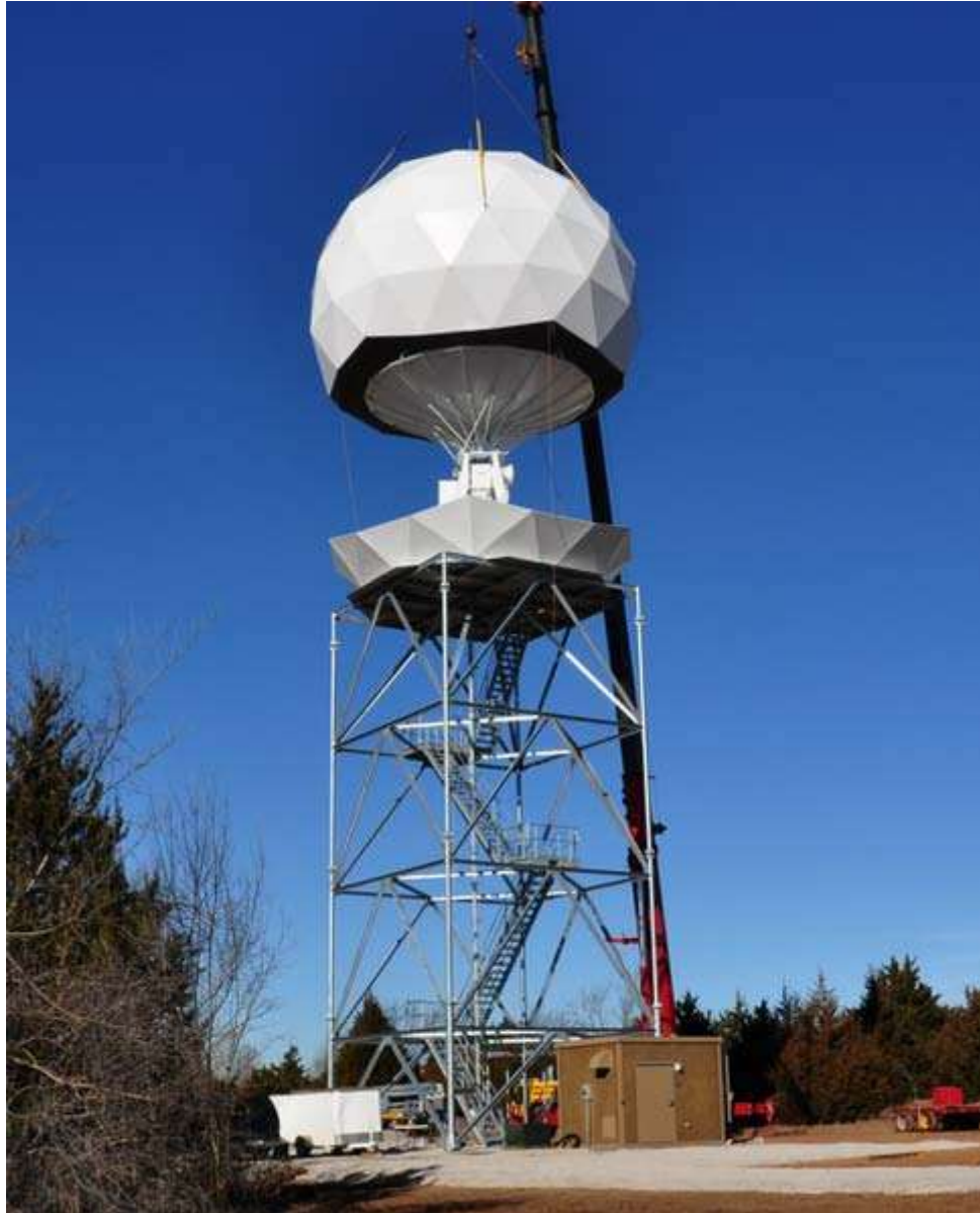
University of Oklahoma OU-PRIME C-band, polarimetric, weather radar during construction
