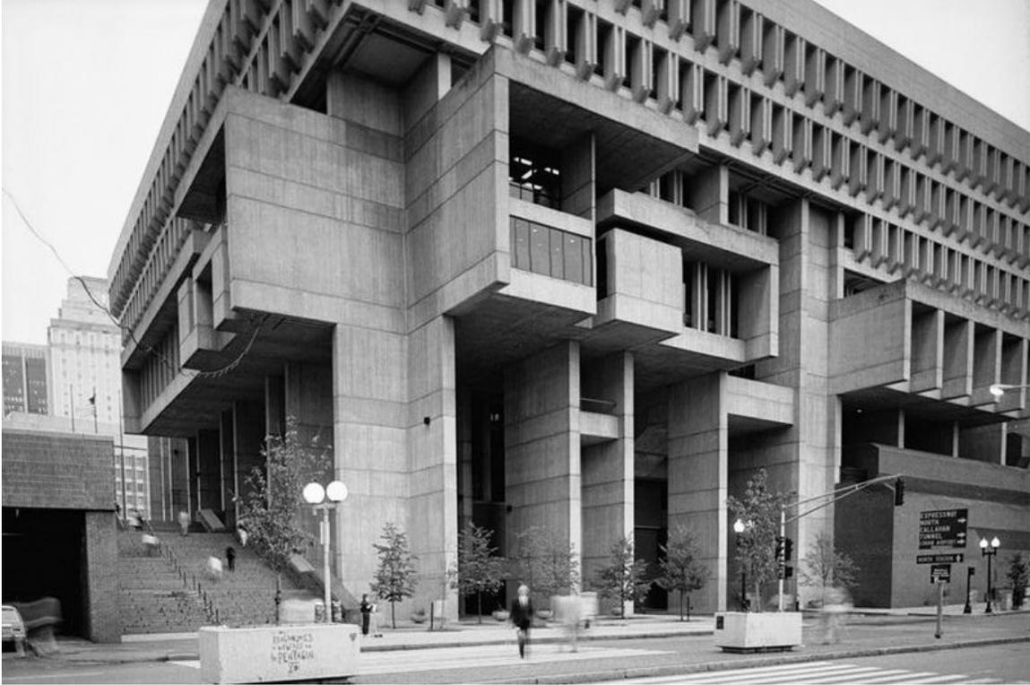
A modern building: Boston City Hall (completed 1968) is largely constructed of concrete, both pre-cast and poured-in-place.
