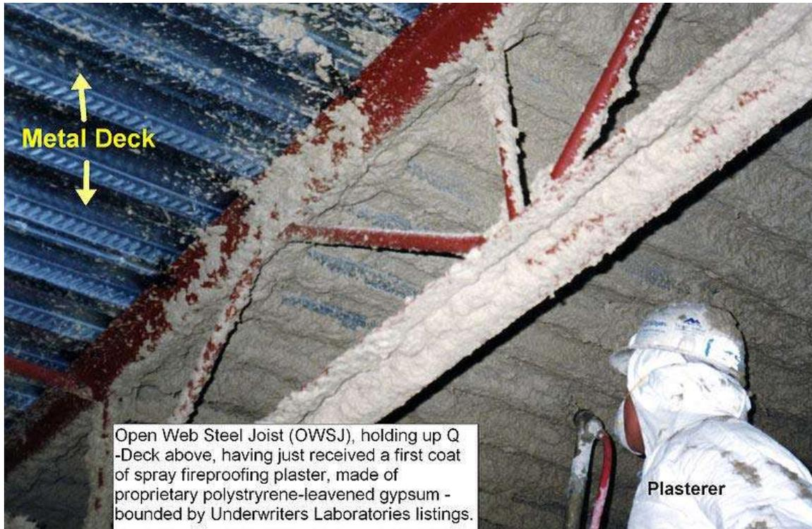
Metal deck and OWSJ (Open Web Steel Joist), receiving first coat of spray fireproofing plaster, made of polystyrene leavened gypsum.
