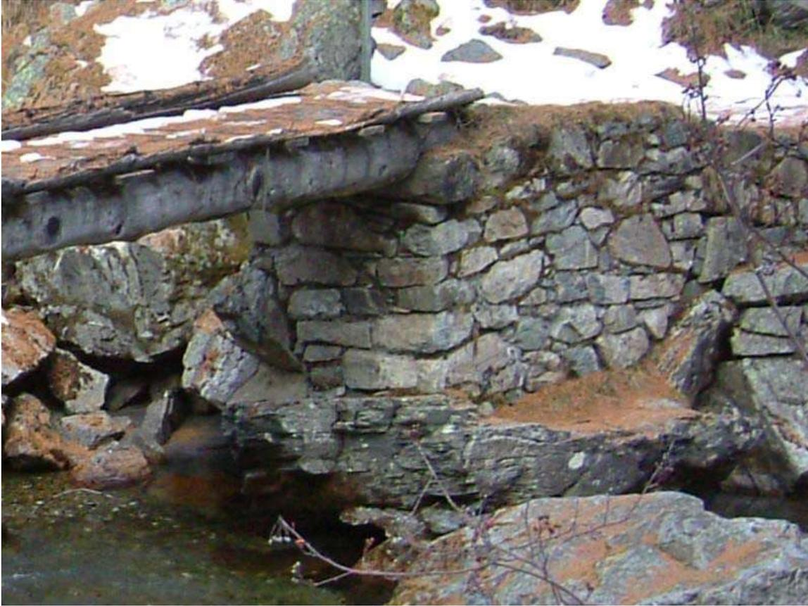
Dry set masonry supports a rustic log bridge, where it provides a well-drained support for the log (this will increase its service life).
