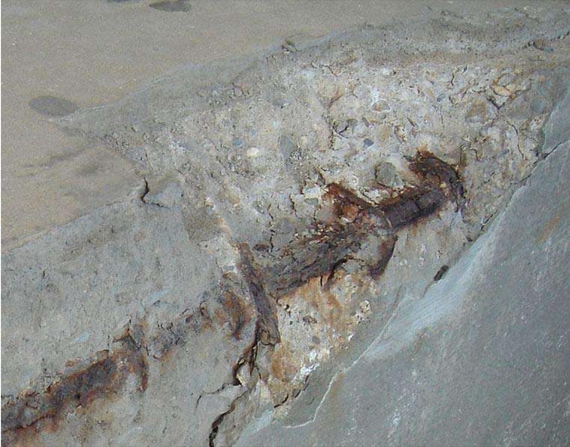
Concrete spalling caused by the corrosion of reinforcement bars after that carbonation of cement decreased the pH below the passivation threshold for steel.
