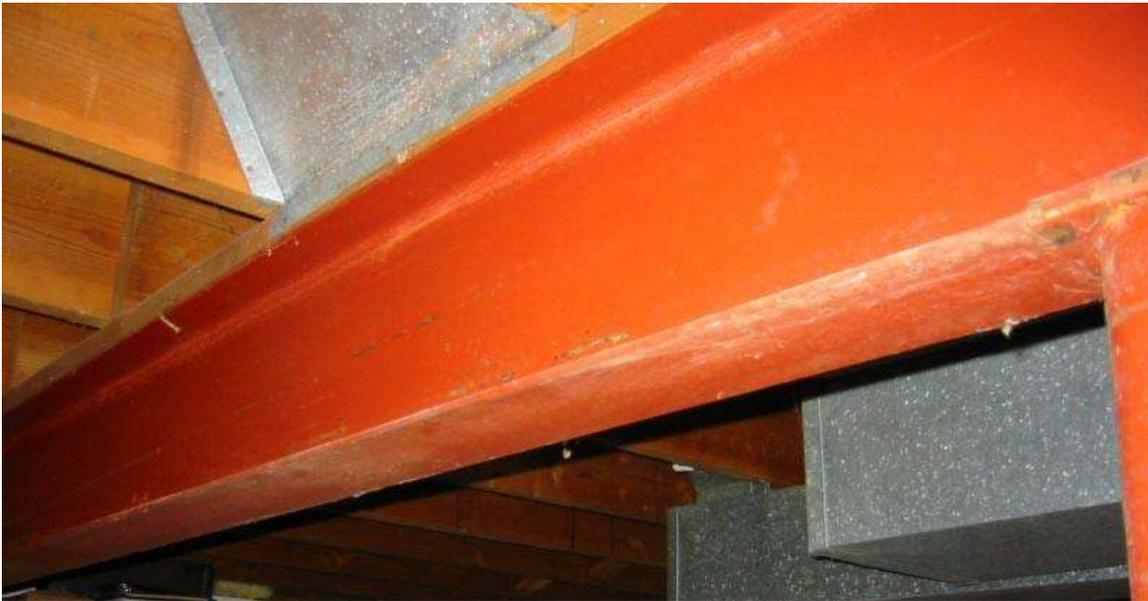
A steel I-beam, in this case used to support wood beams in a house
