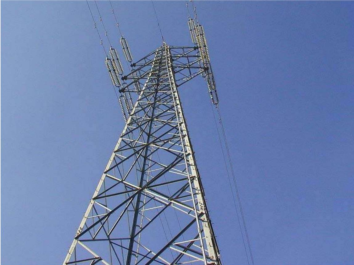
A steel pylon suspending overhead powerlines
