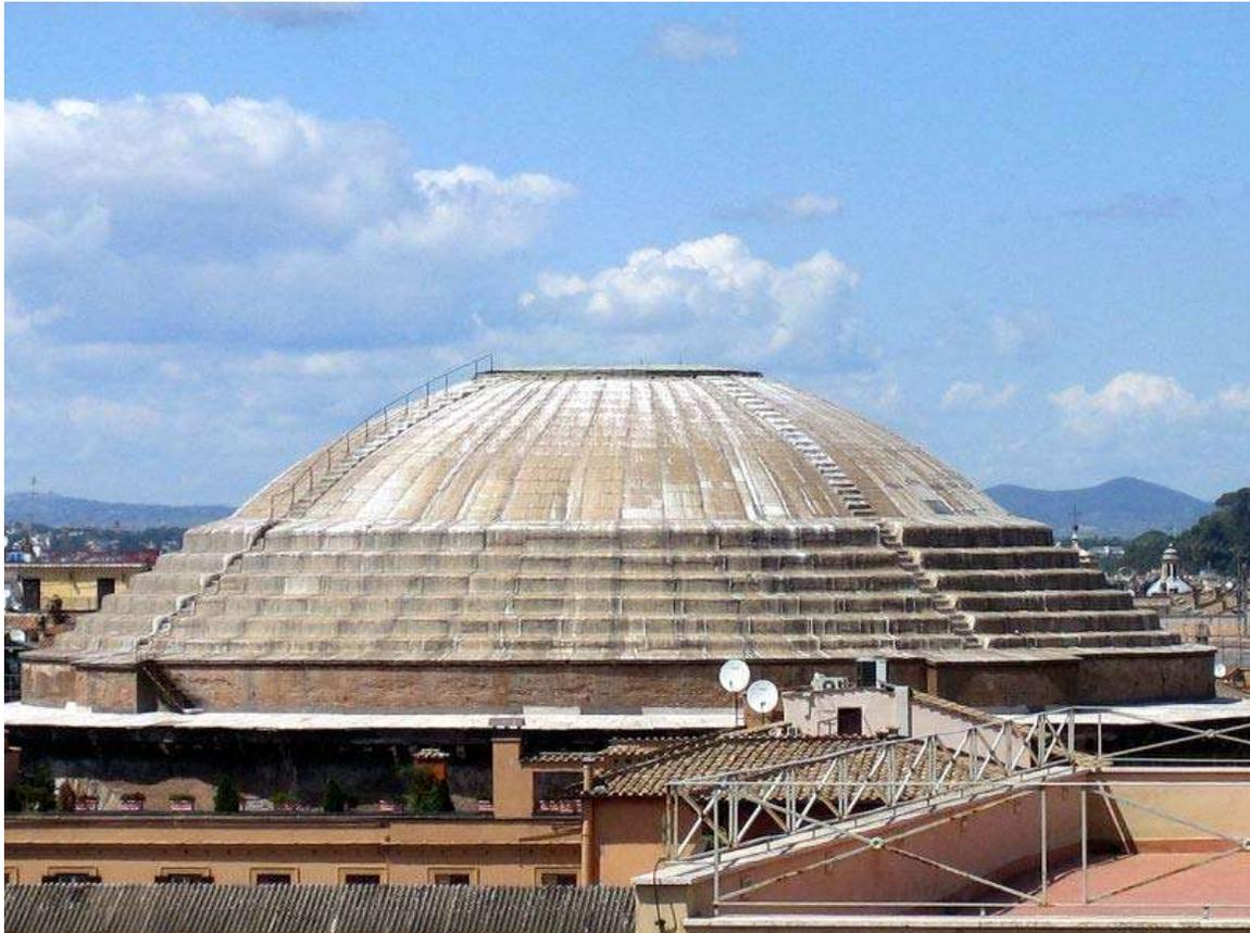
Outer view of the Roman Pantheon, still the largest unreinforced solid concrete dome
