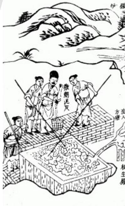
The puddling process of smelting iron ore to make wrought iron from pig iron, the right half of the illustration (not shown) displays men working a blast furnace, *Tiangong Kaiwu* encyclopedia published in 1637, written by Song Yingxing (1587–1666).
