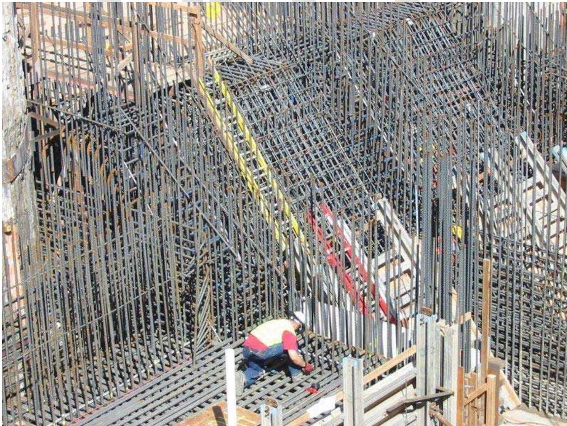
Rebar for foundations and walls of sewage pump station
