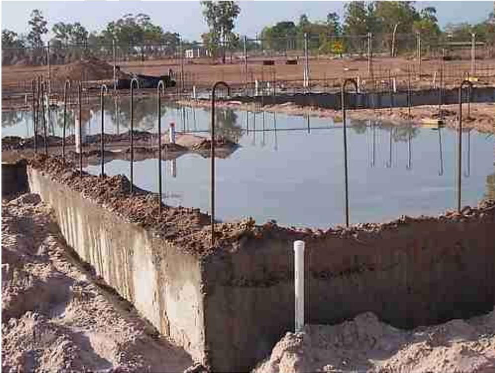
A concrete slab ponded while curing
