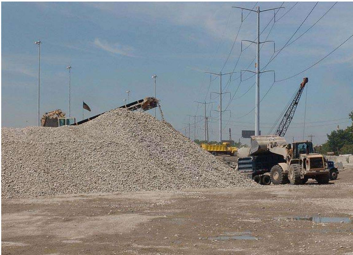
Recycled crushed concrete being loaded into a semi-dump truck to be used as granular fill.
