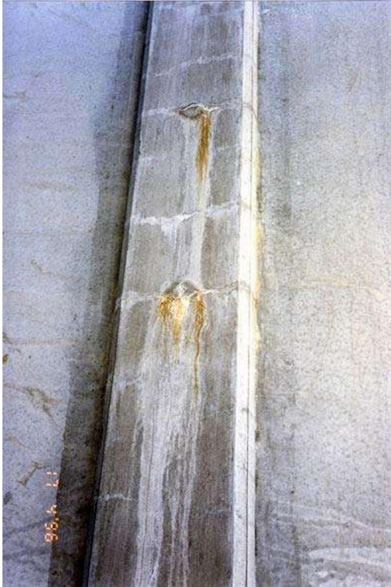
Secondary efflorescence: Water seeping through the concrete, often in cracks, having dissolved components of cement stone. Osteoporosis of concrete often happens in parking garages, as road salt comes off cars to the concrete floor as a saline solution in the winter.
