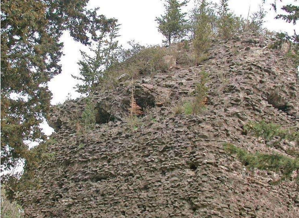
*Opus caementicium* laying bare on a tomb near Rome. In contrast to modern concrete structures, the concrete walls of Roman buildings were covered, usually with brick or stone.
