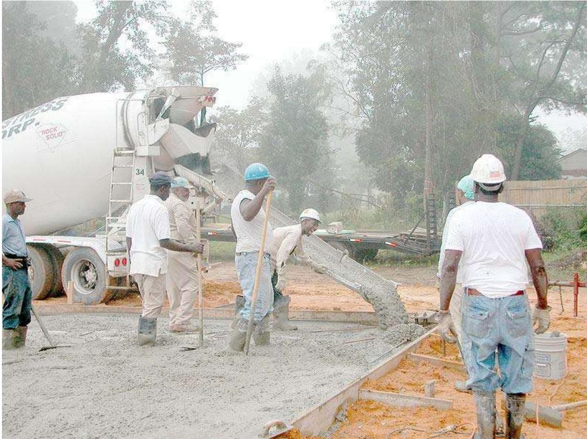
Pouring a concrete floor for a commercial building, *slab-on-ground*
