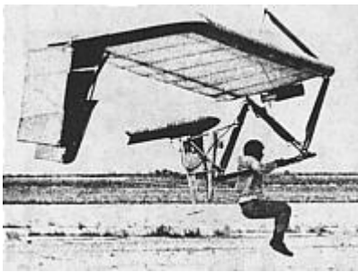
Icarus V hang glider powered with a G8-2 rocket engine, 1979.
