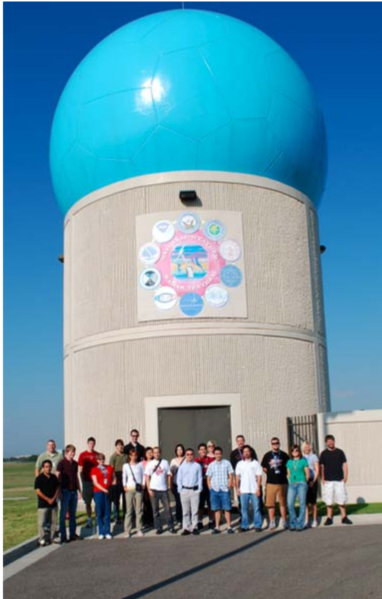
Phased Array Weather Radar in Norman, Oklahoma
