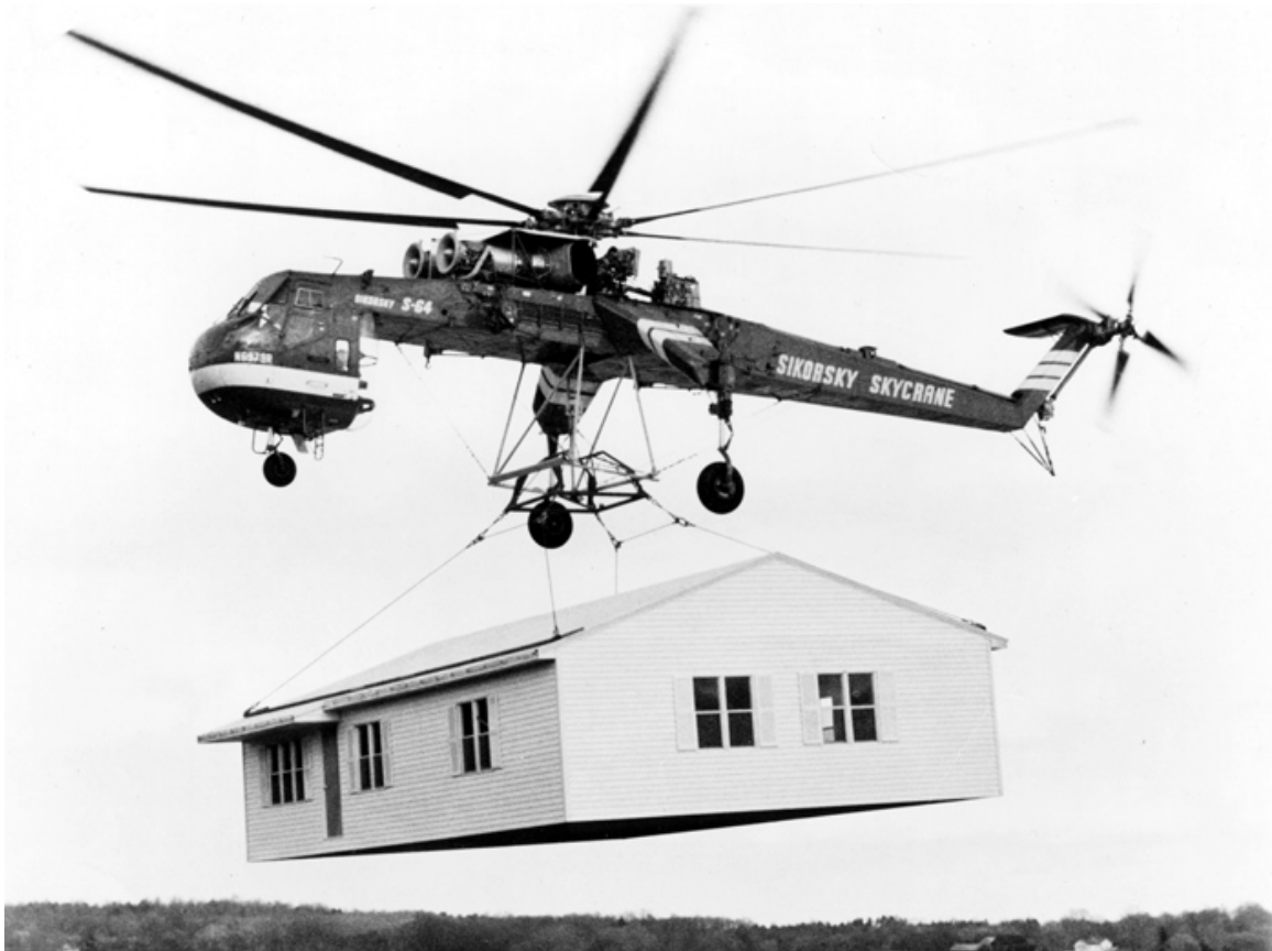
Sikorsky S-64 Skycrane lifting a prefab house
