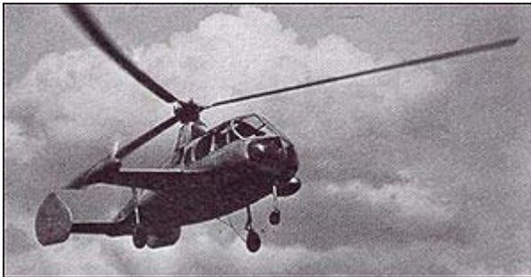
The Fairey FB-1 Gyrodyne prototype in test
