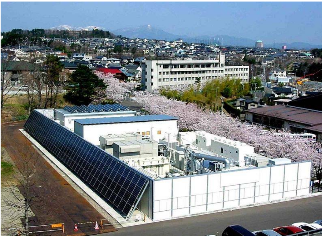
Picture of a local microgrid
