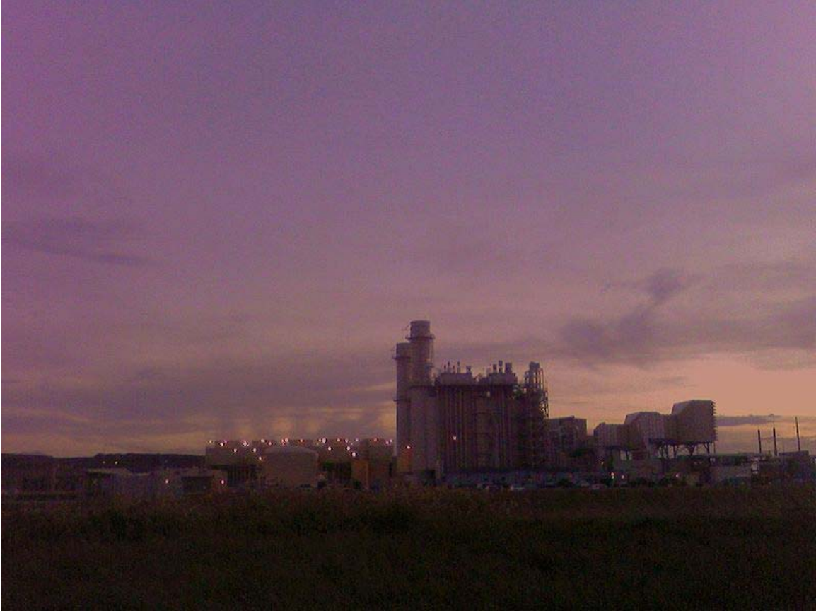
A combined cycle natural gas power plant near Orem, Utah.
