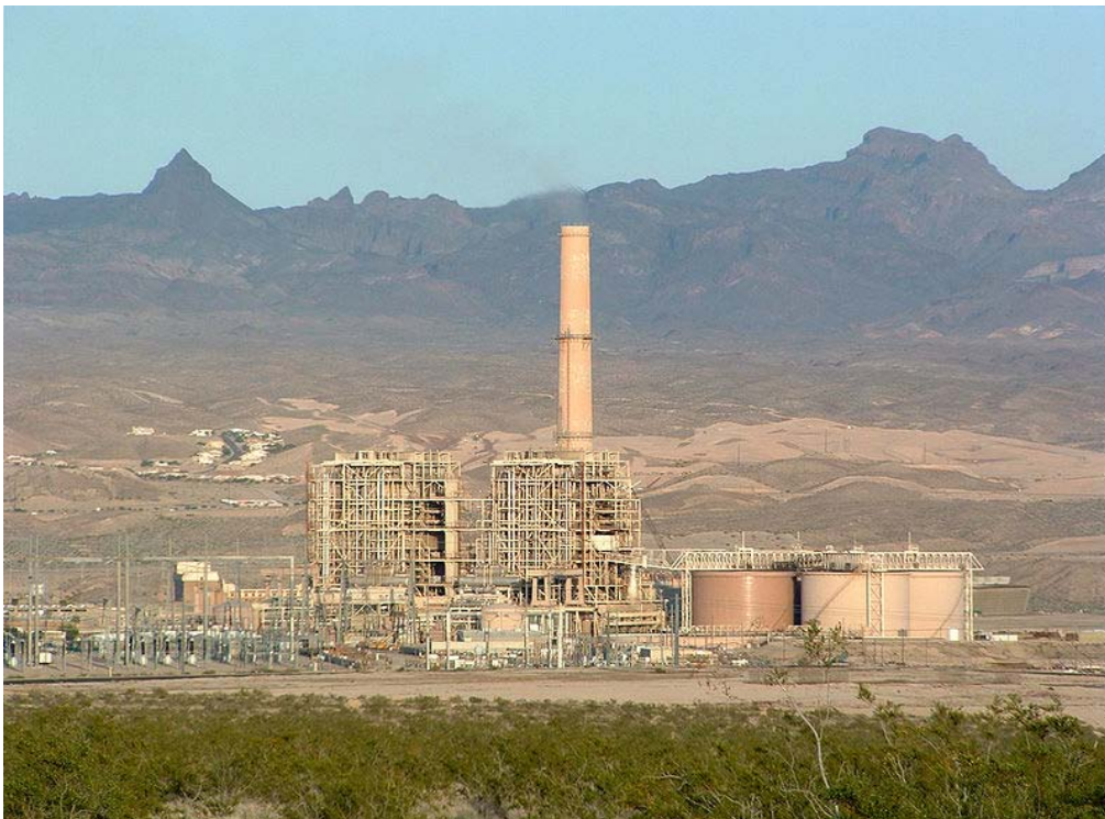
The Mohave Power Station, a 1,580 MW coal power station near Laughlin, Nevada, out of service since 2005 due to environmental restrictions
