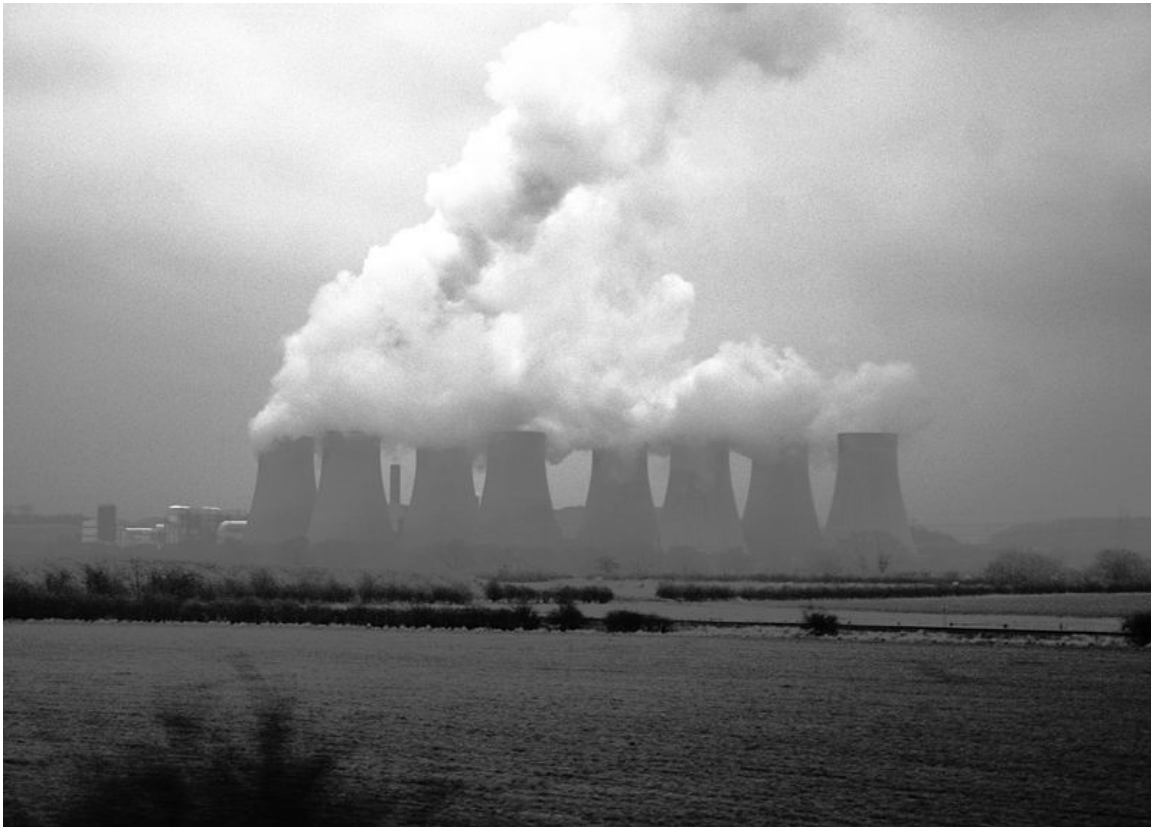
Cooling towers evaporating water at Ratcliffe-on-Soar Power Station, United Kingdom.
