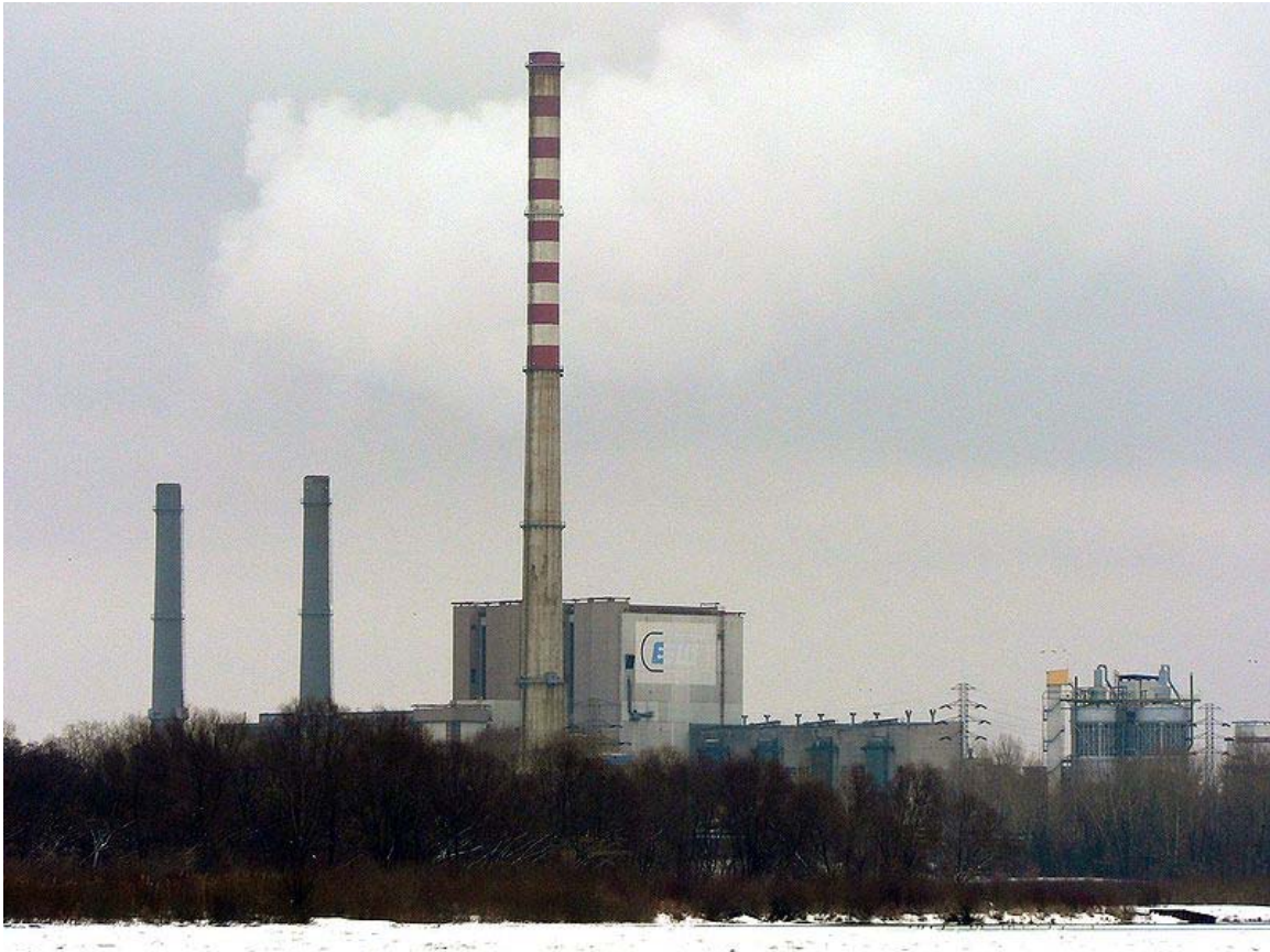
CHP plant in Warsaw, Poland.
