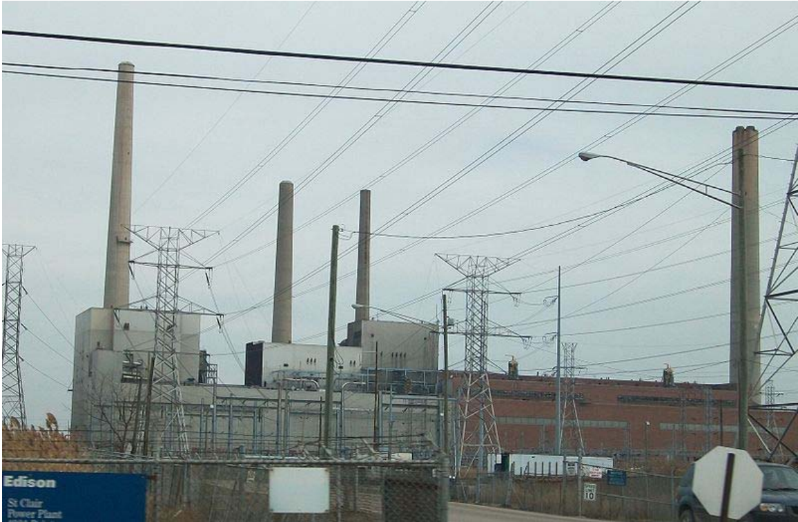
The St. Clair Power Plant, a large coal fired generating station in Michigan.
