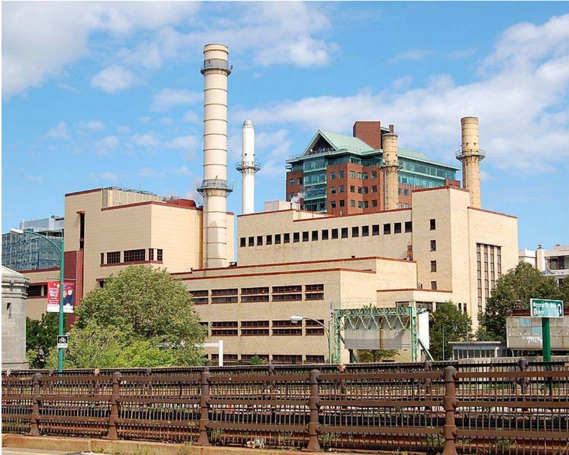
A 250 MW cogeneration plant in Cambridge, Massachusetts
