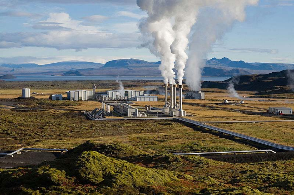
Geothermal power station in Iceland.
