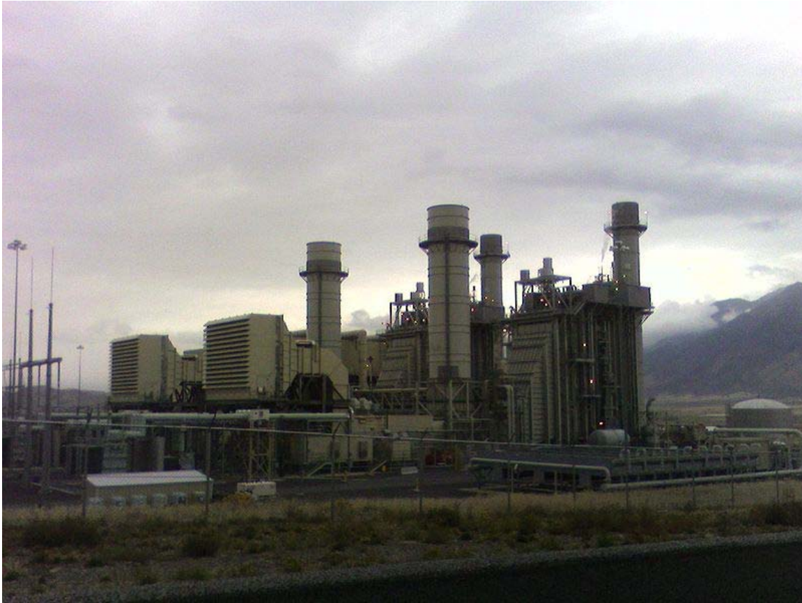
Curren Creek Power Plant near Mona, Utah is a natural gas fired electrical plant.
