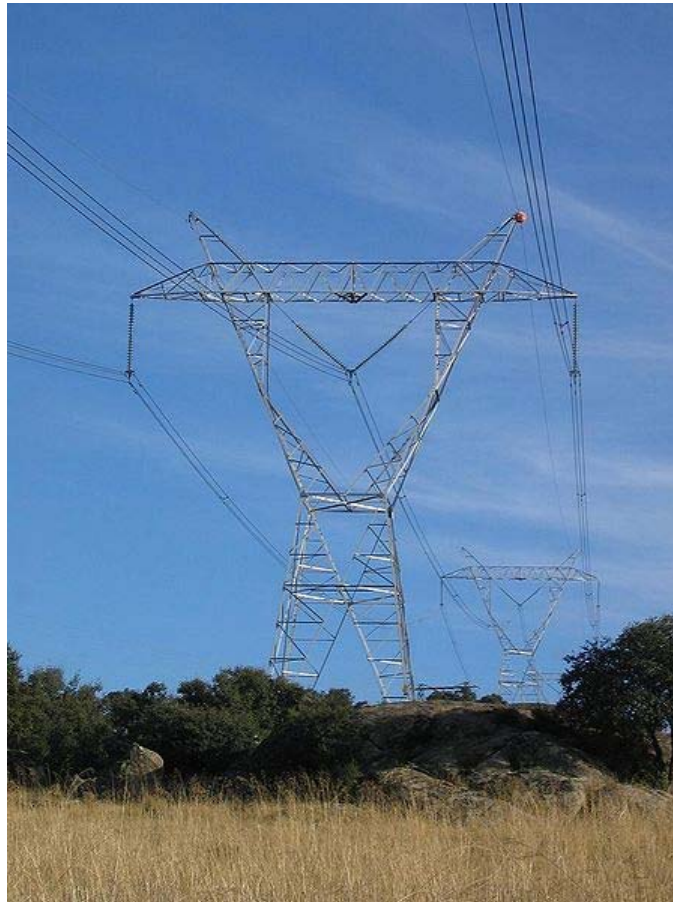
400 kV high-tension transmission lines near Madrid
