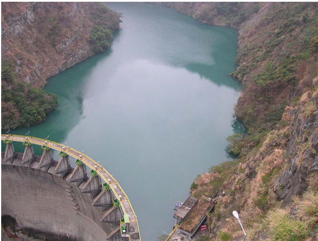
The Zhonghua Dam on the Dahan River in Taoyuan County, Taiwan.
