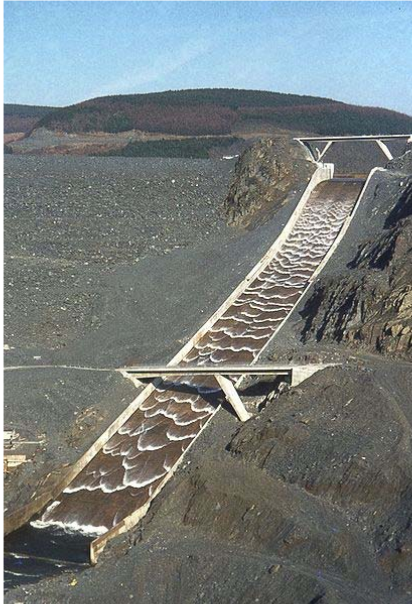
Figure 5: Series of roll waves moving down a spillway, where they terminate in a stationary hydraulic jump.
