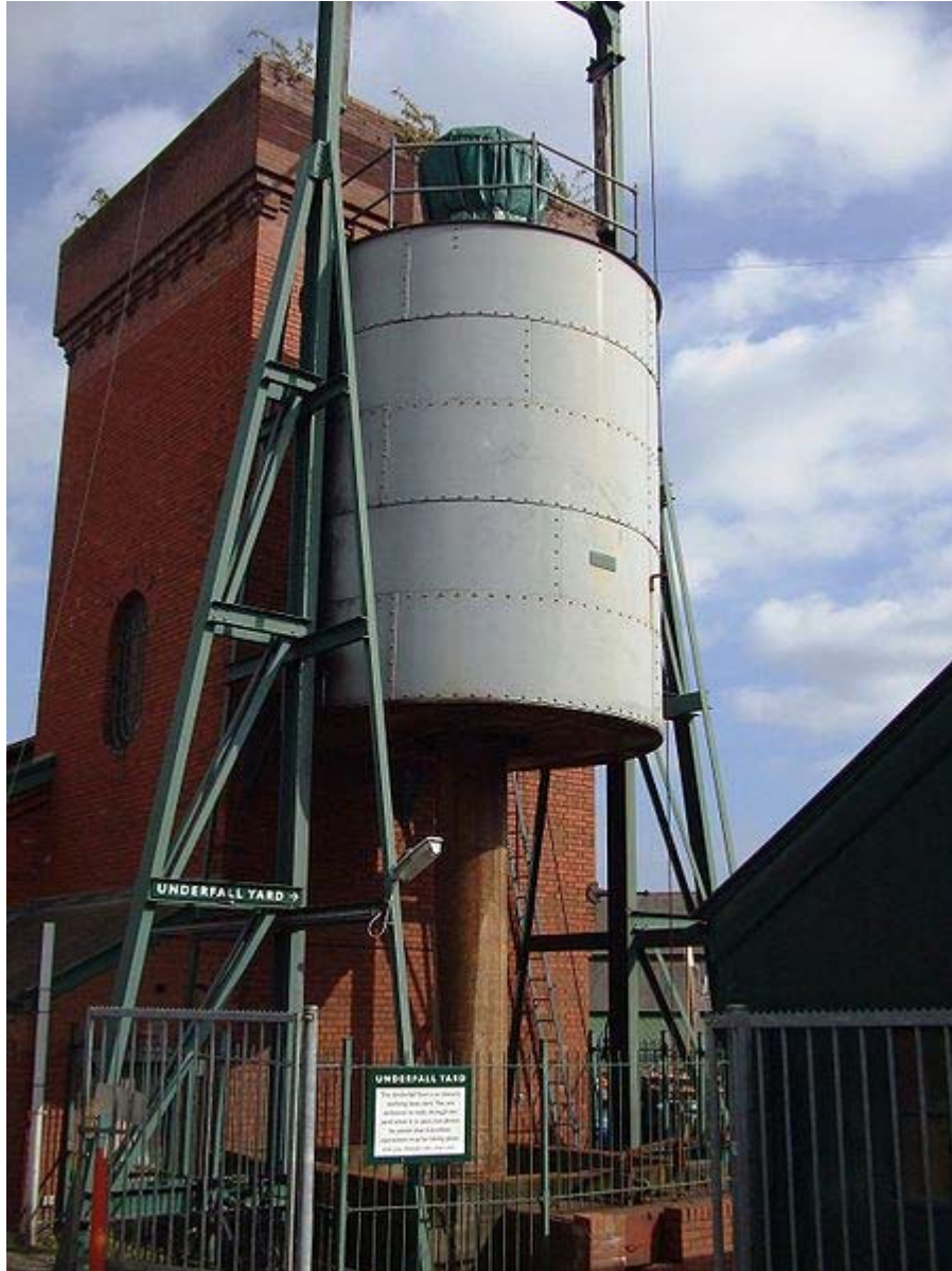
Hydraulic engine house, Bristol Harbour
