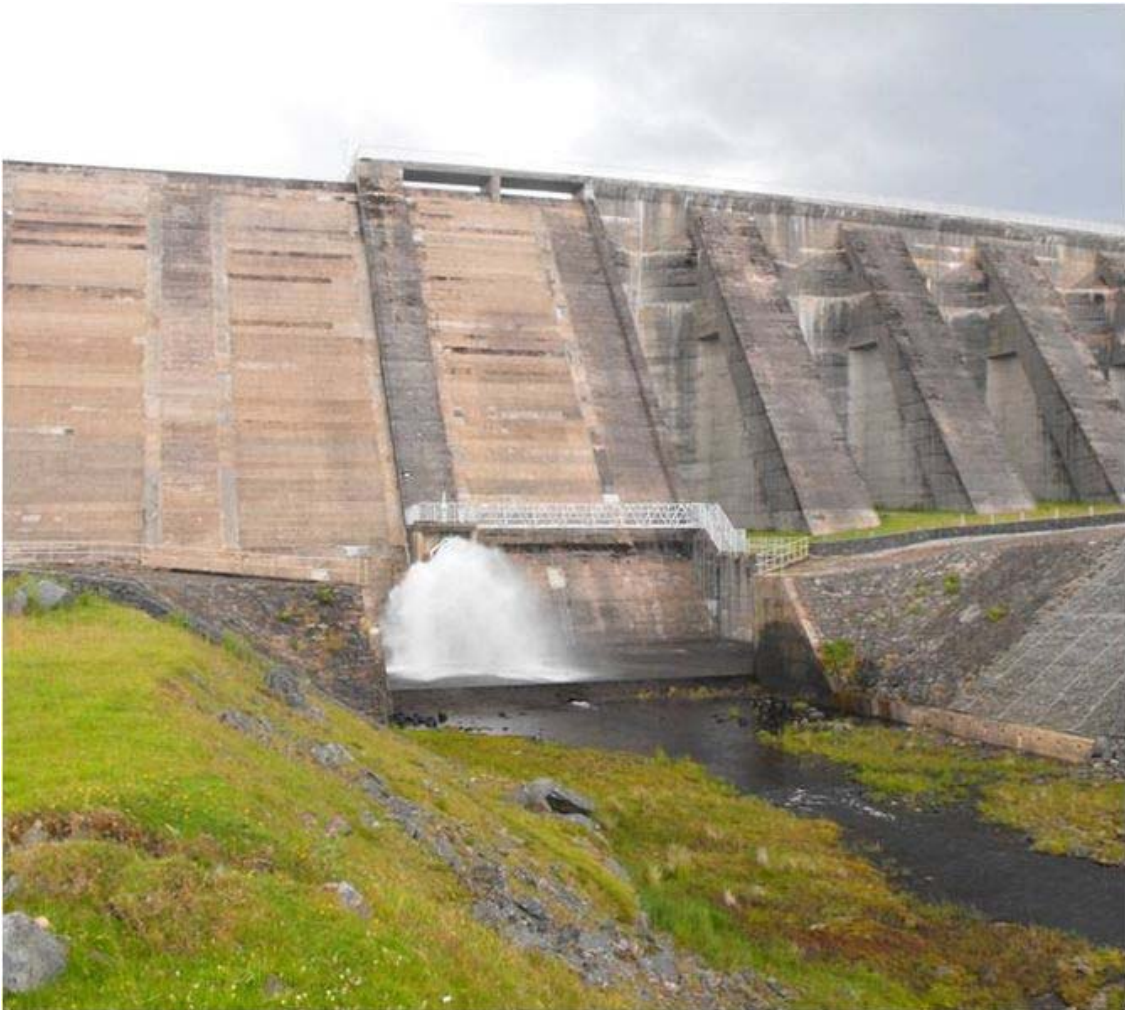
Hydraulic Flood Retention Basin (HFRB)
