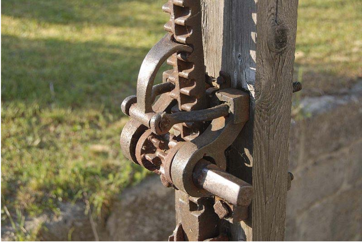
200-year-old paddle gear on the Wiener Neustädter Kanal, Austria
