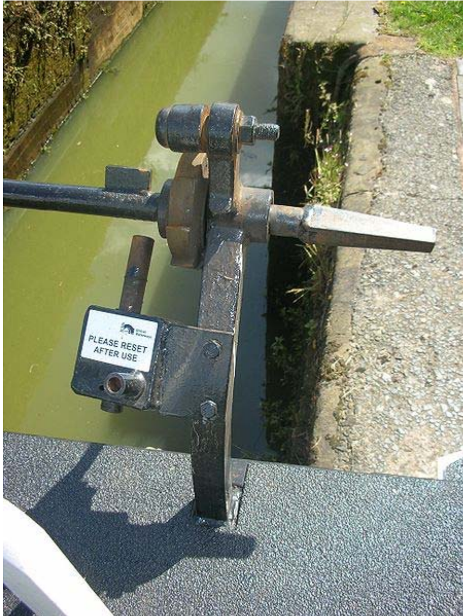
Water conservation gear on the Birmingham Canal Navigations
