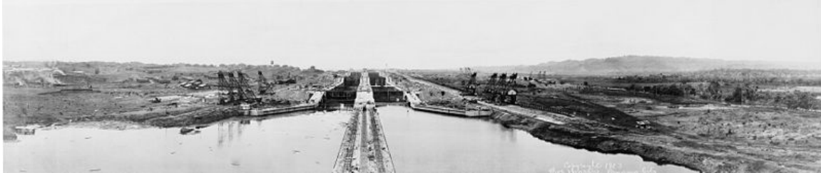
Locks of the Panama Canal during construction, 1913.
