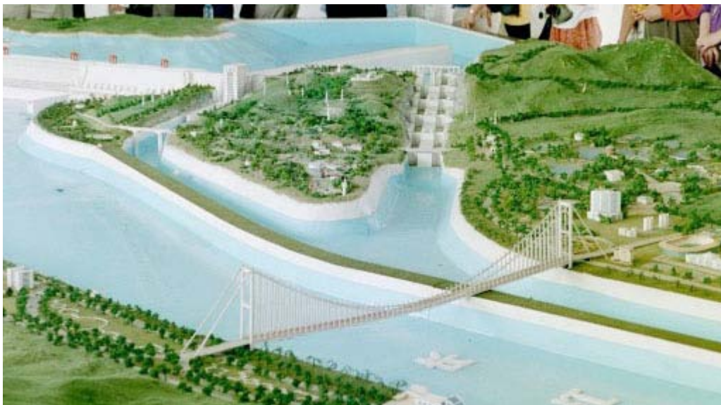
Three Gorges Dam model view. A pair of five locking steps is at center with a ship lift to the left
