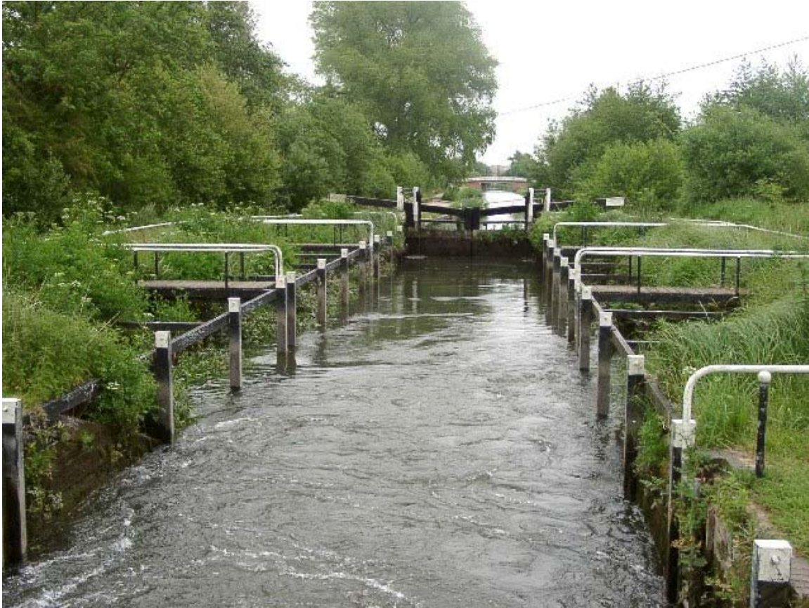
The turf-sided Monkey Marsh Lock on the Kennet & Avon Canal at Thatcham
