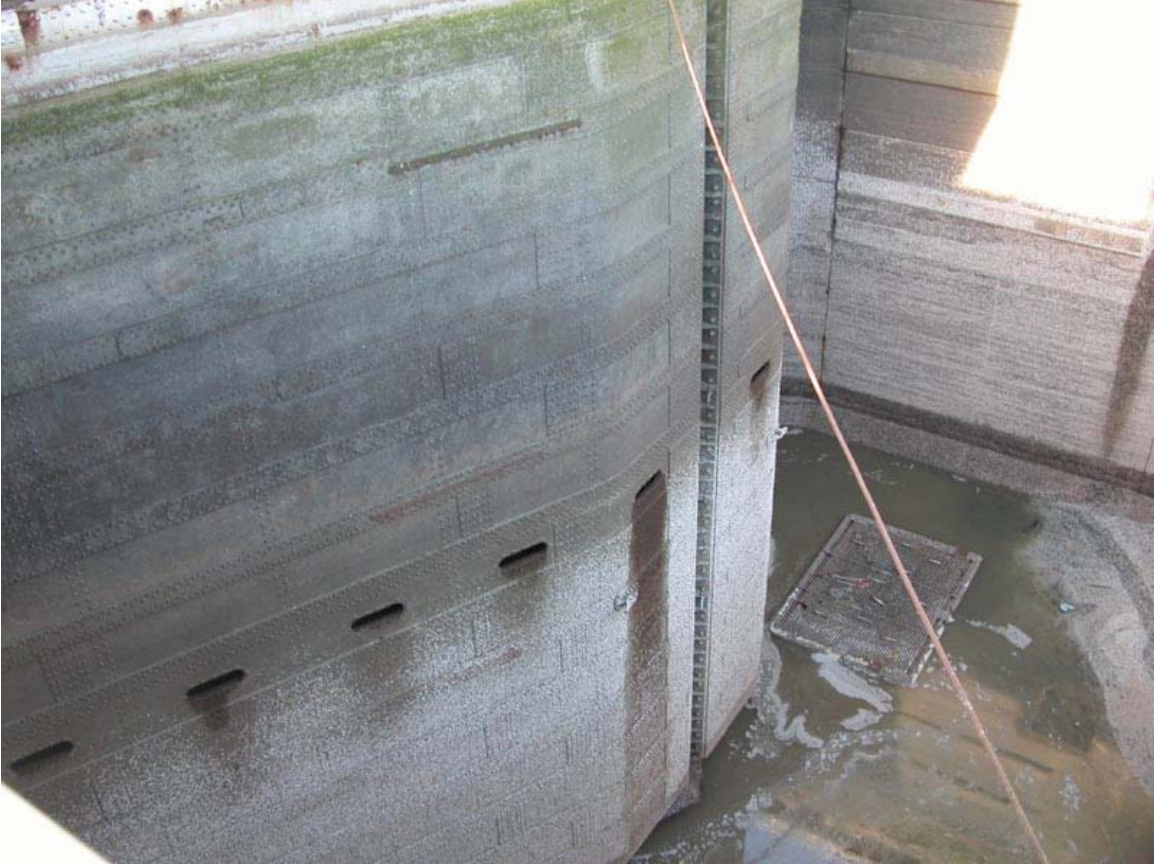
Lock emptied for maintenance – centre pair of gates.
