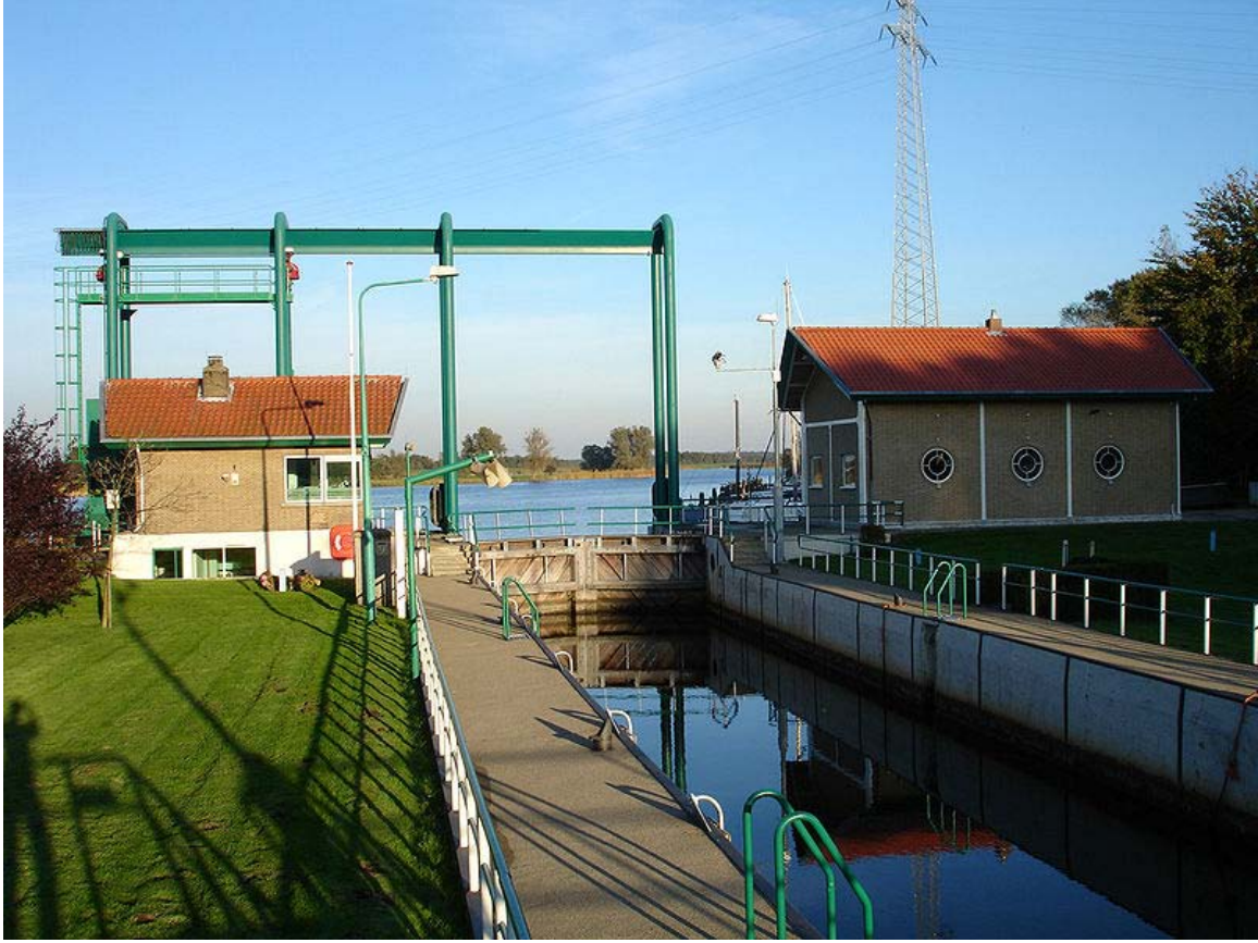
Canal lock in the Noordoostpolder, Netherlands.
