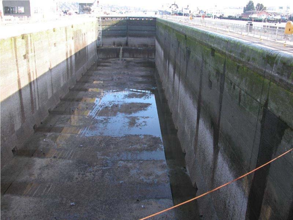
Lock emptied for maintenance – high water end of the lock.
