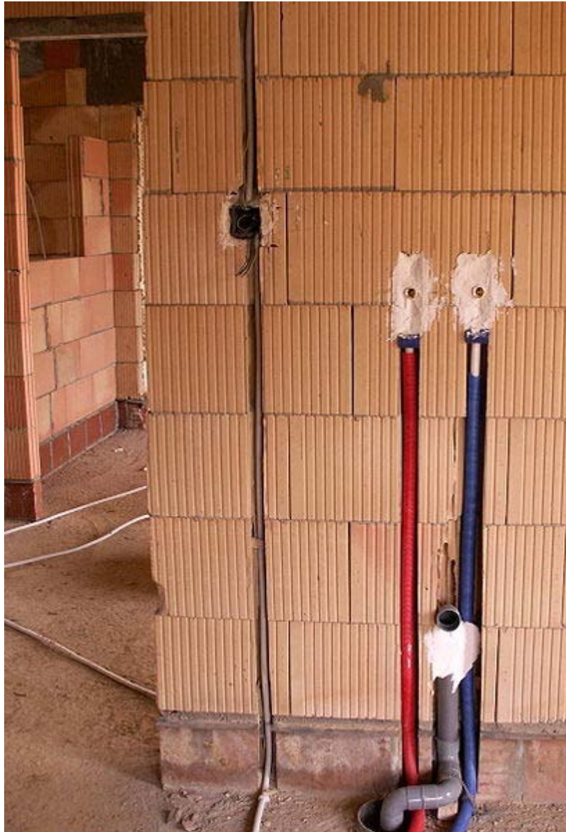
Piping being placed for a sink
