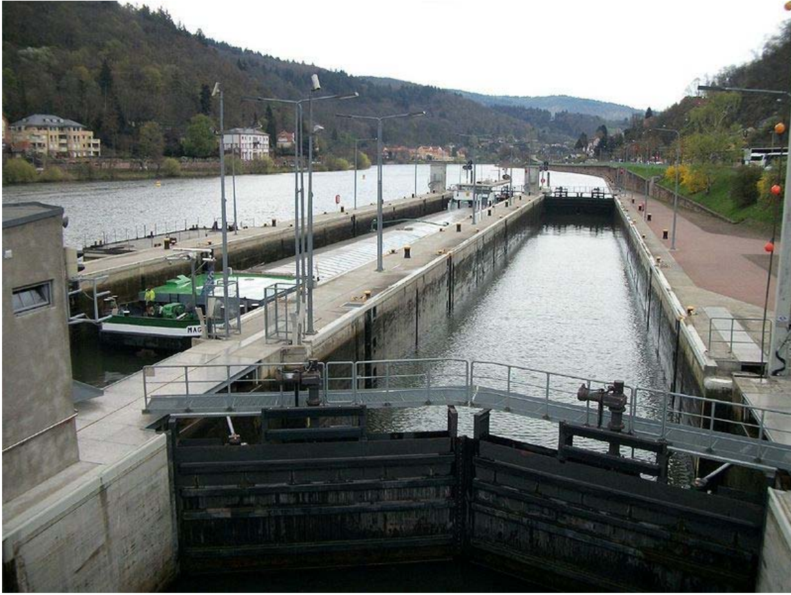
Lock in river Neckar, Heidelberg, Germany
