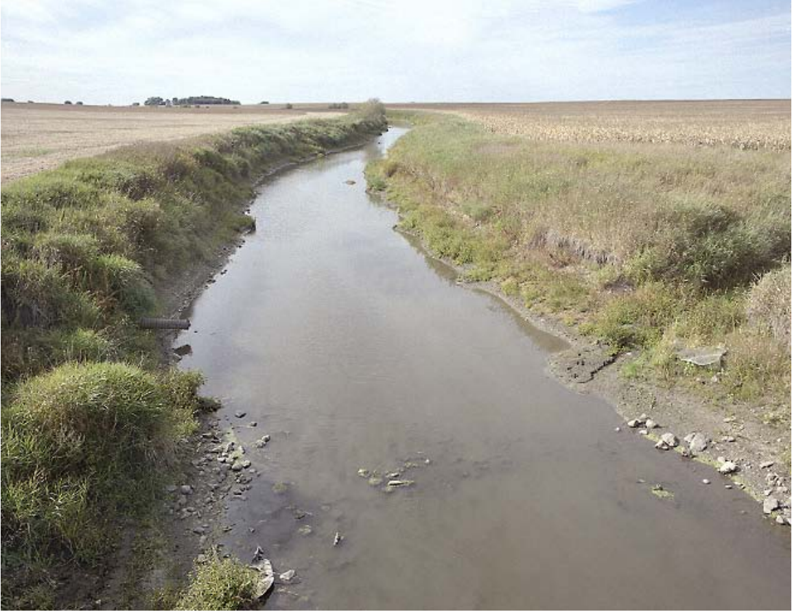
A channelized section of the South Fork of the Crow River in Meeker County, Minnesota
