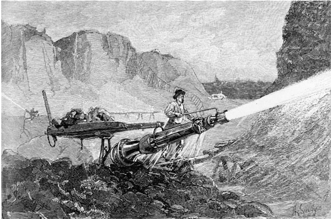
Hydraulic mining for gold in California, from The Century Magazine January 1883
