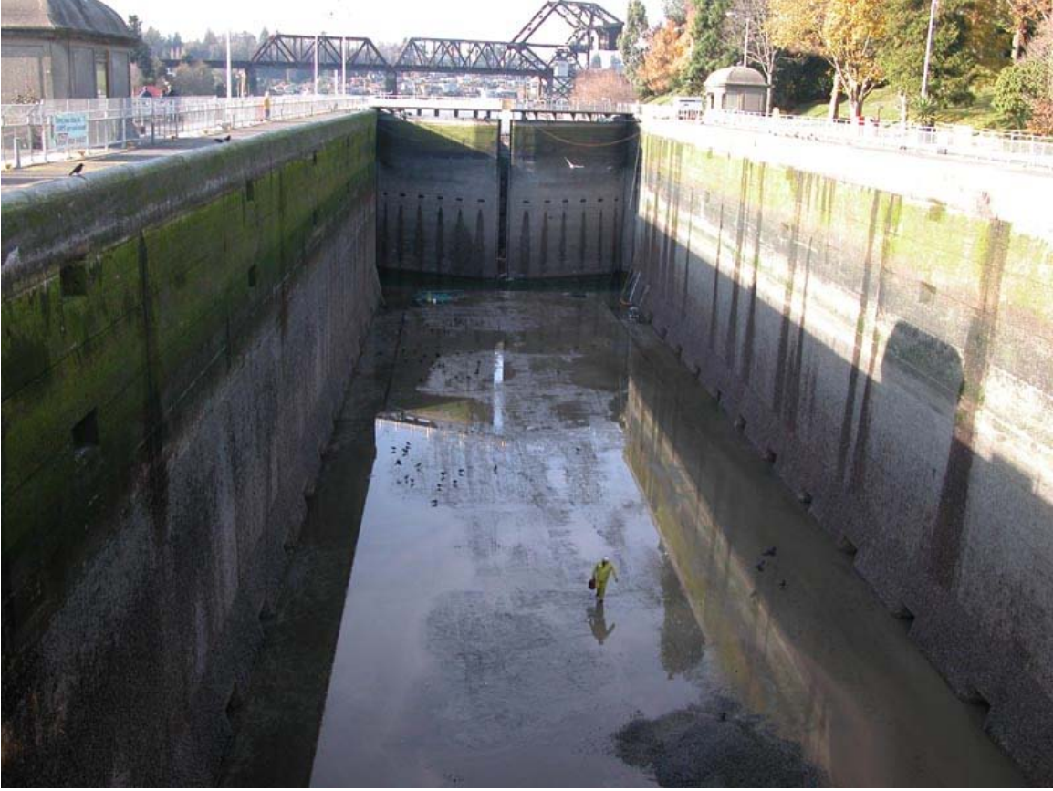
Lock emptied for maintenance – low water end of the lock.
