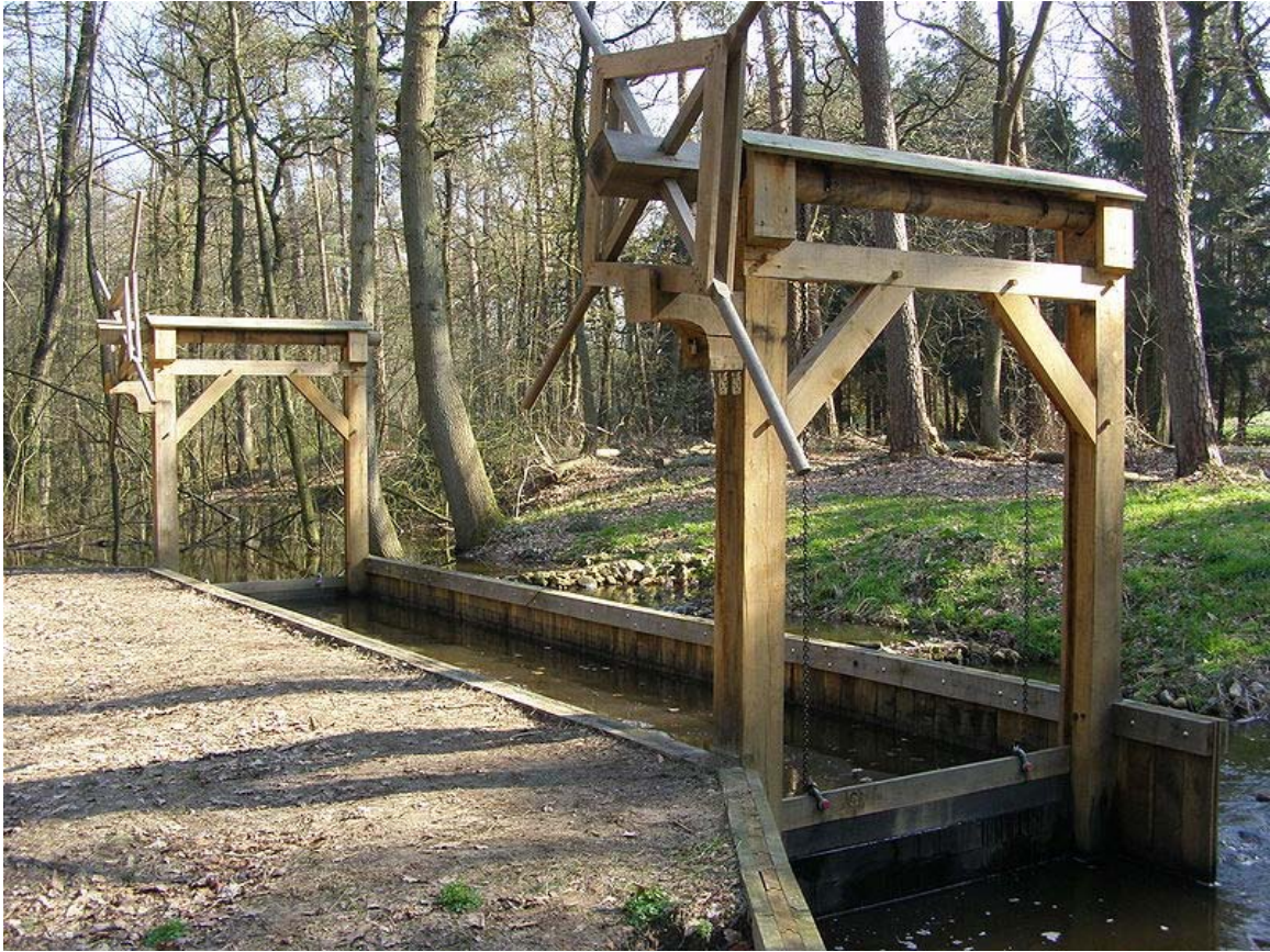
Model of early river pound lock, constructed in Lankheet water park, Netherlands
