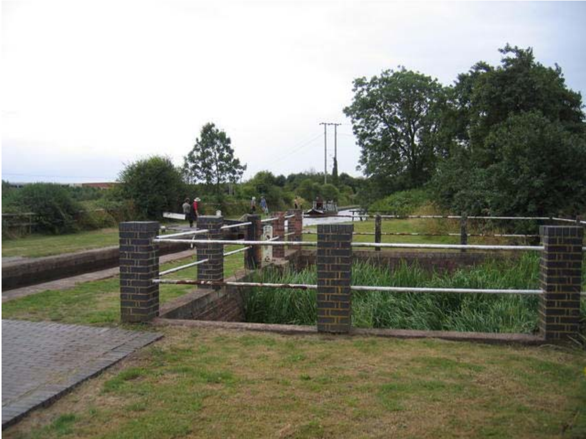
Disused side pond at Atherstone on the Coventry Canal, England
