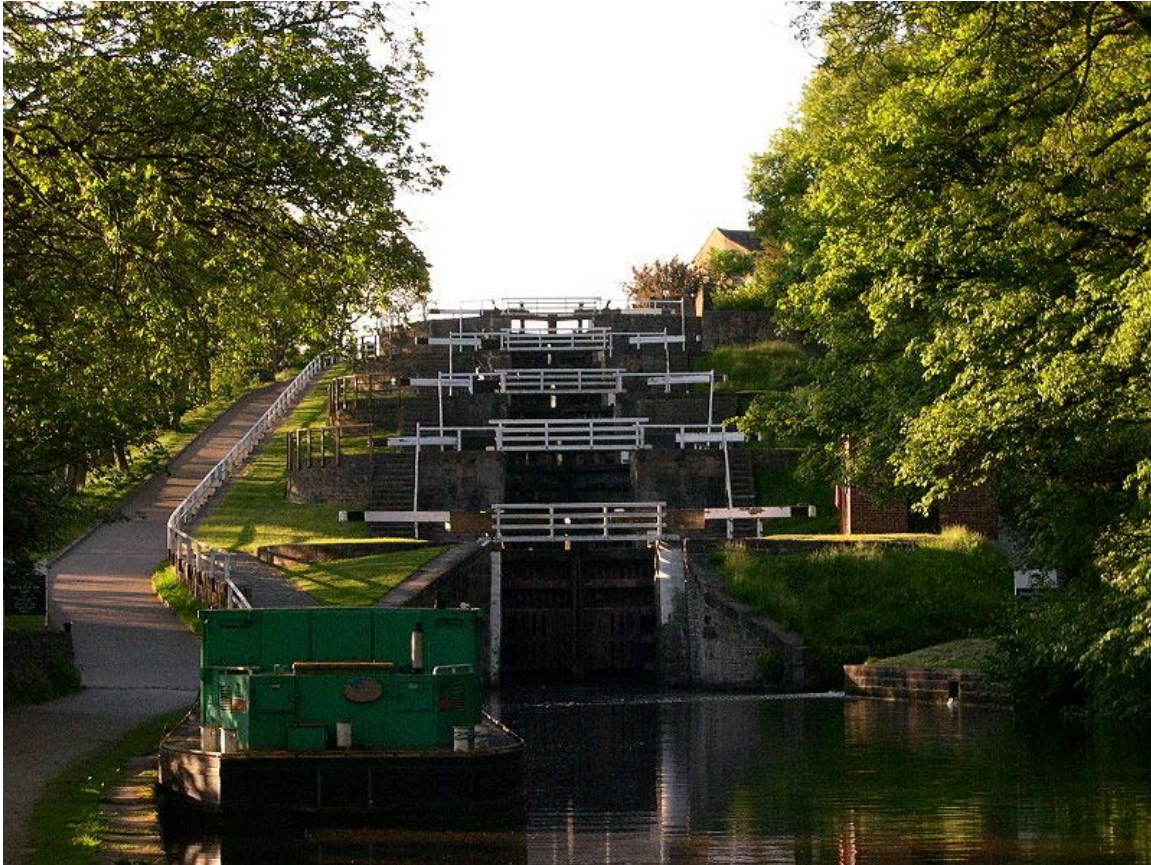
Staircase of five locks, dating from 1774, at Bingley, England
