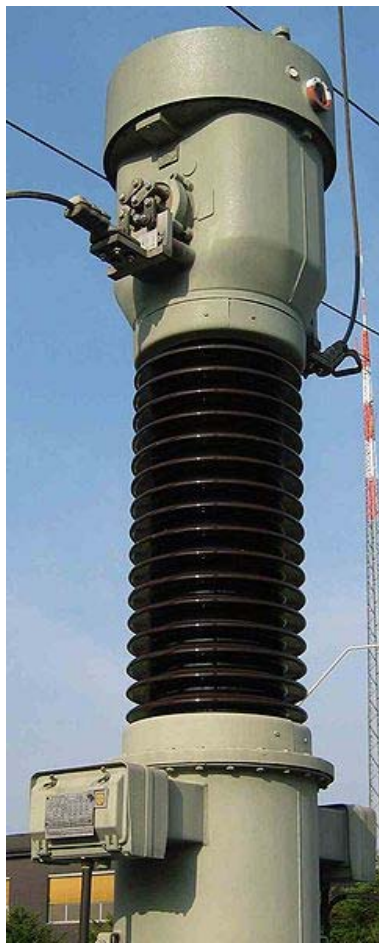
A CT for operation on a 110 kV grid
