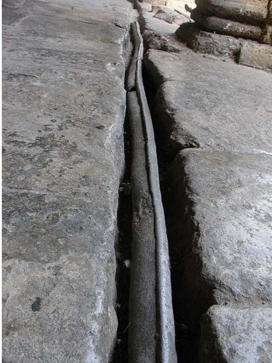
Lead pipe in Roman baths
