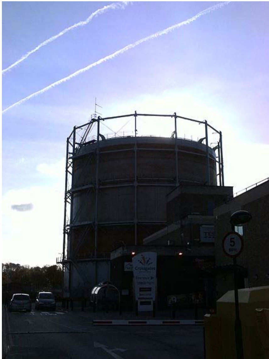
Column guided gas holder at Cross Gates, Leeds This is the first of a former twin holder station constructed around 1900
