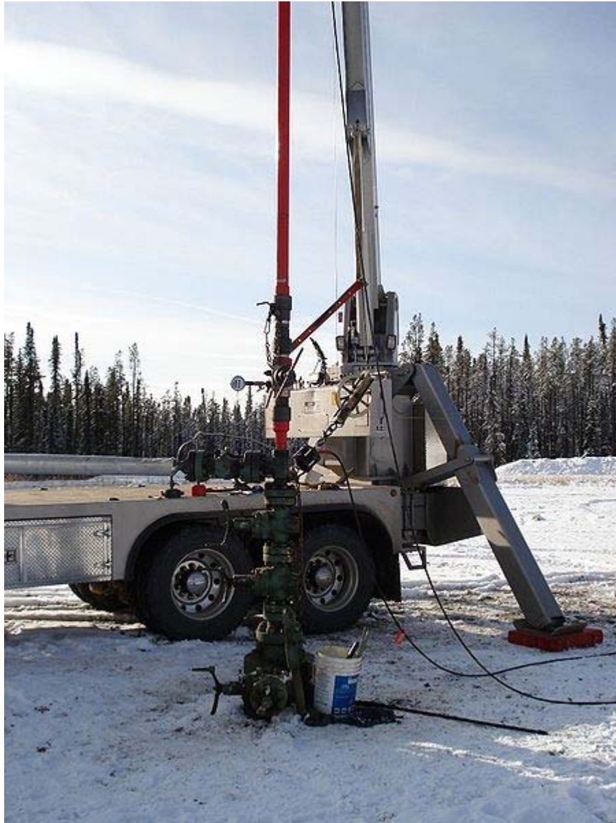
Wireline attached to top of Christmas Tree
