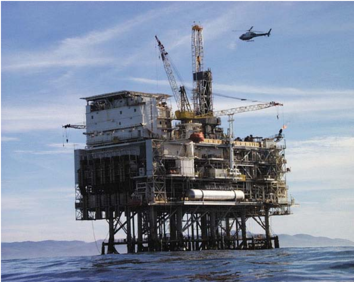
A typical offshore Oil/Gas platform.
