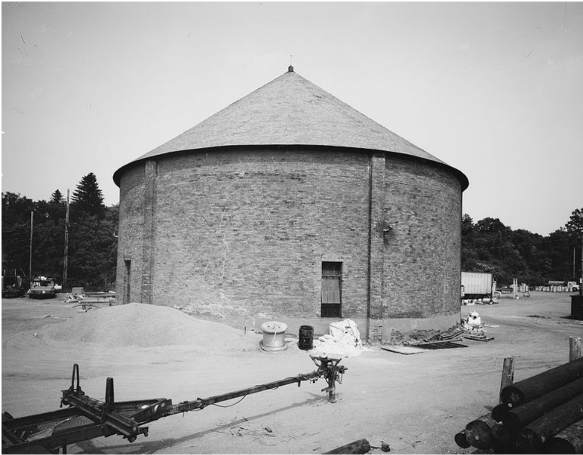
Rare extant 19th century gasholder house in Saratoga Springs, NY.
