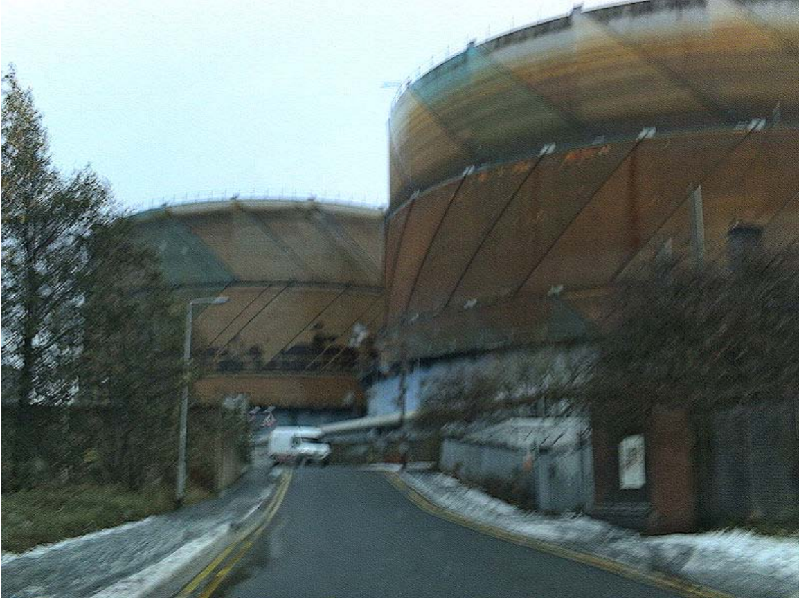
Spiral guided gasholders at the former Meadow Lane Gas Works in Hunslet, Leeds. These were constructed around 1965
