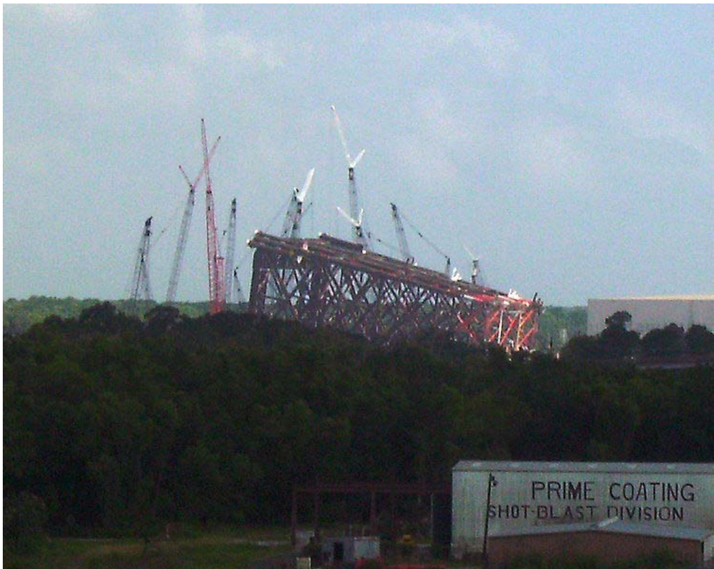
A fixed platform base under construction on a Louisiana river
