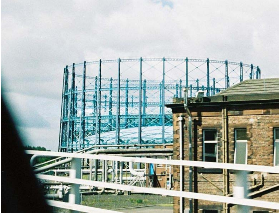
Large gas holders imposing on the skyline in Glasgow, pipework and the booster house can also be seen.
