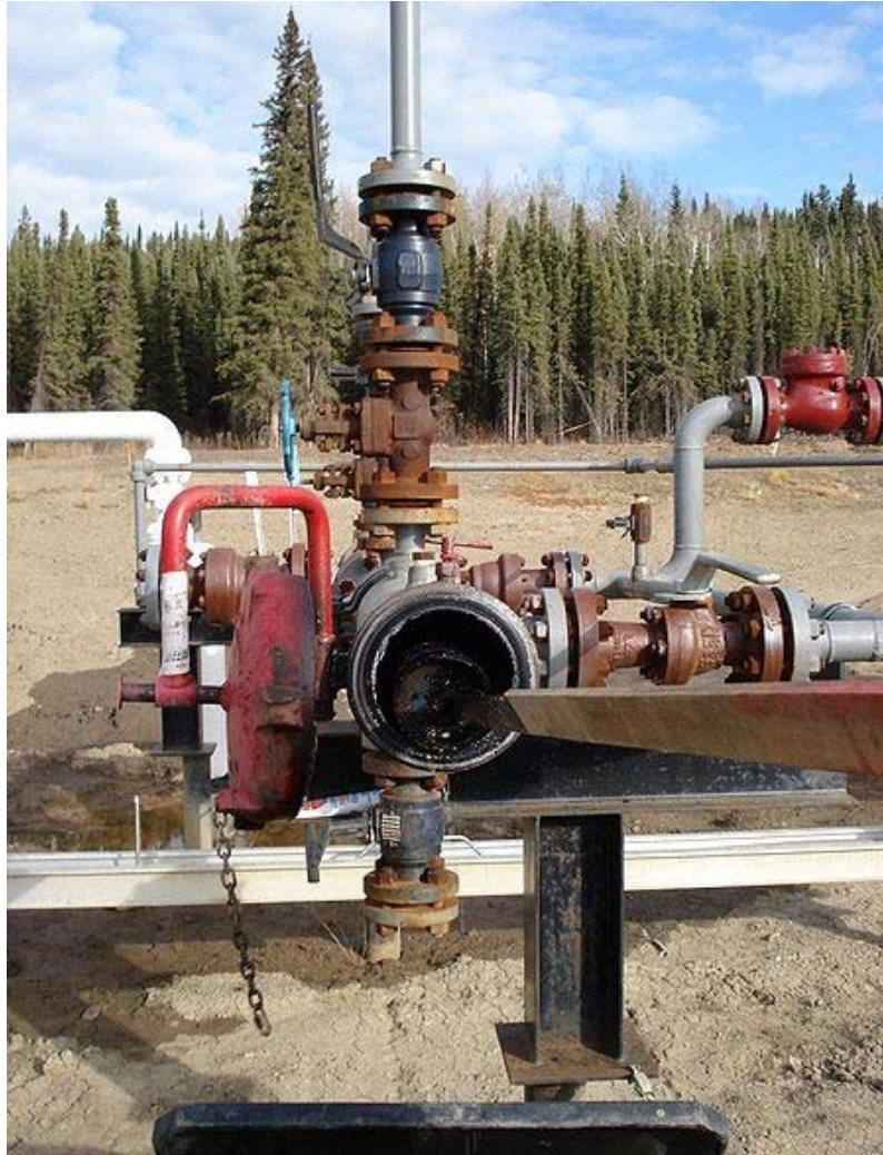
Inserting a pig into a natural gas pipeline
