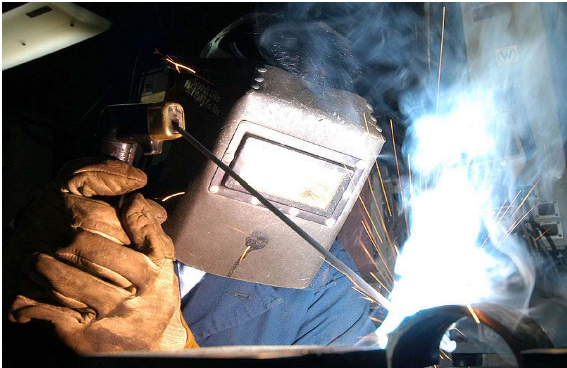
Shielded metal arc welding
