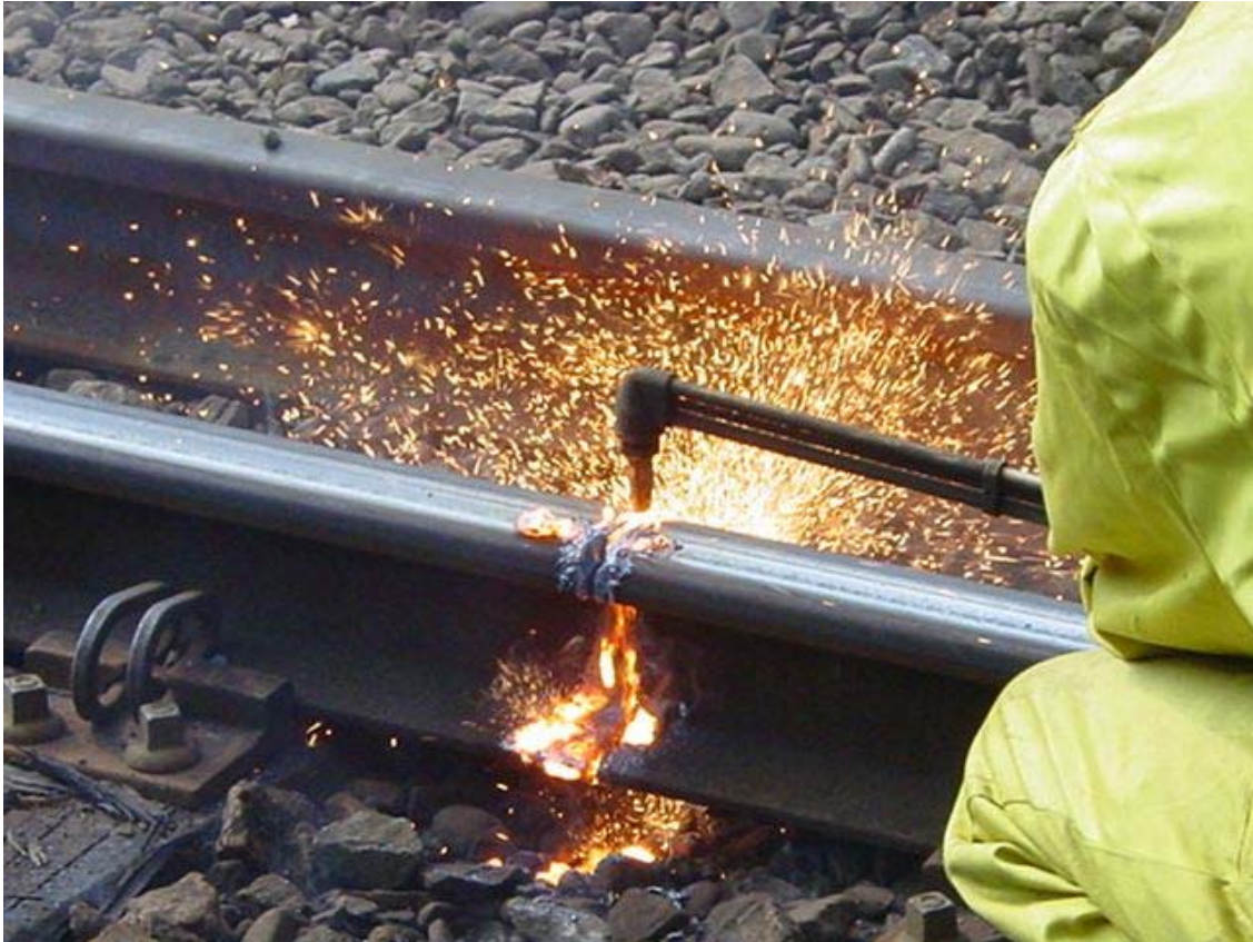
Cutting a rail just before renewing the rails and the ballast.
