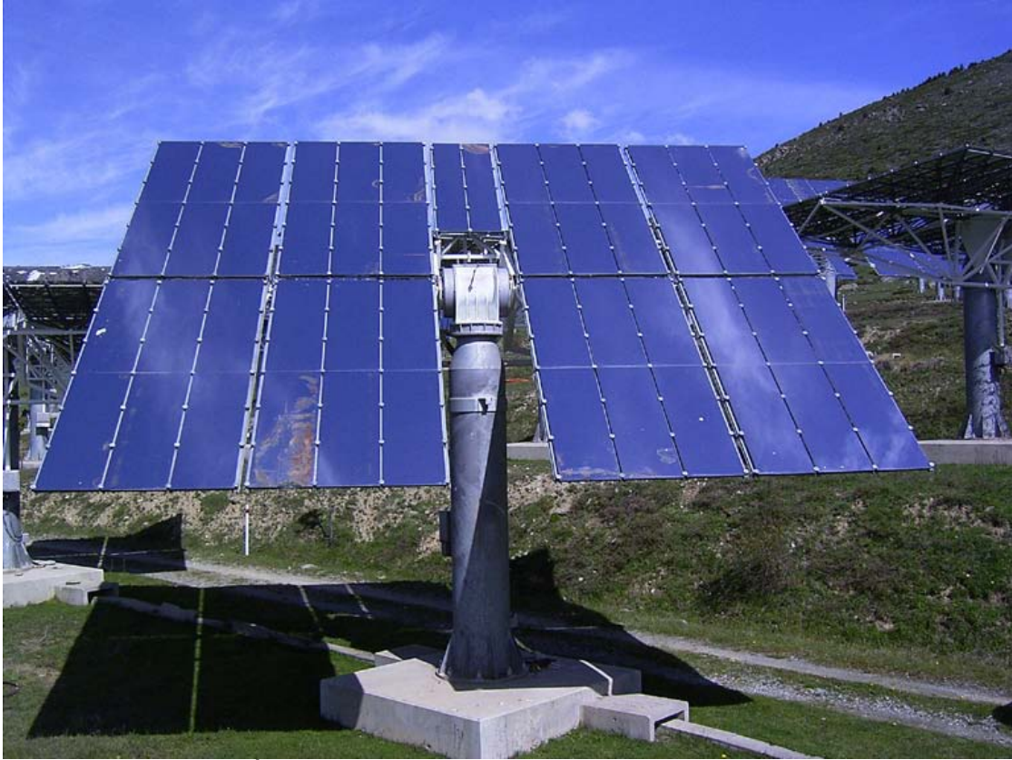
A heliostat at the THEMIS experimental station in France. The mirror rotates on an altazimuth mount.
