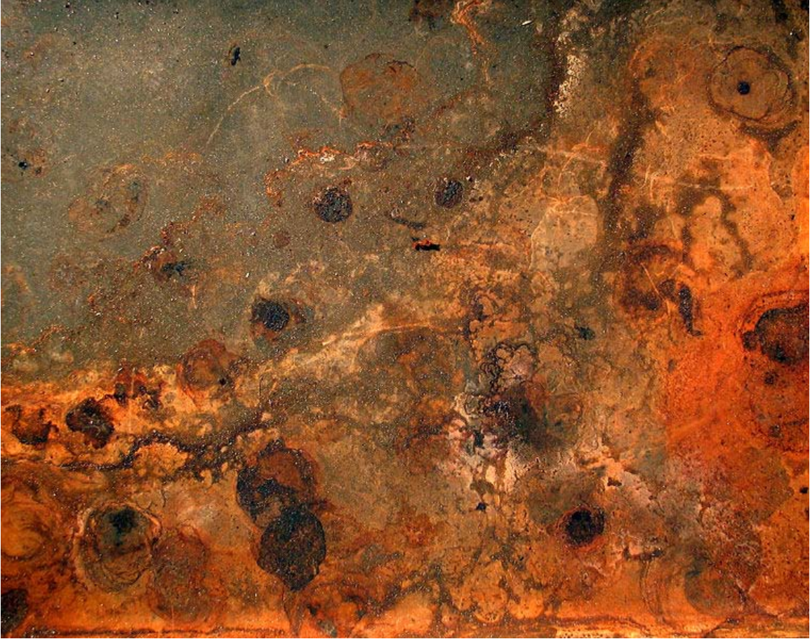
Rust, the most familiar example of corrosion.
