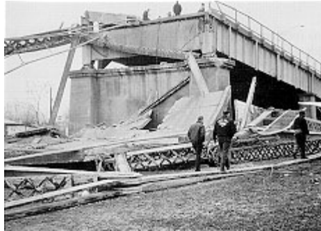
The collapsed Silver Bridge, as seen from the Ohio side
