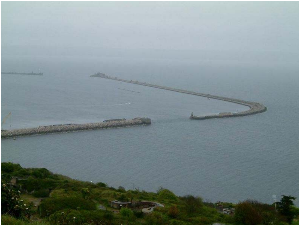
3 of the 4 breakwaters forming Portland Harbour
