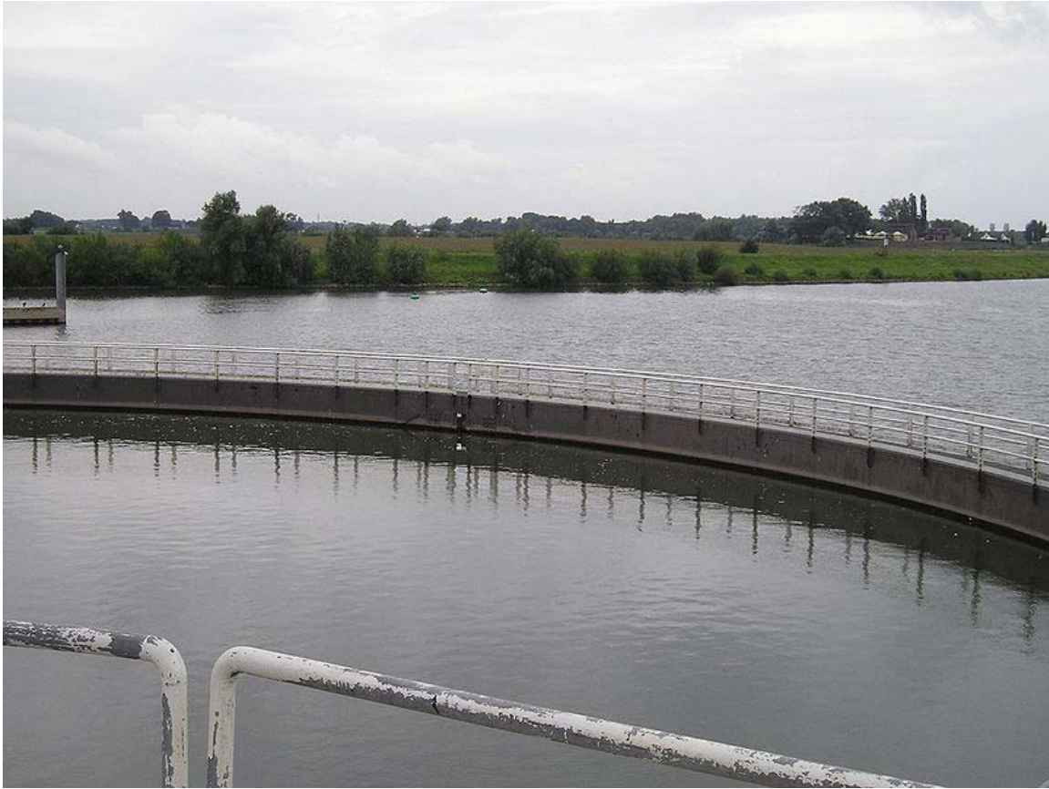
Floodgate Amerongen, The Netherlands
