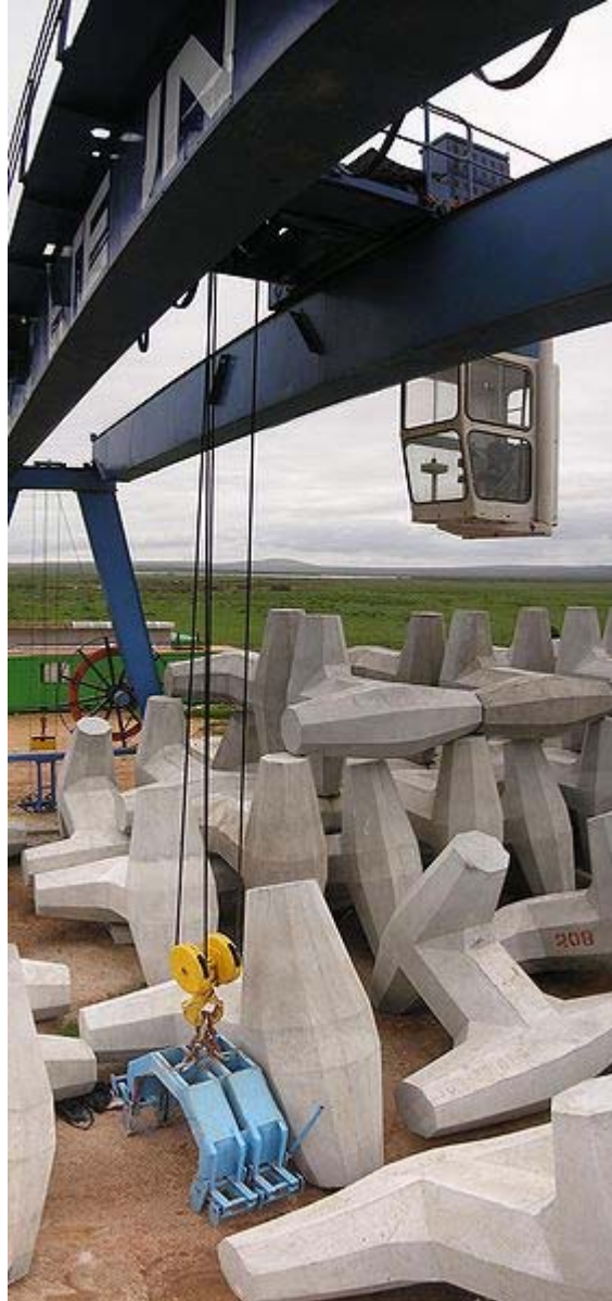
Dolos construction yard - Yzerfontein, South Africa
