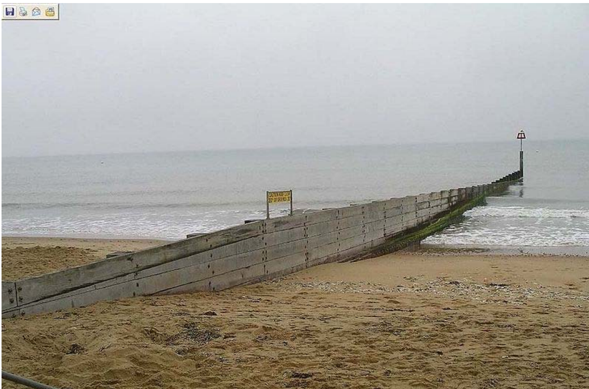
Timber groyne in Sandown, Isle Of Wight, England
