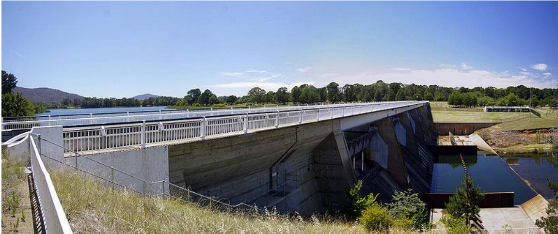
Fish belly flap gates at the Scrivener Dam, Canberra
