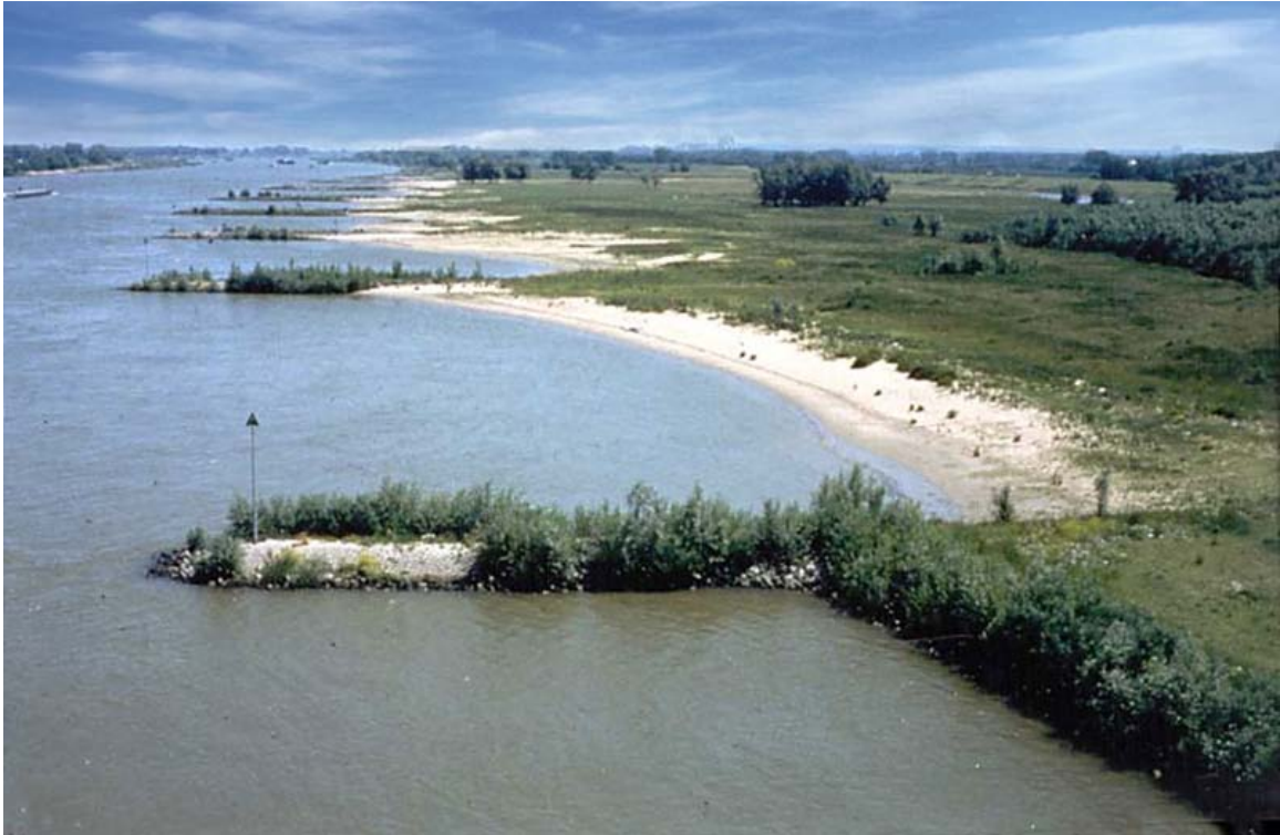
Groynes in the Waal river, part of the Rhine in the Netherlands
