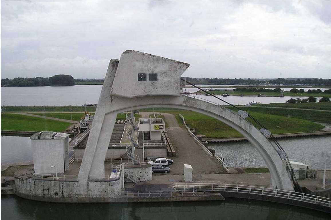
Floodgate Amerongen, The Netherlands
