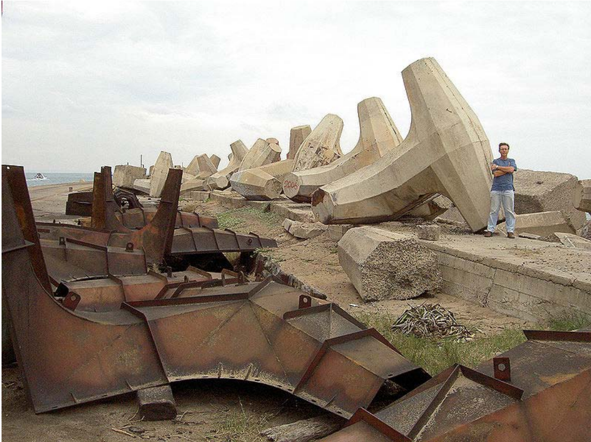
A man stands next to a dolos, showing its relative size. Dolosse moulds are in the foreground - Durban, South Africa
