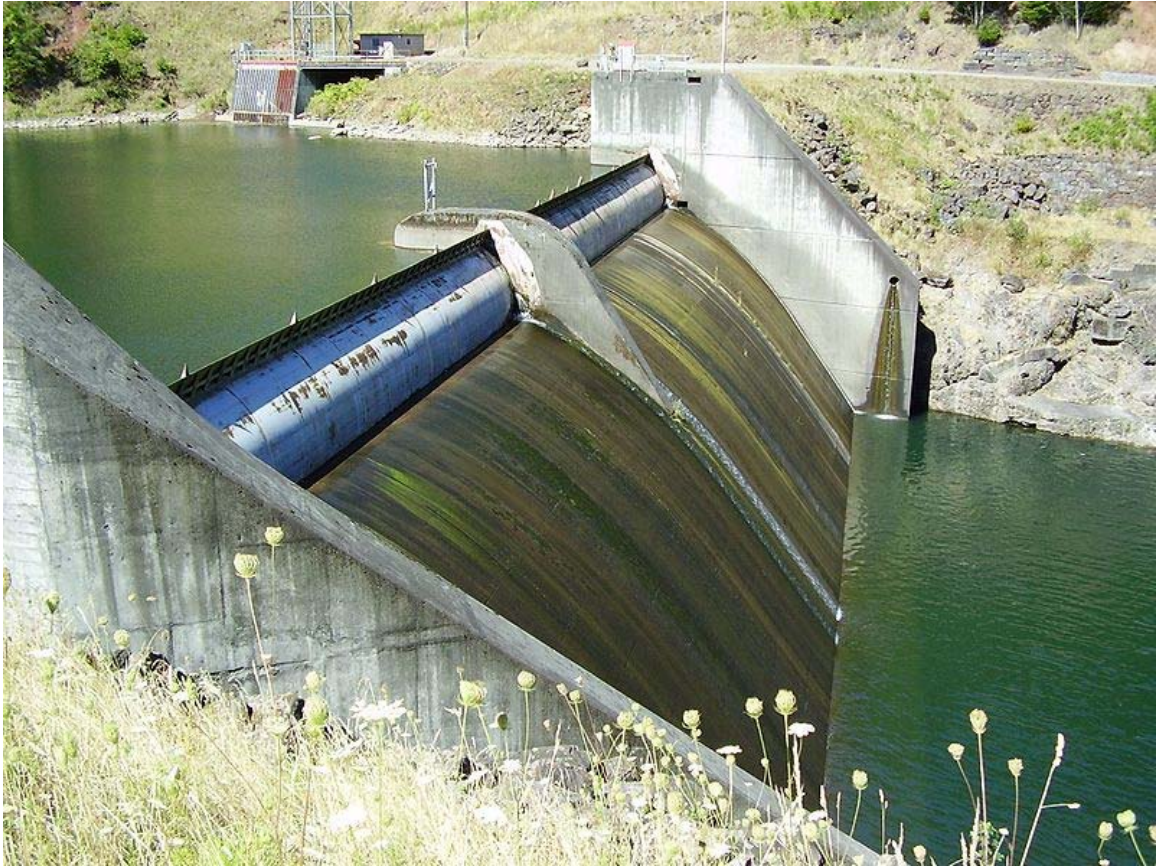
Drum gates on a diversion dam
