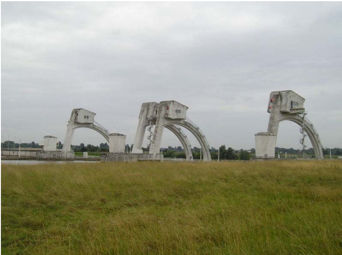
Floodgate Amerongen, The Netherlands
