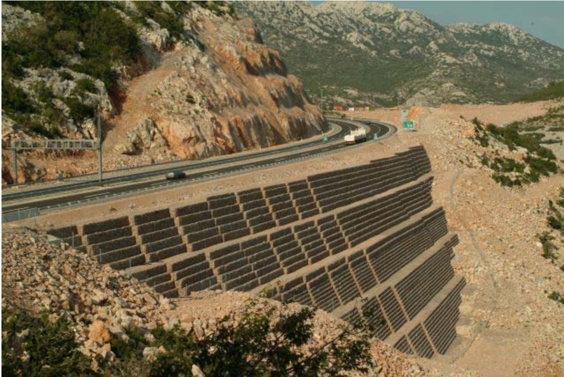
Reinforced earth with gabions, Sveti Rok, Croatia
