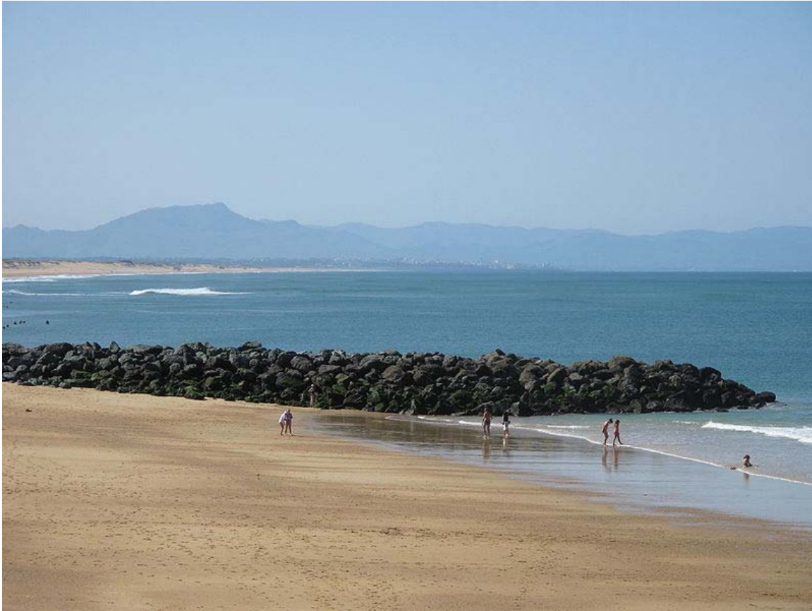
Rocky groyne in Capbreton, France
