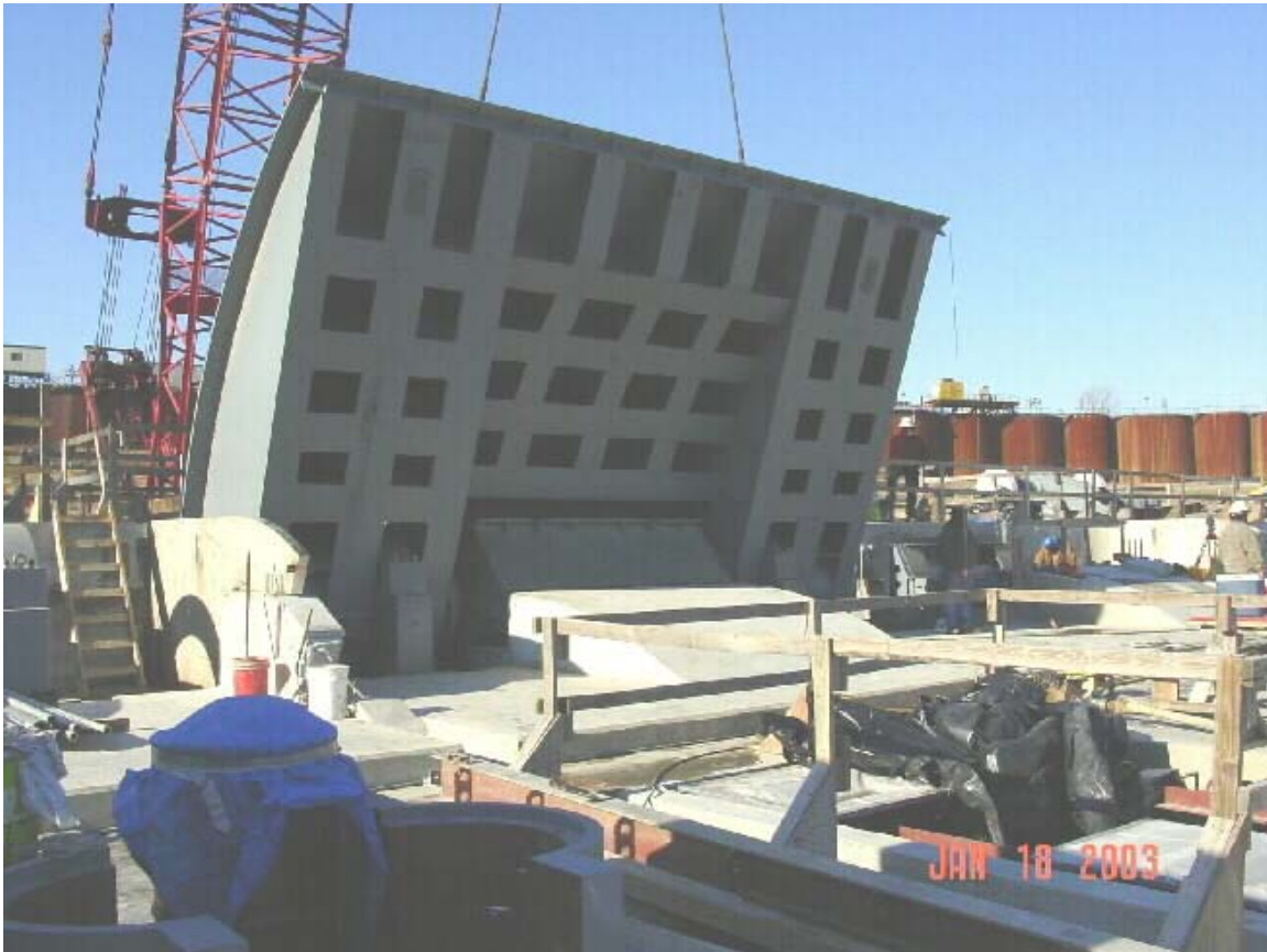
A hinged crest gate during installation
