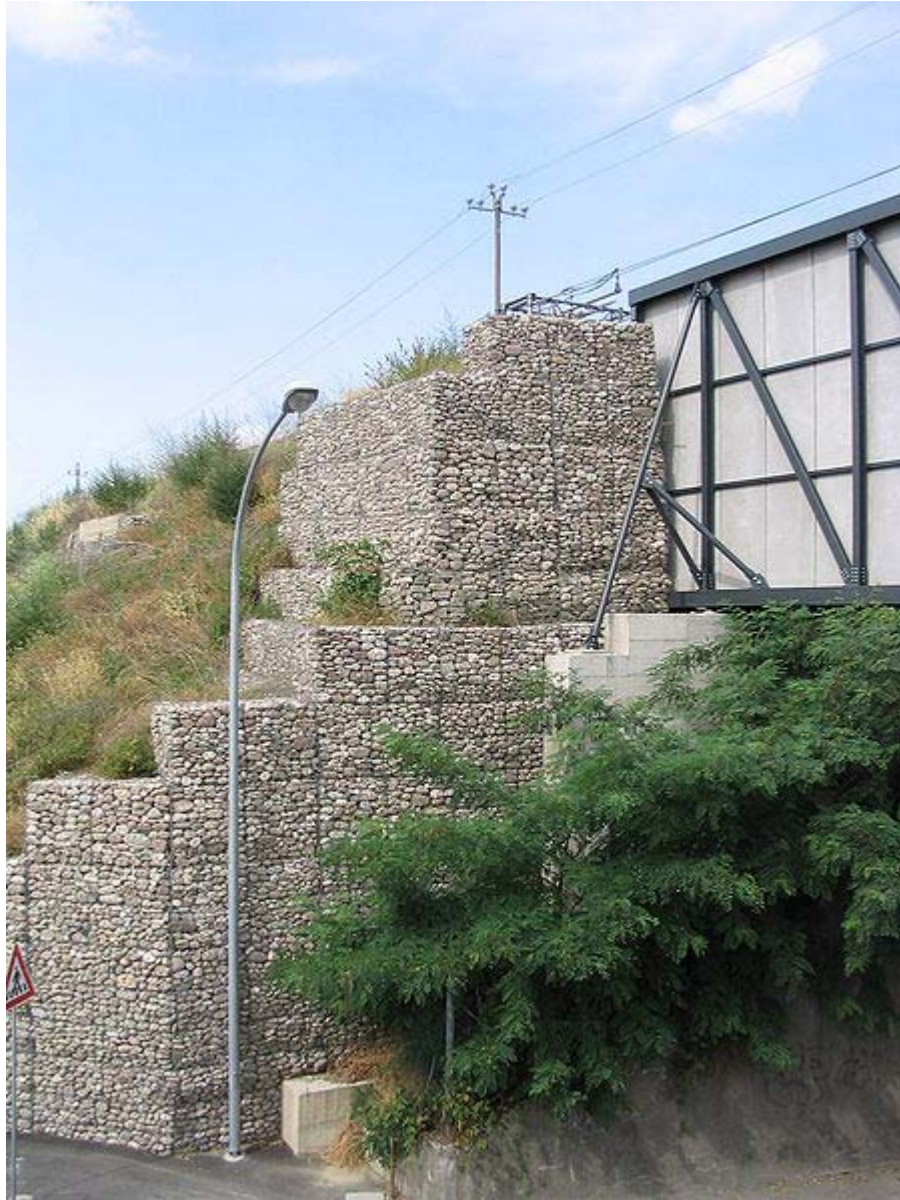
Bridge abutment with gabions
