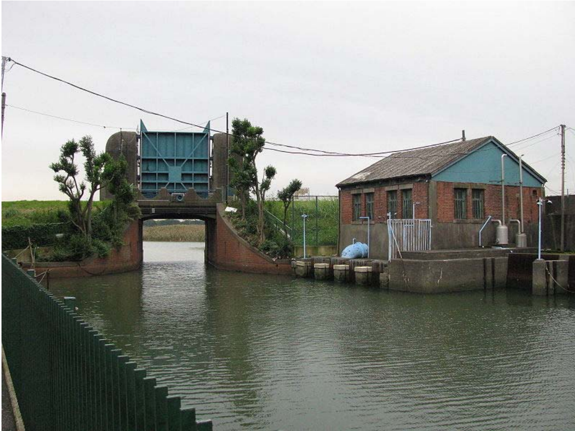
Floodgate in Ota Ward, Tokyo, Japan
