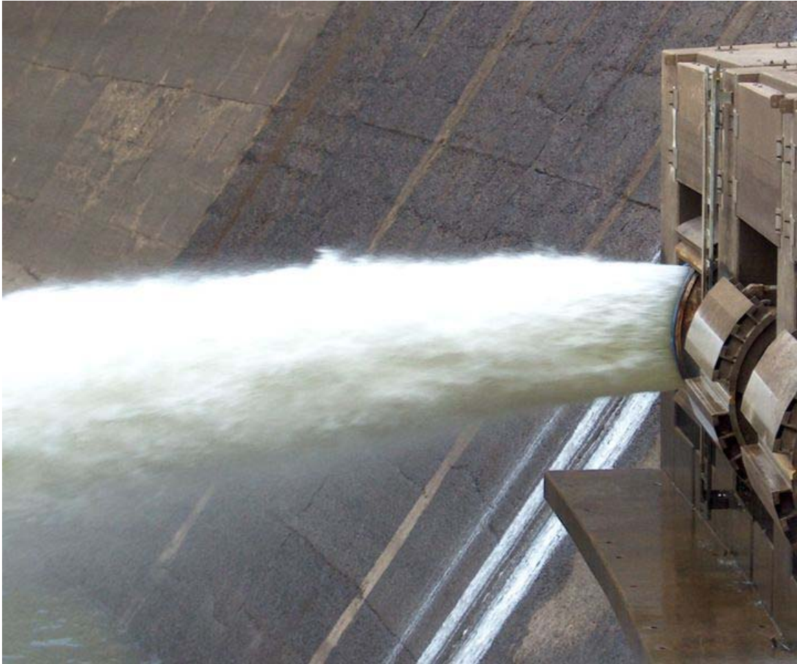
Clamshell floodgates at the Arrowrock Dam
