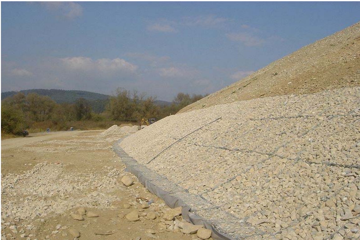
Up close view of a bank protection made with mattresses in Vrtižer, Slovakia
