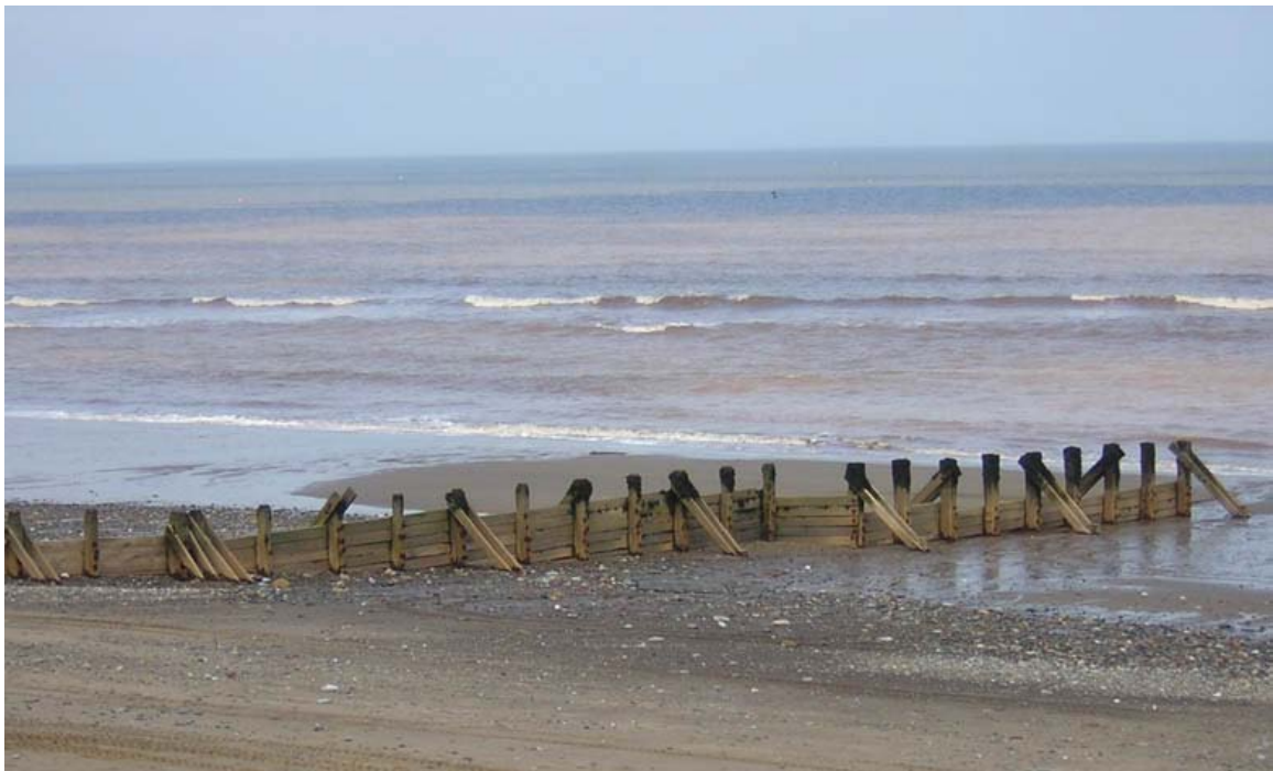
Groyne on the East coast of England
