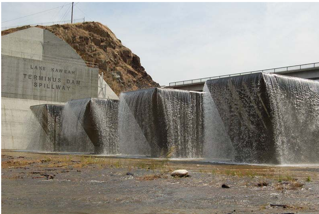
Fusegate in Terminus Dam - Lake Kaweah
