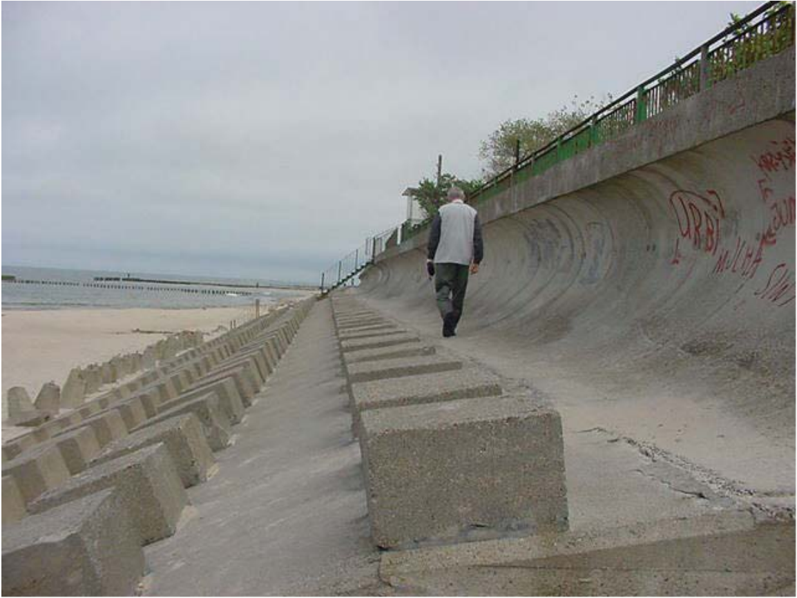
Seawall in Poland
