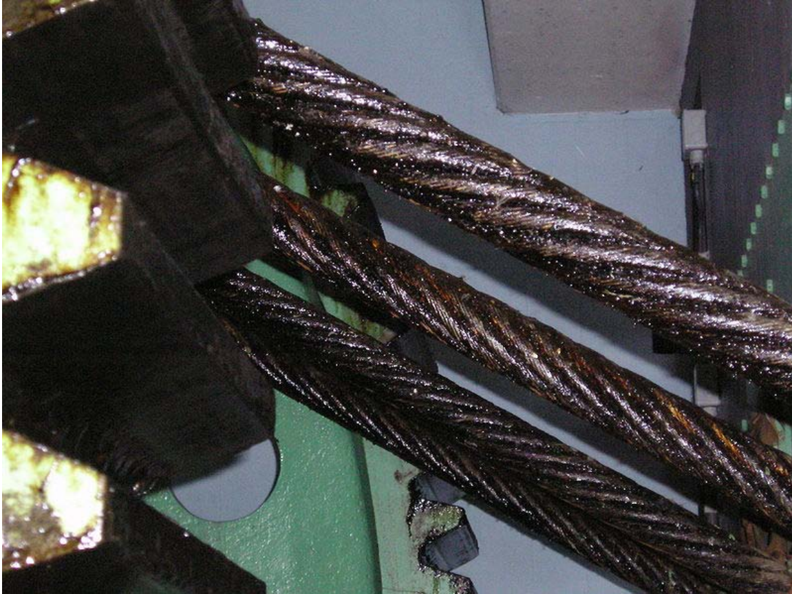
Floodgate Amerongen, The Netherlands
