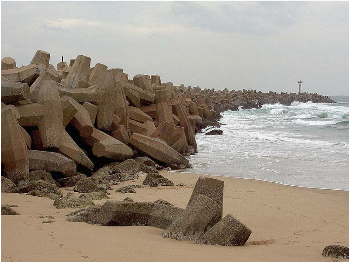
Durban's South Pier with a line of interlocking dolosse, South Africa
