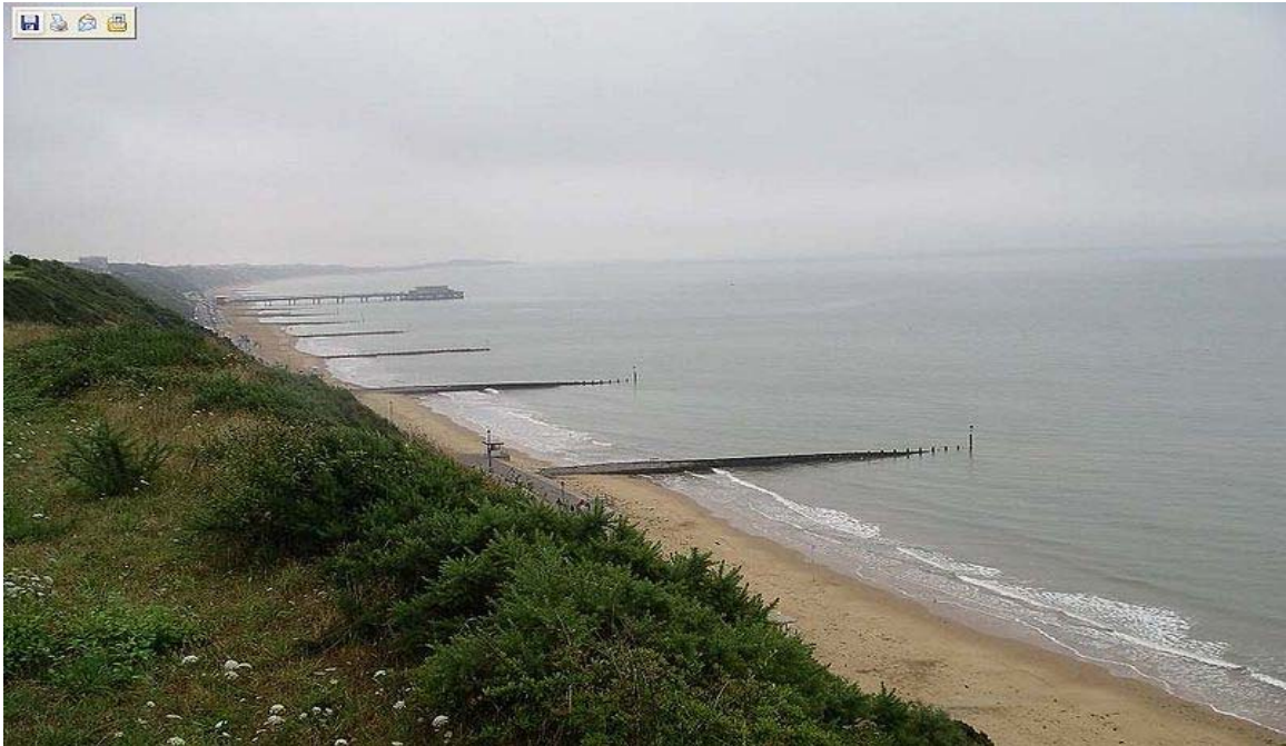
Timber groynes in Bournemouth, England
