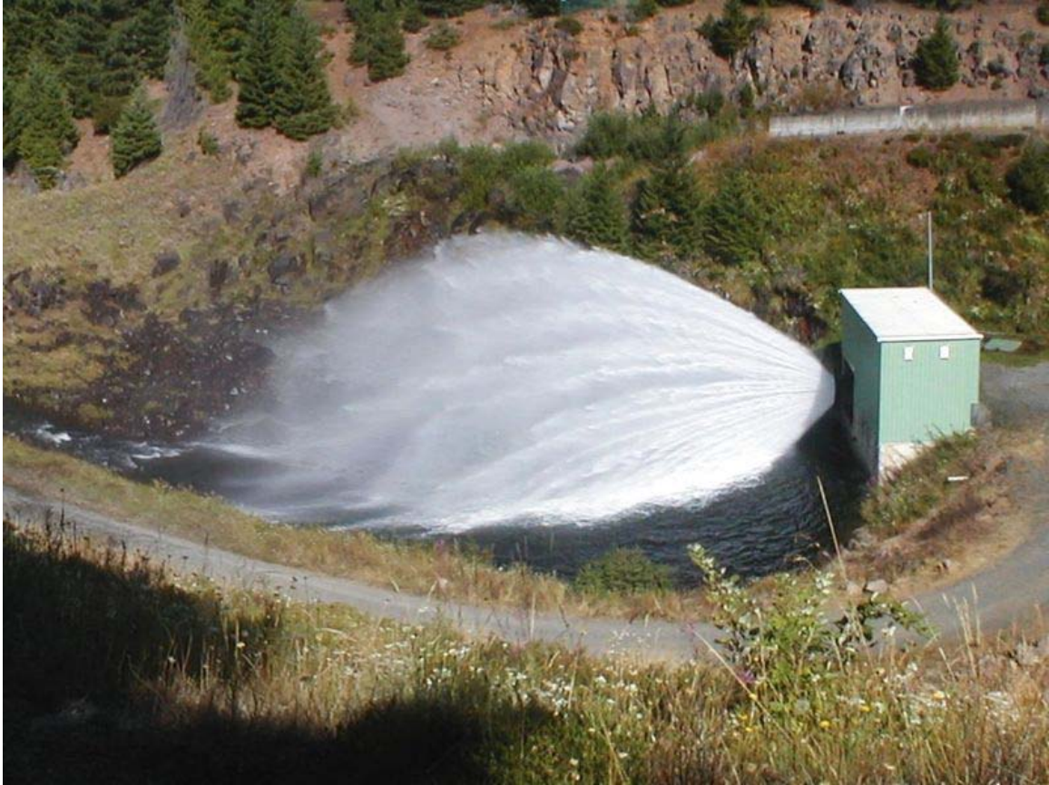
Discharge from a Howell-Bunger valve
