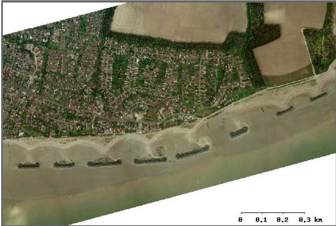
The eight offshore breakwaters at Elmer, UK
