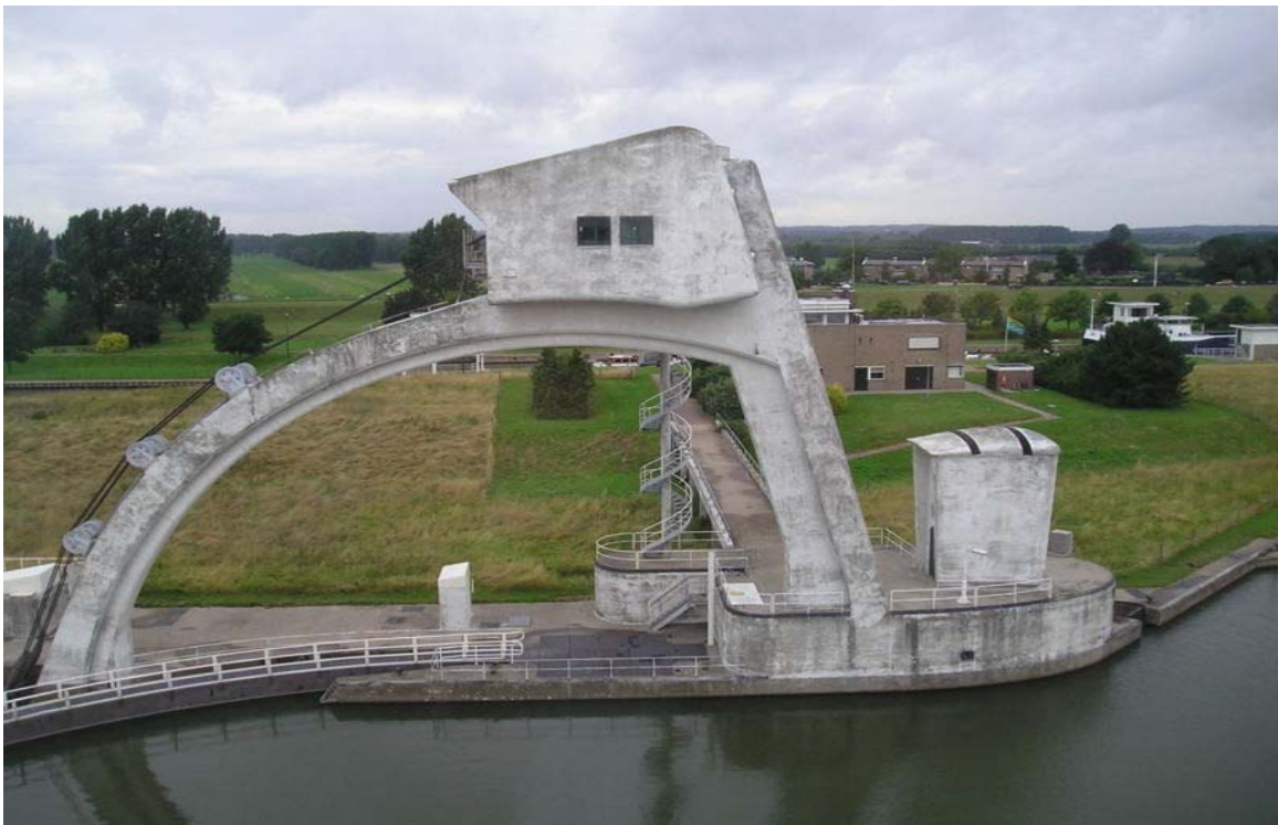
Floodgate Amerongen, The Netherlands
