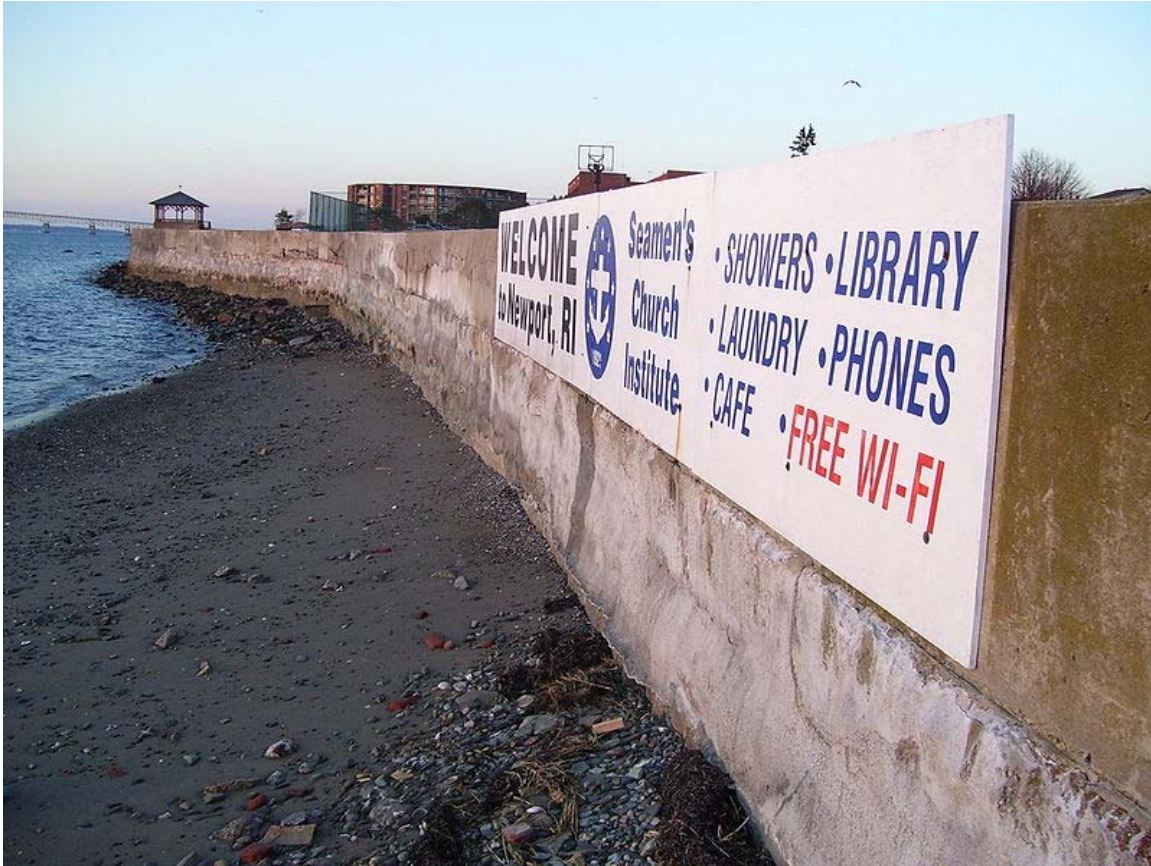
Seawall on Goat Island in Newport, Rhode Island, USA
