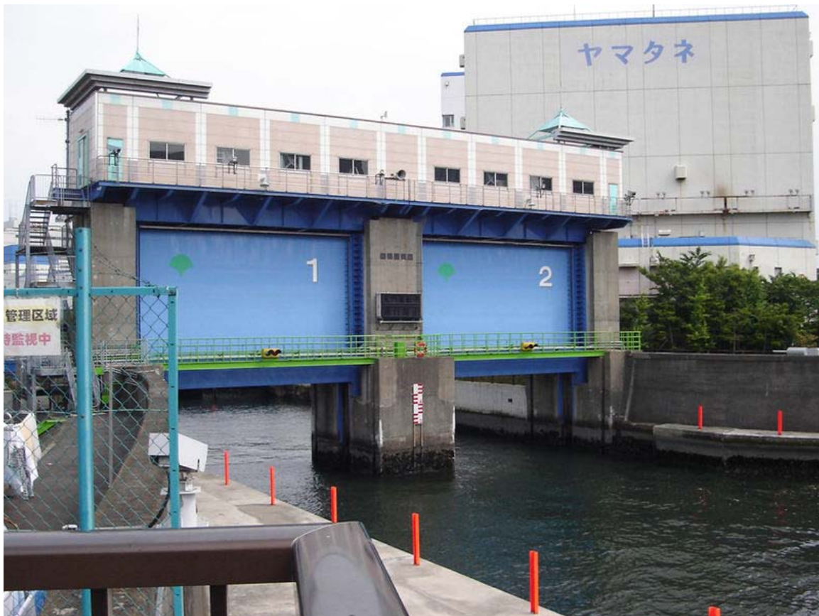
Tokyo floodgates created to protect from typhoon surges
