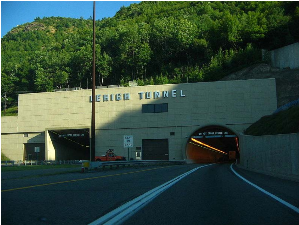
Lehigh Tunnel, Pennsylvania
