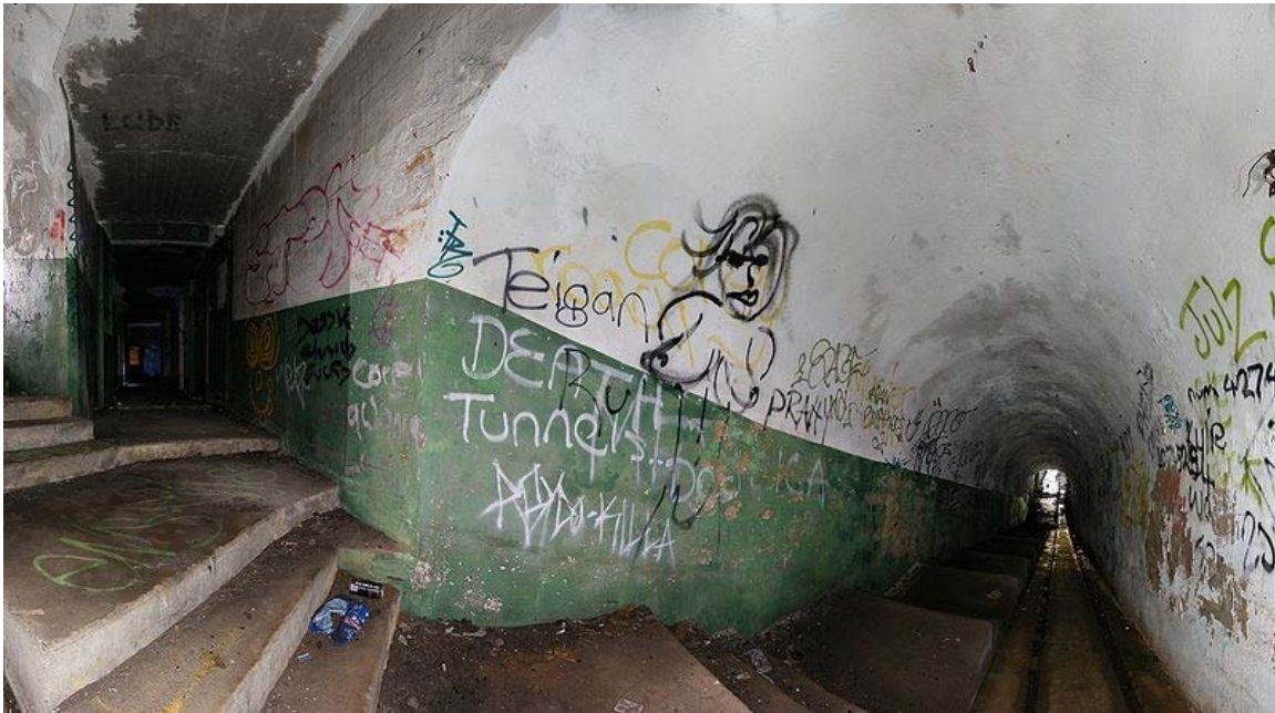
Illowra Battery utility tunnel, Port Kembla. One of many bunkers south of Sydney.
