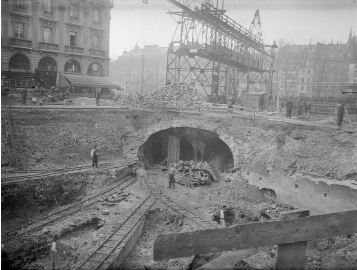
Cut-and-cover constructions of the Paris Métro in France
