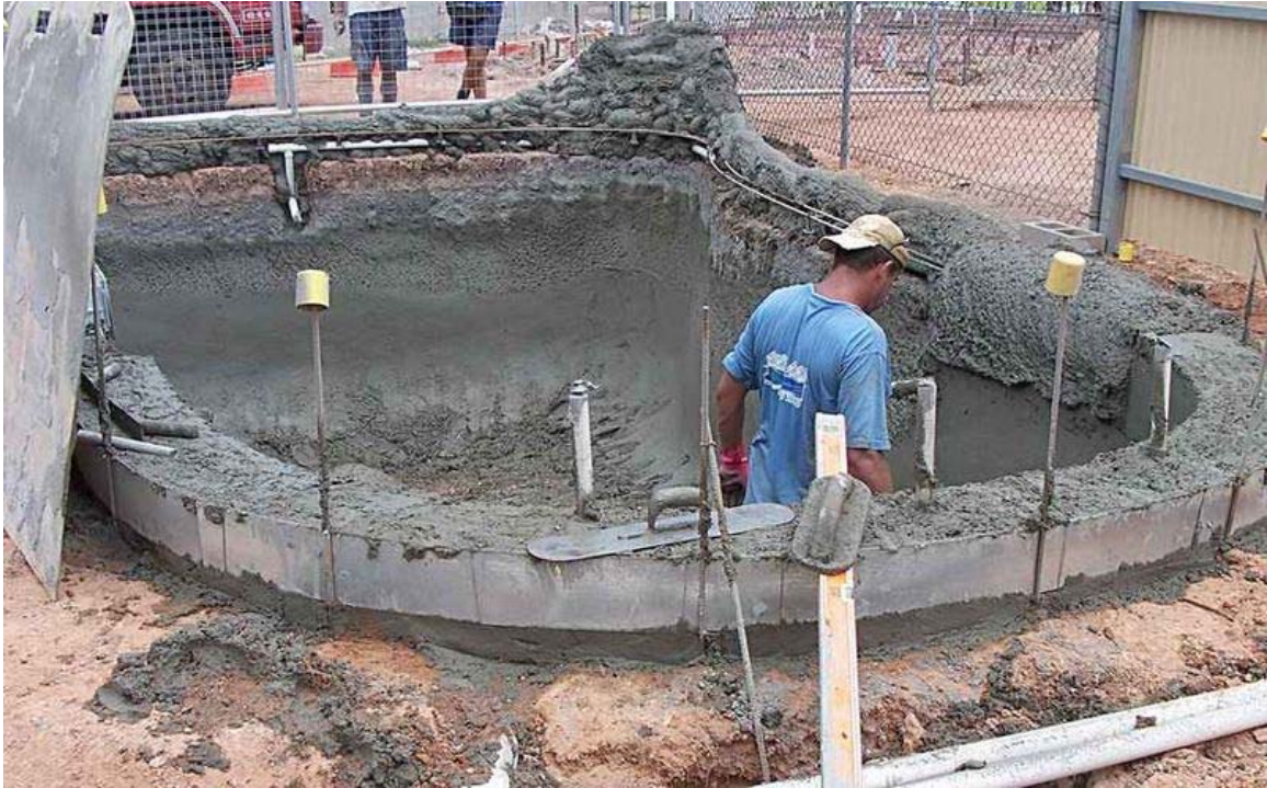
Shotcrete swimming pool under construction in Northern Australia.
