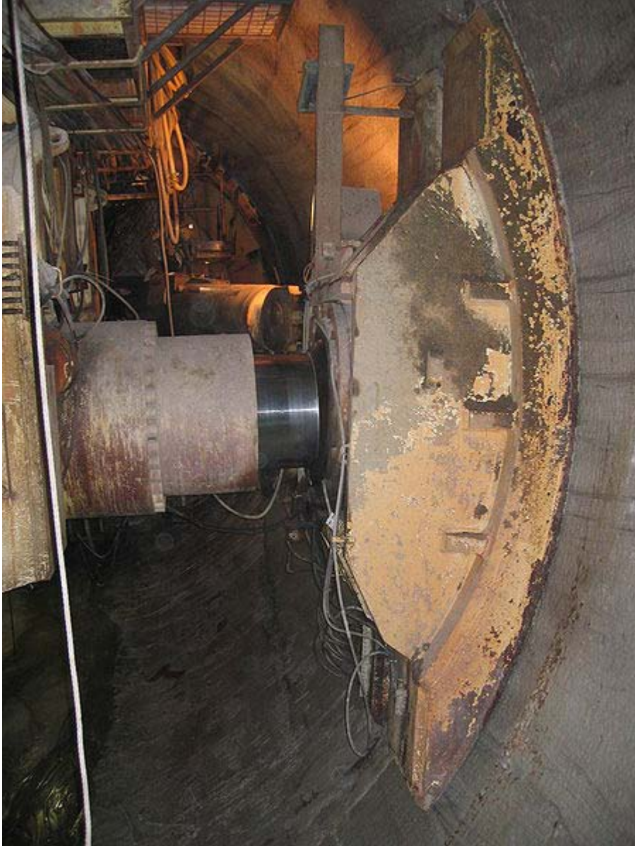
Hydraulic jacks holding a TBM in place.
