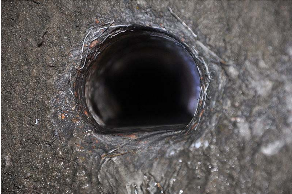
A 76 mm borehole in fibre reinforced shotcrete on a tunnel wall
