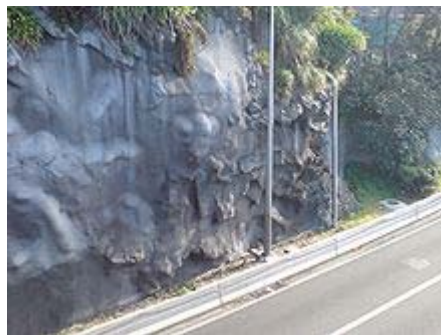
Shotcrete-stabilized cliff above a motorway in New Zealand
