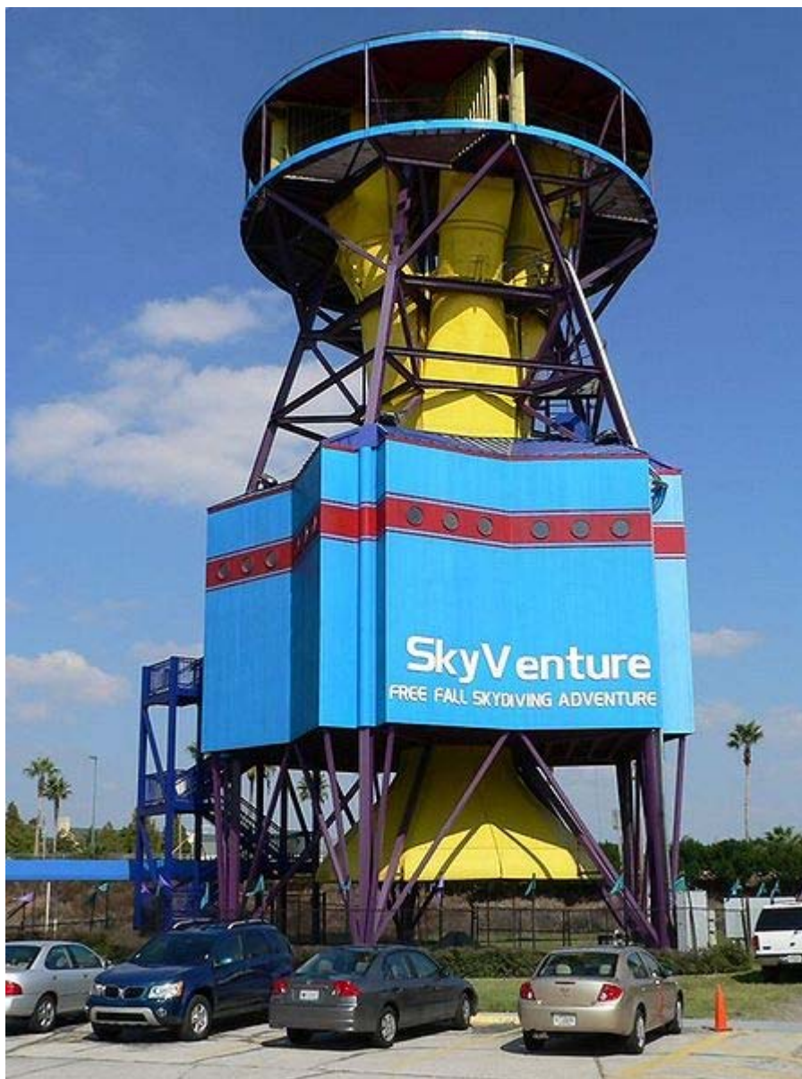
Non-recirculating indoor vertical wind tunnel.
