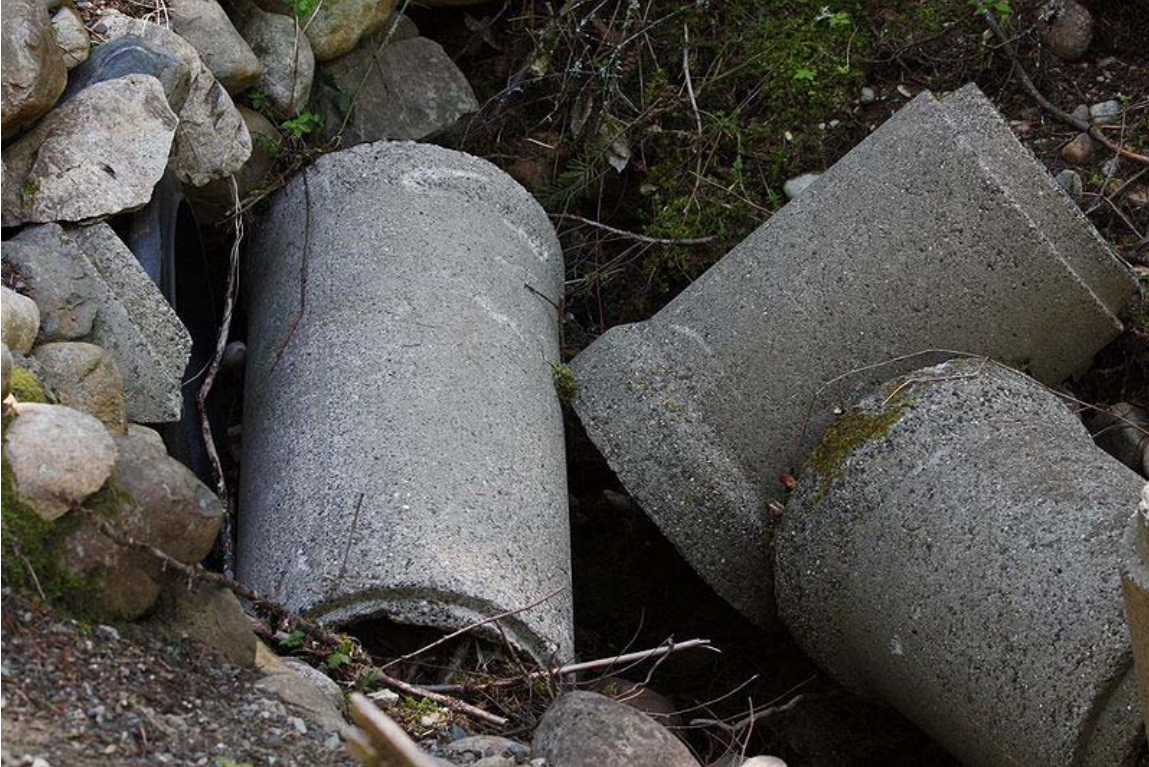
Precast concrete culvert segments
