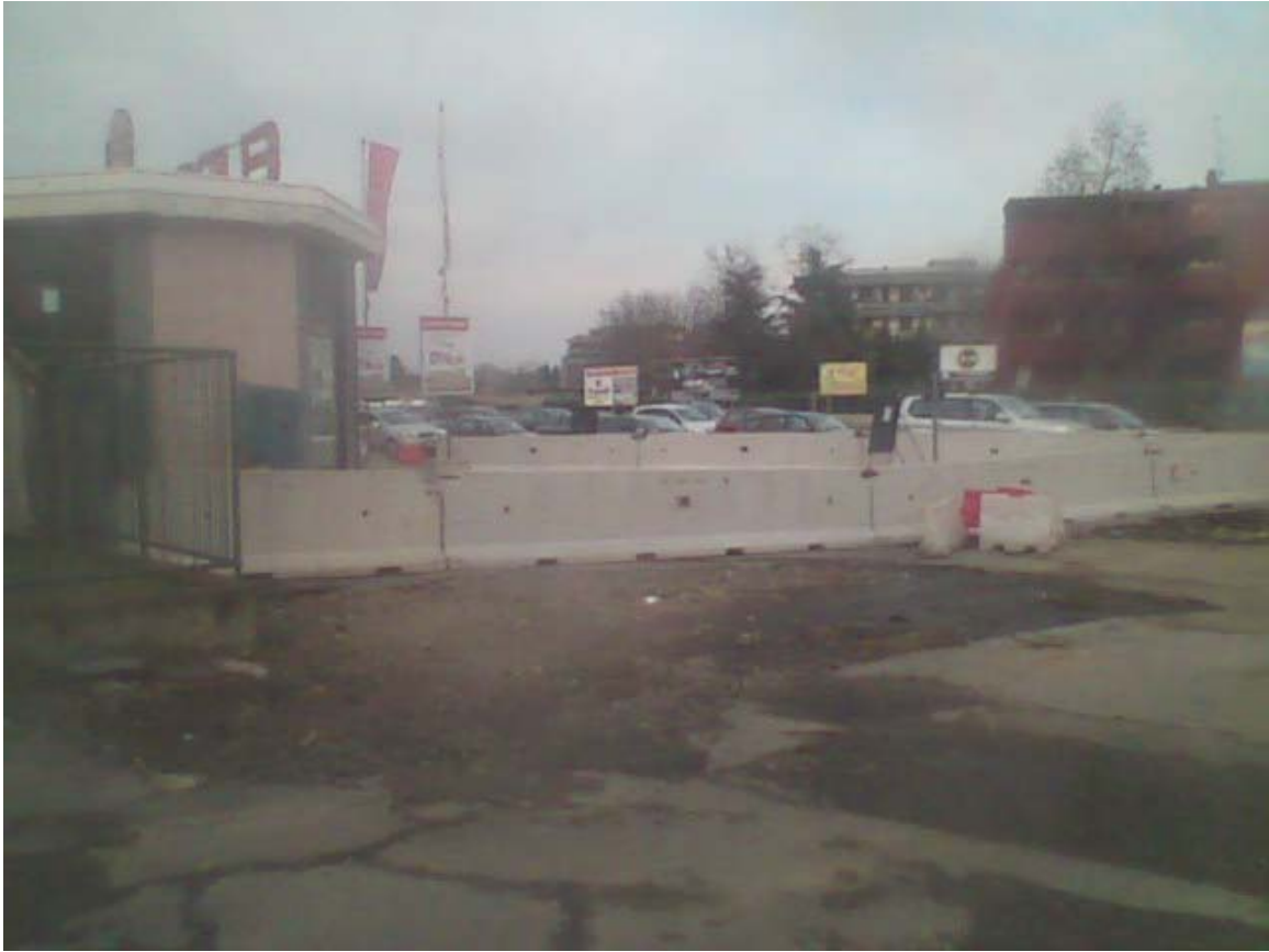
The construction of a Tunnel at Monza, Italy
