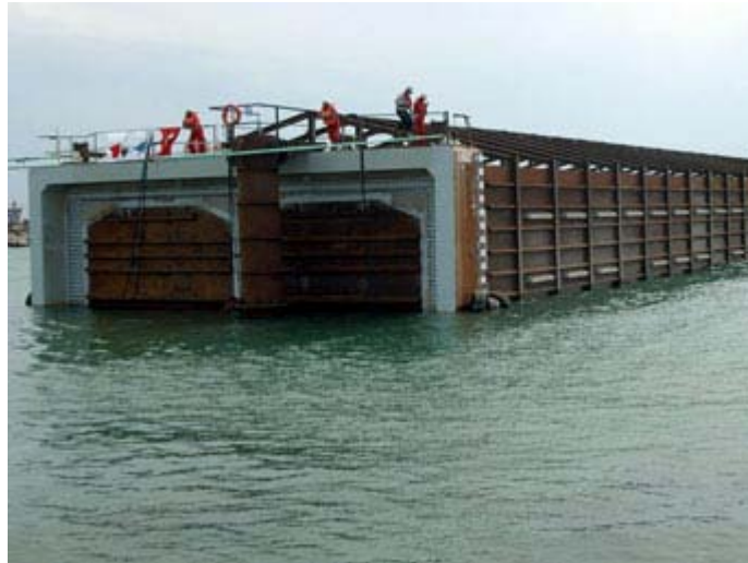
The Marmaray immersed tube in Istanbul, Turkey during construction.
