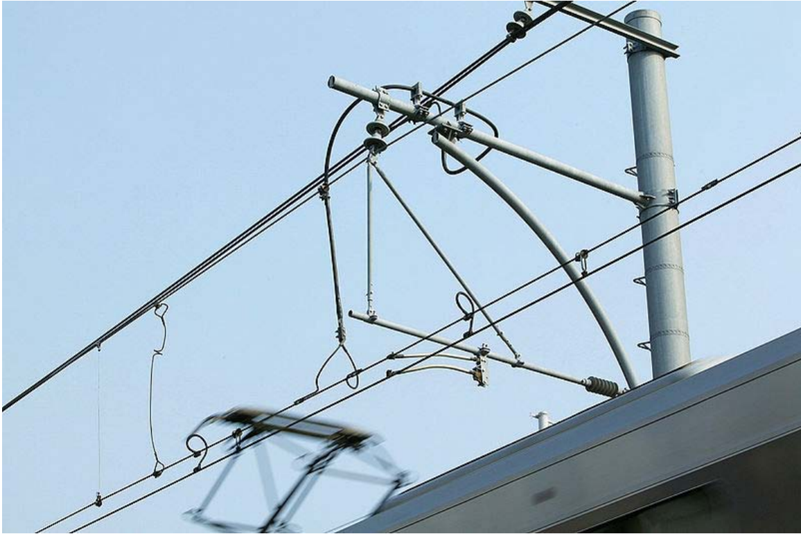
Compound catenary equipment of JR West
