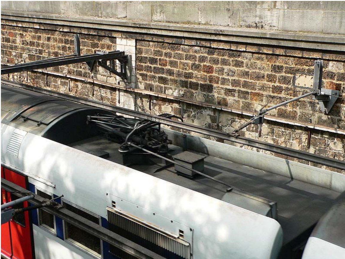
Overhead feeding rail on the RER Line C trenches and tunnels in central Paris
