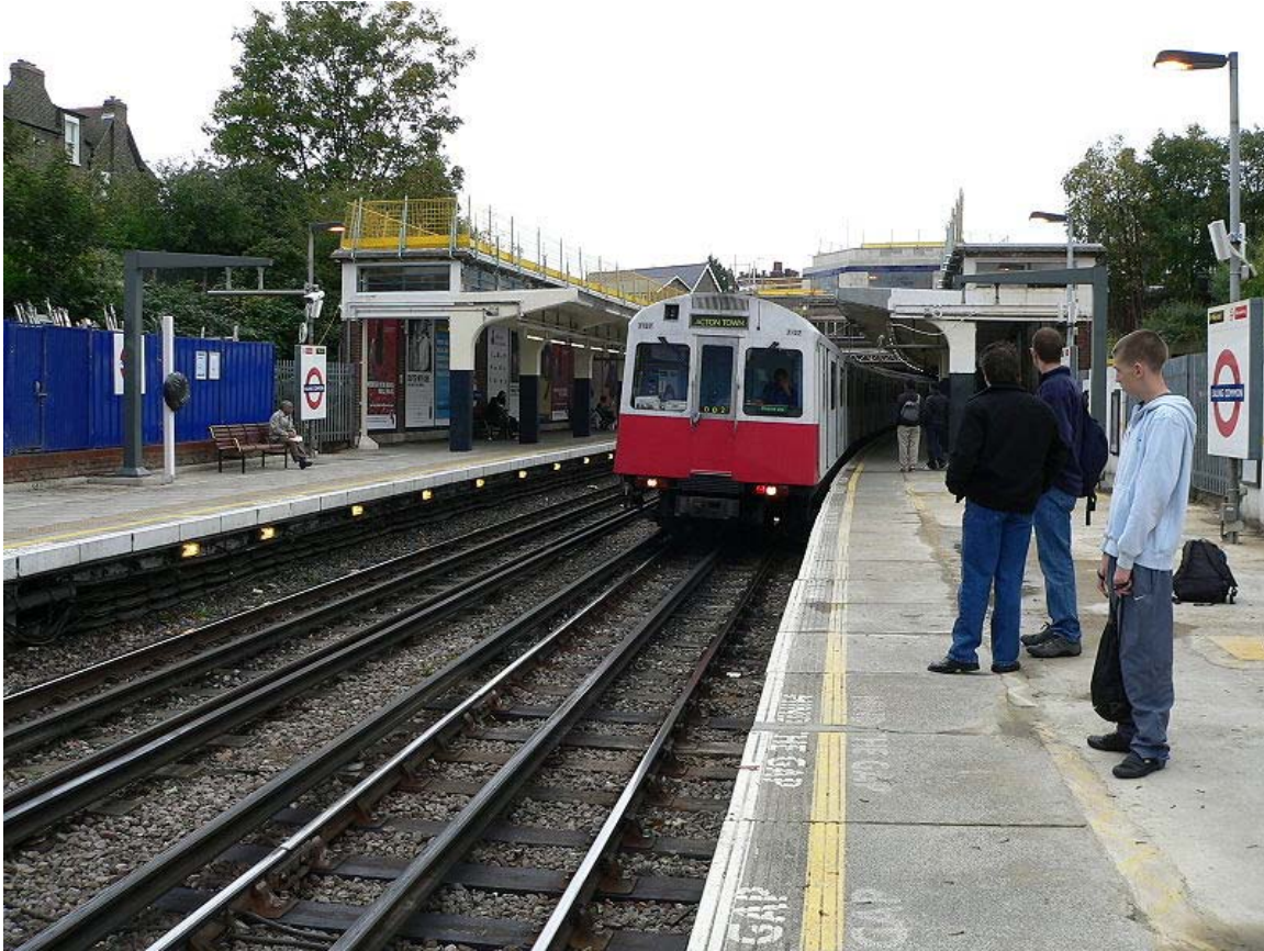
London Underground track at Ealing Common on the District Line, showing the third and fourth rails beside and between the running rails
