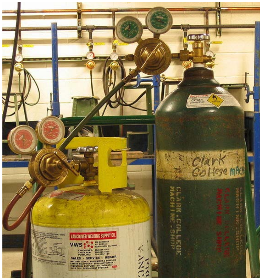
Oxygen and MAPP gas cylinders with two-stage pressure regulators
