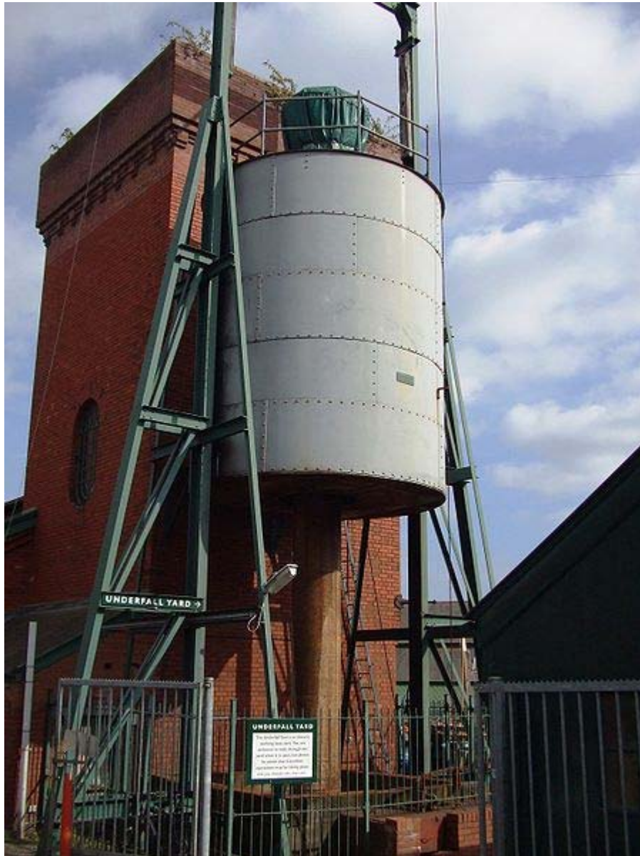
Hydraulic engine house, Bristol Harbour
