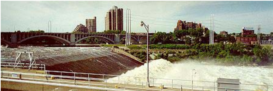
Saint Anthony Falls on the Mississippi River showing a pronounced hydraulic jump.
