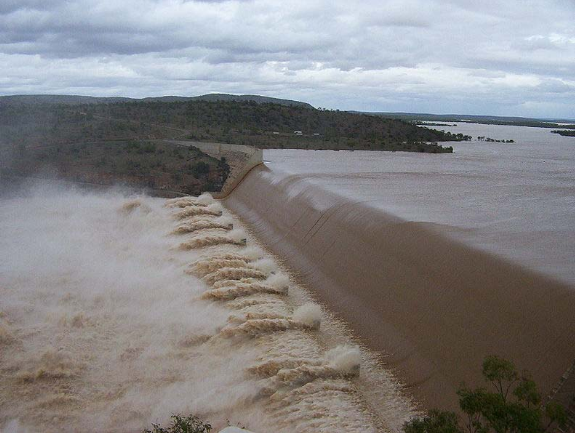
Burdekin Dam on the Burdekin River in Queensland, Australia showing pronounced hydraulic jump induced by down-stream obstructions and a grade change.
