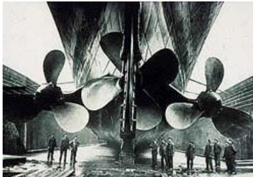
Propellers of the *Titanic*: 2 triple-blade and 1 quadruple-blade at center
