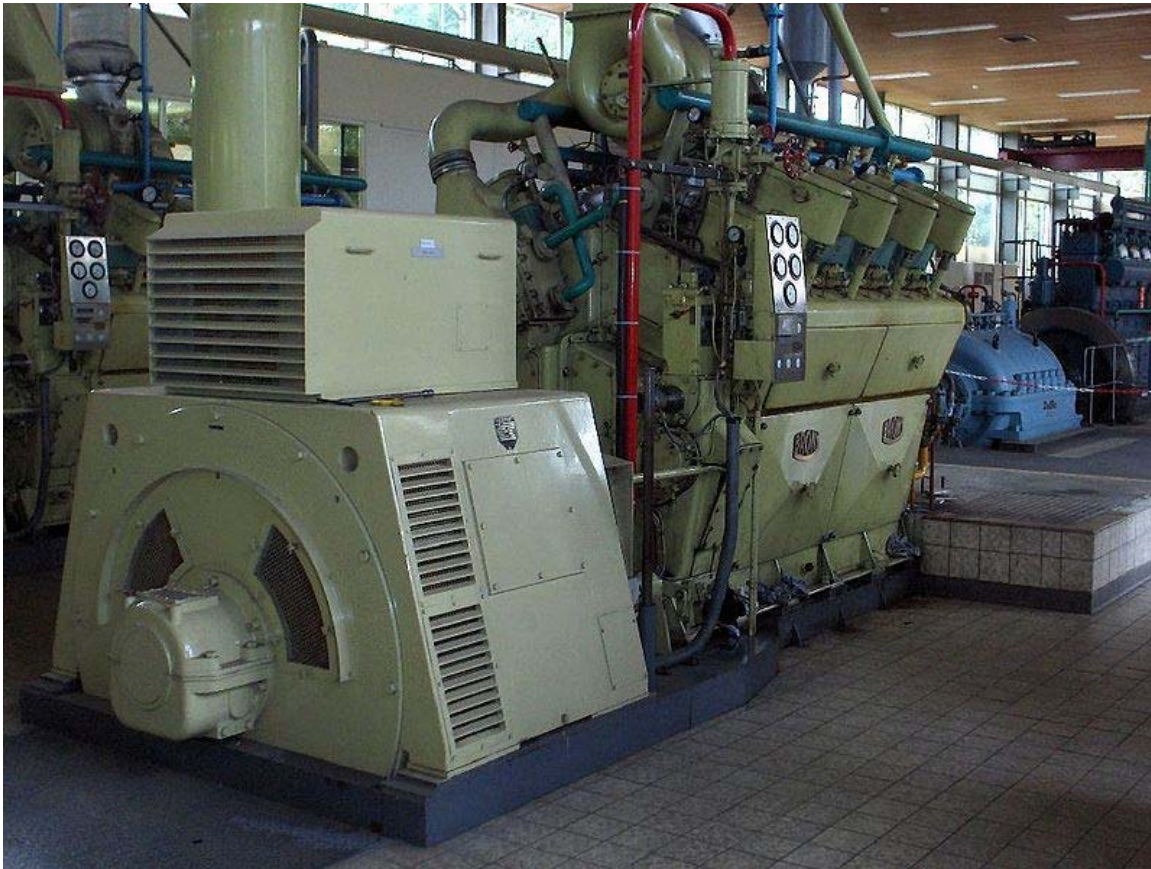
Brons two-stroke V8 Diesel engine driving a Heemaf generator.
