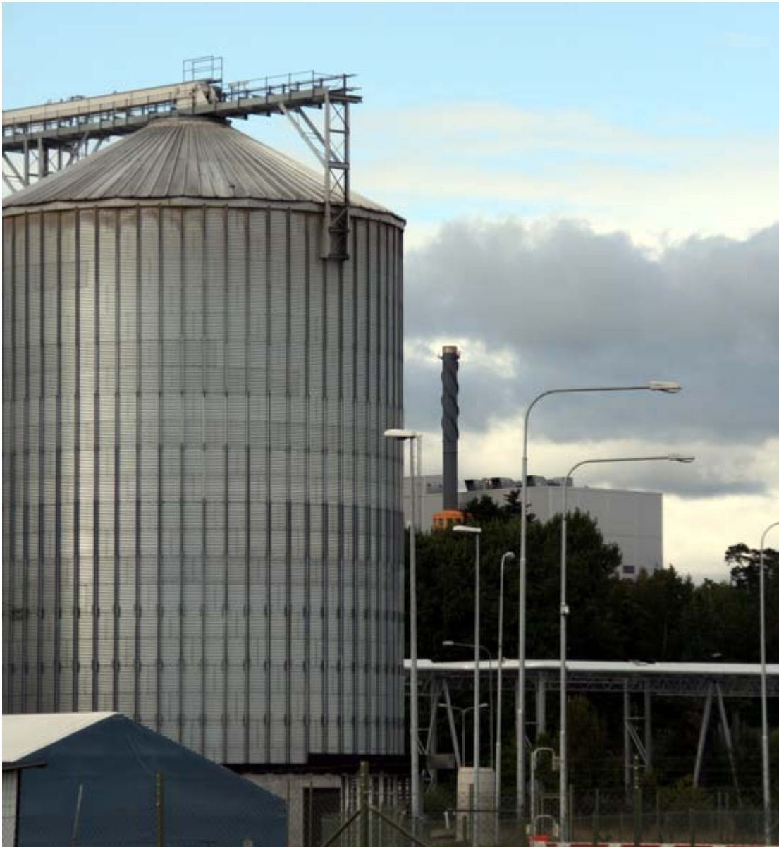
Example of Industrial Symbiosis. Waste steam from a waste incinerator (right) is piped to an ethanol plant (left) where it is used as input to their production process.
