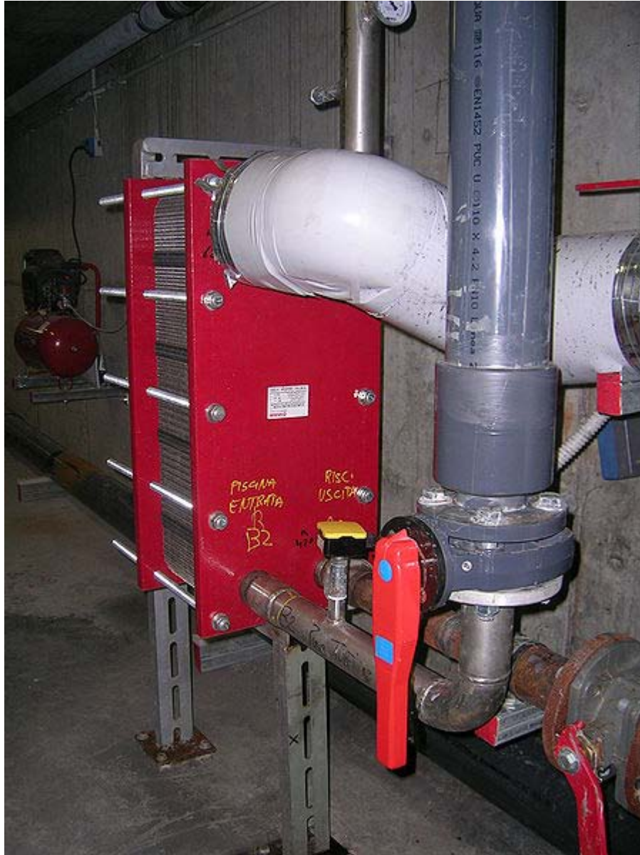
An interchangeable plate heat exchanger applied to the system of a swimming pool
