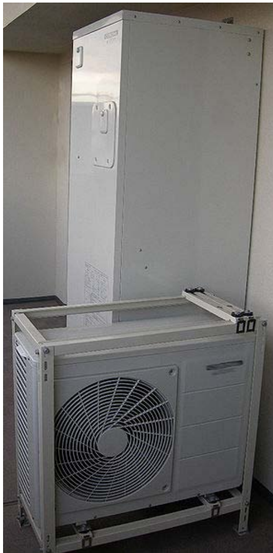
Domestic EcoCute outdoor unit (front) and hot water storage tank (back)
