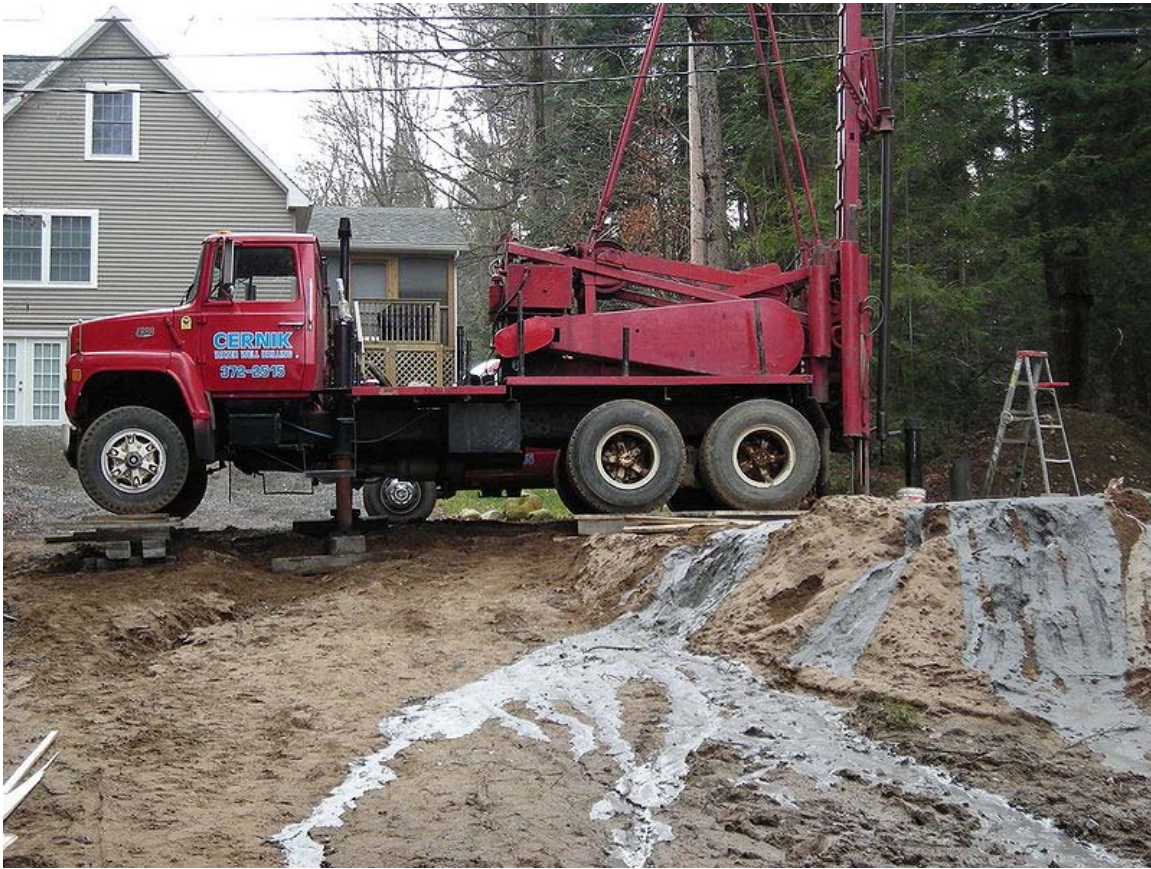
Typical drill rig for water source installation, length 22 ft
