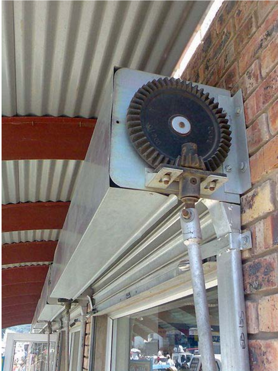
Bevel gear on roller shutter door.
