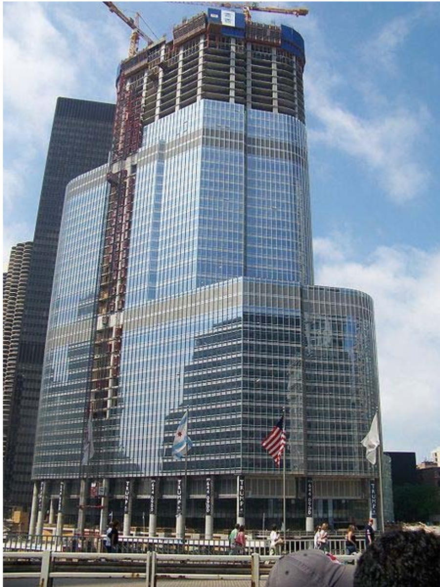
A hoist on the Trump International Hotel & Tower-Chicago
