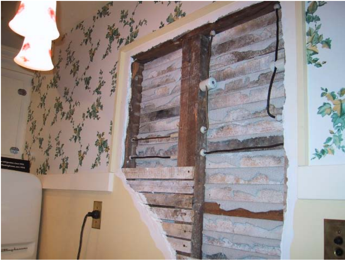
Knob and tube wiring at a museum display
