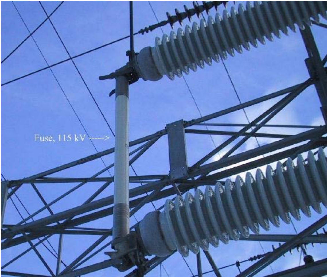
A 115 kV high-voltage fuse in a substation near a hydroelectric power plant.
