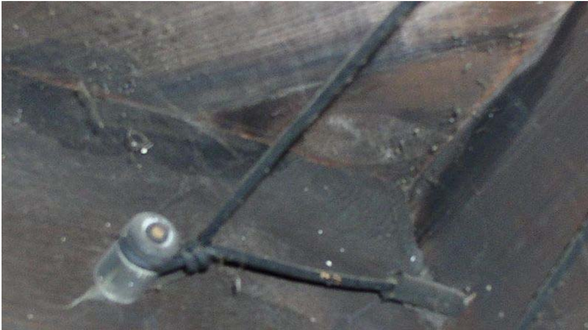
Knob supporting a wire change in direction.
