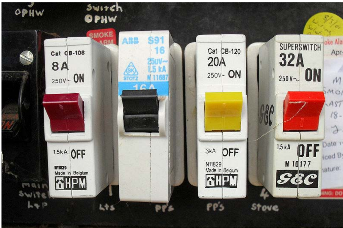
Four 1 pole circuit breakers
