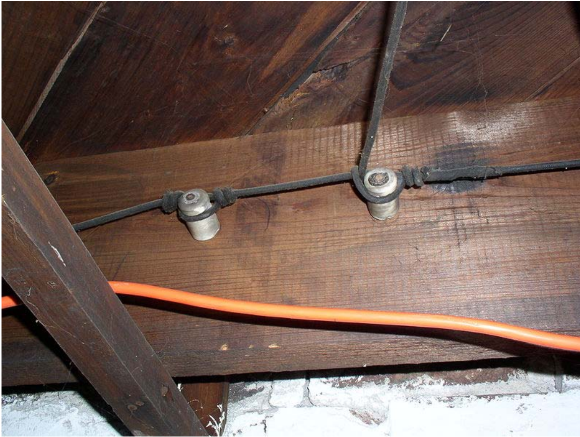
Knob-and-Tube wiring
