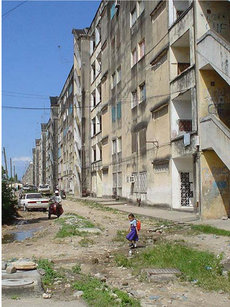
Urban decay in Zanzibar, Tanzania.
